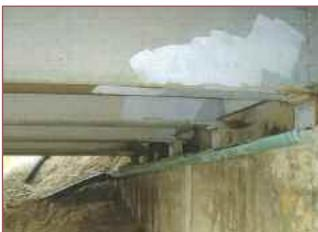
Drainage trough to contain leaking seal – existing bridge
