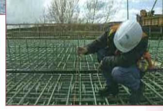
Checking cover to reinforcing steel
