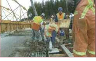
Placing South abutment deck thickening
