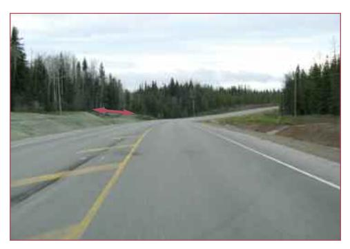
Reapplication of revegetative seeding and west end back slope failure still requiring repair
