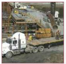
Moving rock socket reinforcing cage.
