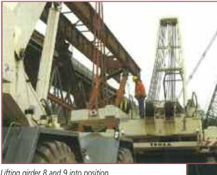
Lifting girder 8 and 9 into position. Mobilizing two 300-Tonne cranes from heavy-lift locations at Pier 3 to Pier 2
