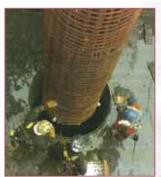
Lowering rock socket cage into pile.
