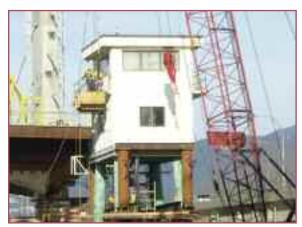
February 2009 Lowering of Control Tower to make room for deck span
