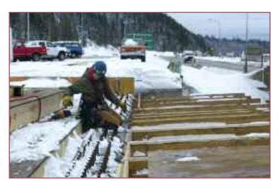
Installing final overhang panels
