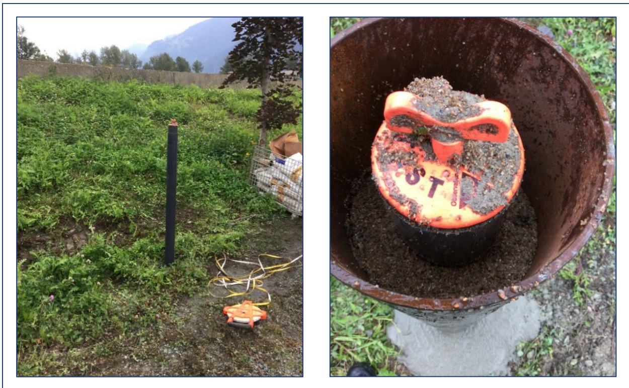
Figure 5-6 Examples of PVC riser pipe before (left) and after (right) the protective surface casing is installed.
