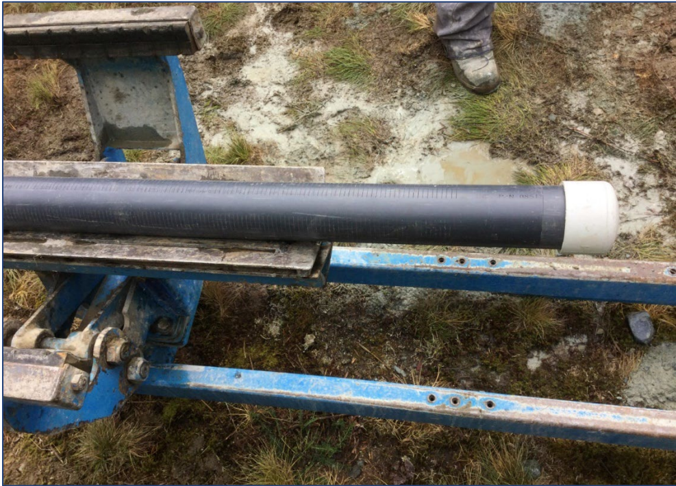
Figure 5-5 Provincial Observation Well screen with endcap prior to installation.
