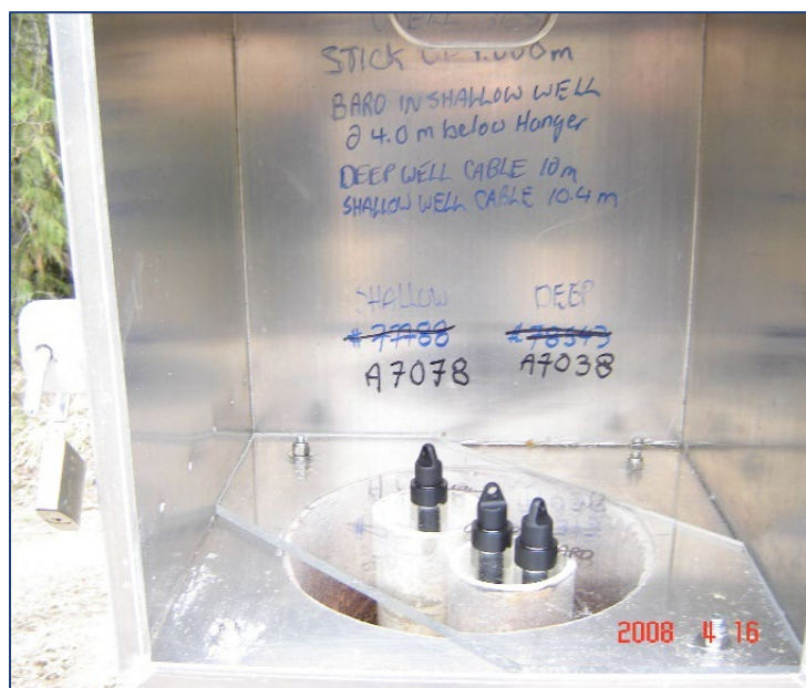
Figure A2-5.1 Suggested direct-read cable set-up to avoid changes in cable length.
