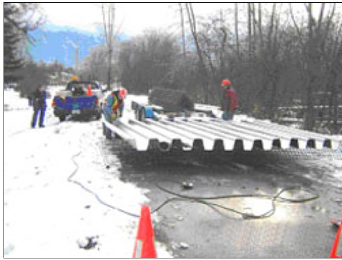
THE FORMED SHEET STEEL STRINGER IS ASSEMBLED
