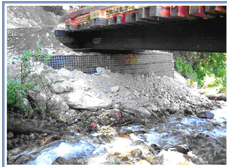
Figure 6 A Reinforced Soil Bridge Abutment
