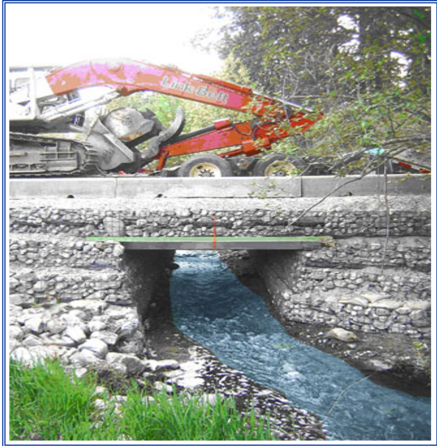
Figure 8 A Reinforced Soil Box Culvert or Small Bridge Structure
