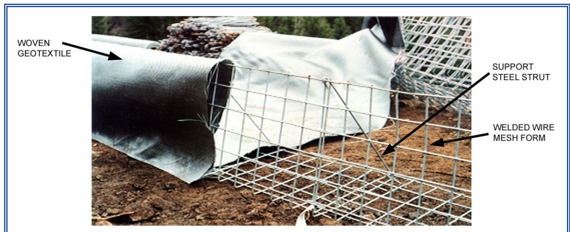
Figure 2 Wire Mesh, Struts and Woven Geotextile Materials
