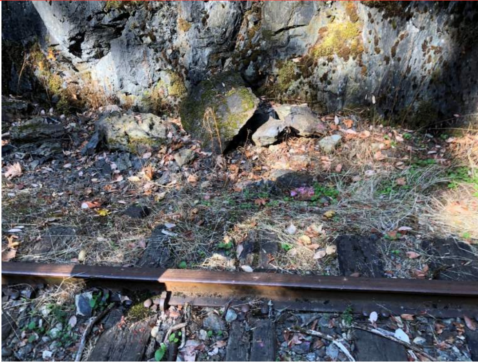
Photo 13: Fallen rock at tunnel entrance South.
