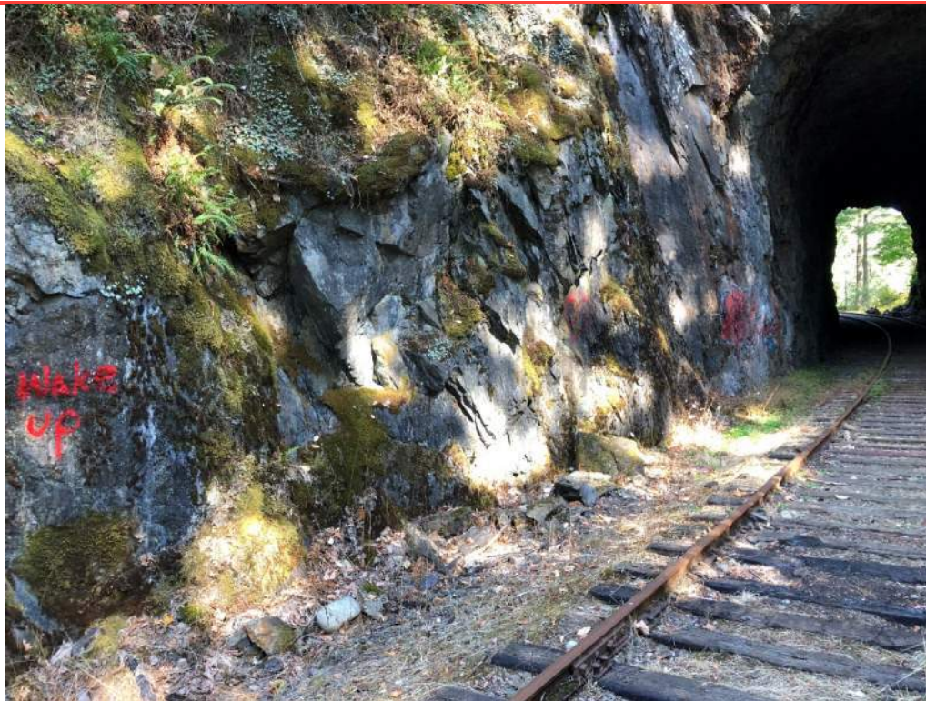
Photo 12: Fallen rock adjacent to Tunnel entrance South.
