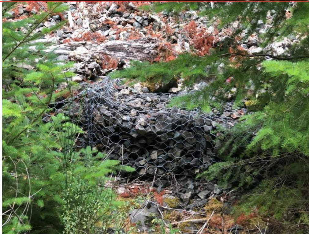
Photo 4: Gabion baskets at toe of slope approx. co-ord. 49.293110 - 124.589763.
