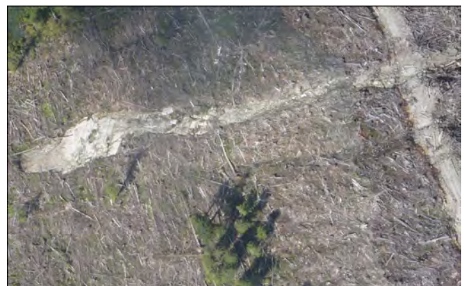
Close-up of Pic_52 showing slope failure.
