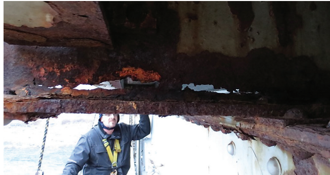
Corrosion Section Loss (approx. 500mmx20mm) in Web at Floorbeam
