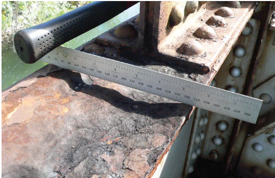
Corrosion Section Loss at Top Flange at Bearing Beam
