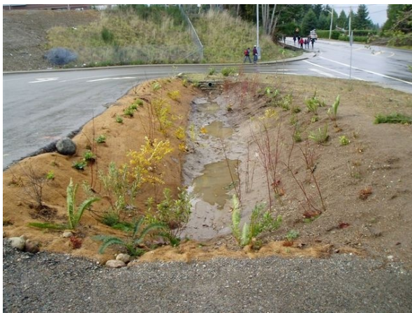
Raingarden built to manage stormwater—at construction. PHOTO: FAYE SMITH
