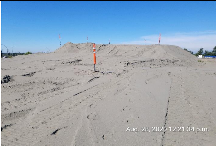
Photo 1. Most working surfaces are covered with sand preload such as the L575 (28 Aug 20)
