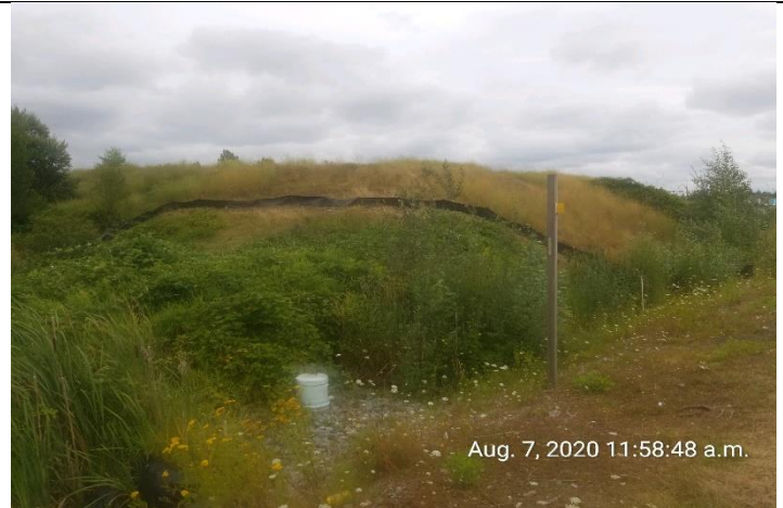
Photo 2. Location: Looking northeast from SFPR towards the L100. Description: Sediment fencing had been erected serving dual purpose as ESC measures and wildlife isolation (07 Aug 2020).
