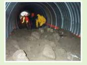
A conveyor system provides a means for infill material to be delivered into the culvert.
