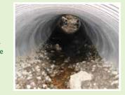
Infill material can be pulsed through or within the culvert during high flow events. Having the proper matrix of material sizes to mimic the natural stream substrate helps to keep this material in place and prevent the culvert bottom from being exposed.
