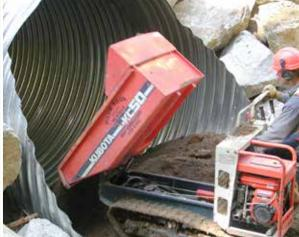
Manual infill methods include buckets and wheelbarrows. Careful attention needs to be given to the staging area to address safety near the edge of the culvert.
