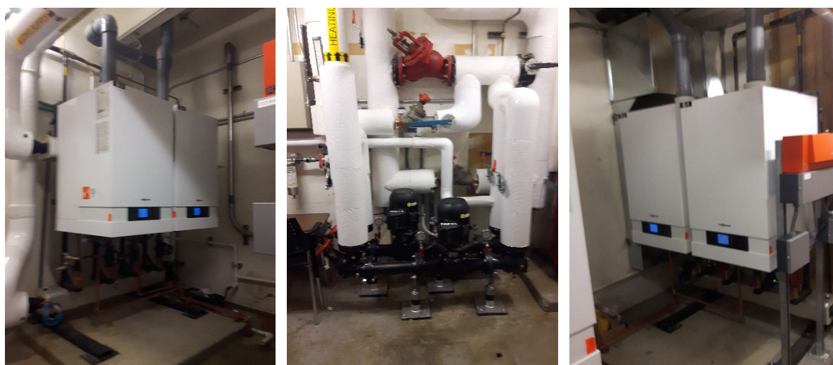
Figure 7 – Ecole Puntledge Park Boiler Plant Upgrade Project: four new high efficiency Viessmann condensing boilers and pumps.
