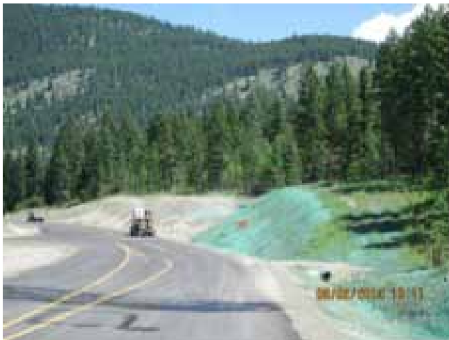
Paved and Hydroseeding 300L
