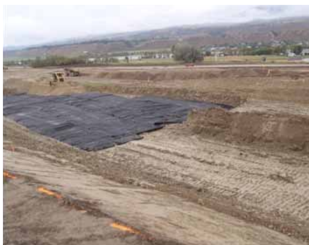
Non-woven Geotextile Placement East Bound Off Ramp
