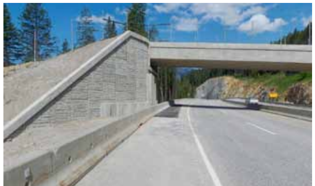
MSE Wall Repair Complete – Glenogle 19 June 2014
