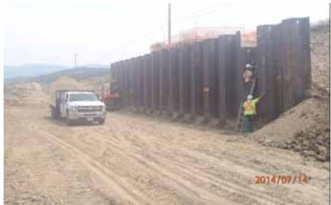
Bostock Sheet Pile Wall
