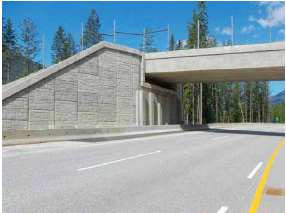
MSE Wall Repair Complete – Glenogle 19 June 2014
