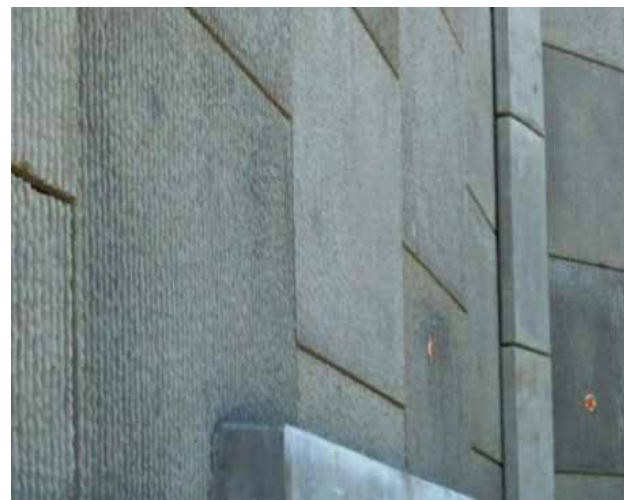
MSE Wall A repairs now completed and backfilled; April 22, 2013
