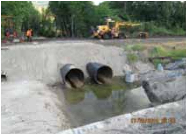
After Augering piper under CP Rail
