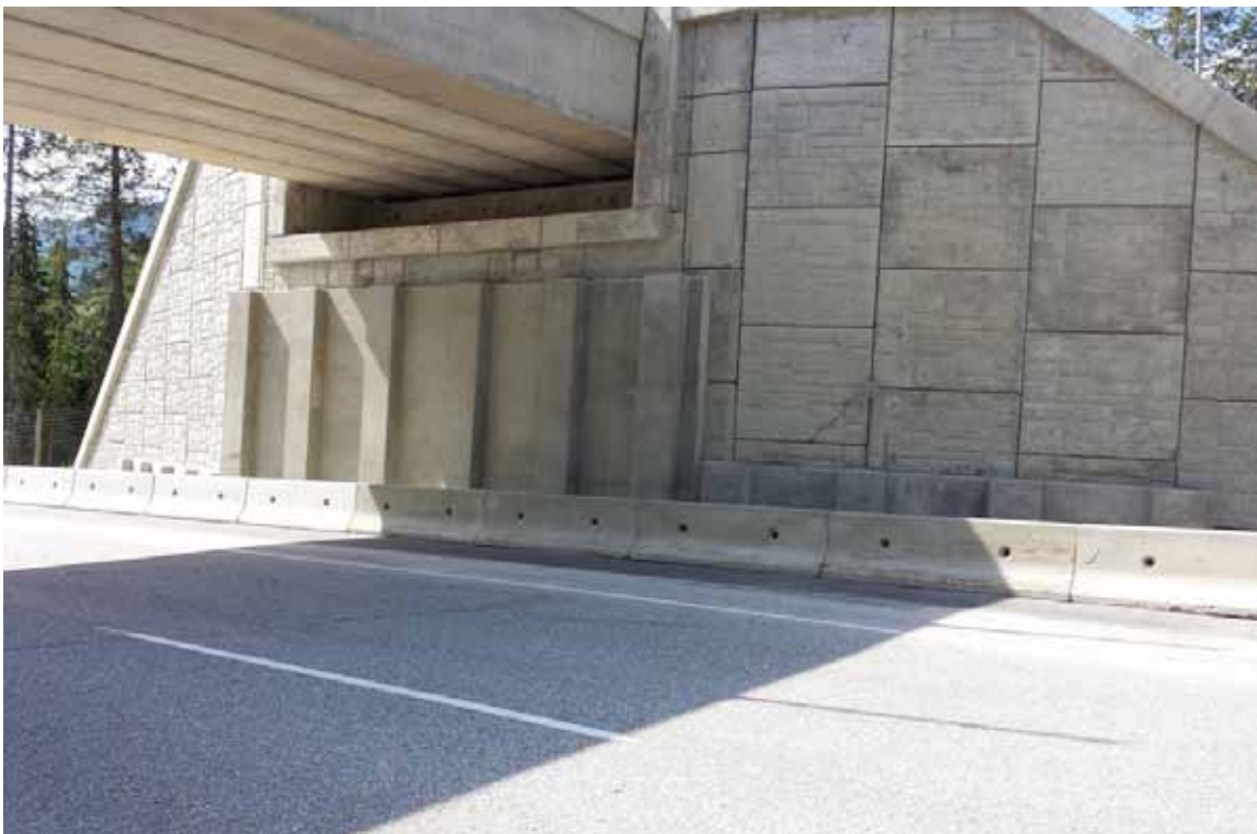
MSE Wall Repair Complete 2014
