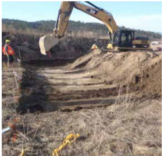
Controlled Excavation
