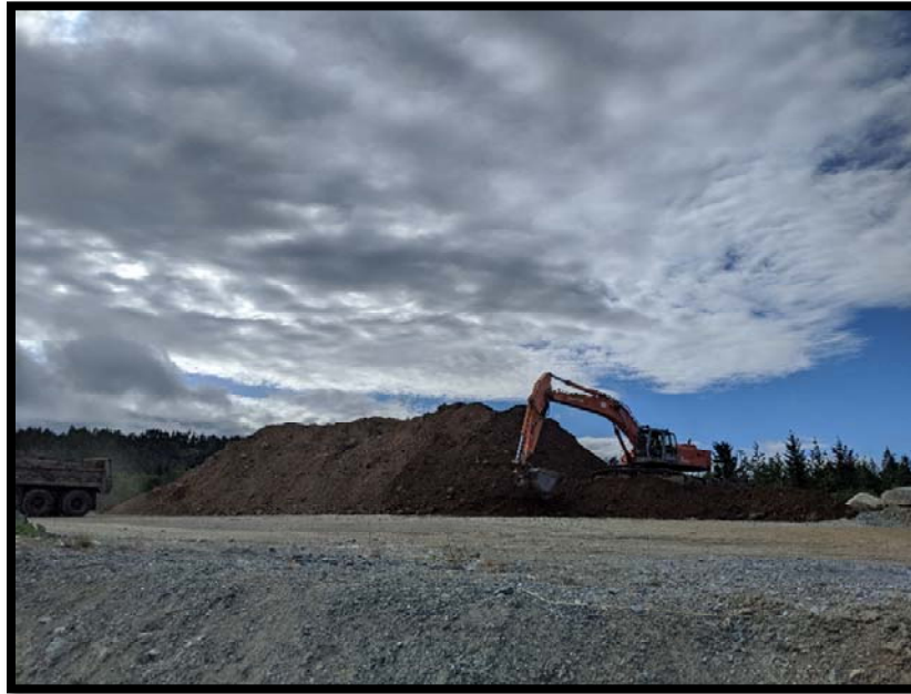
Picture # 3: Looking south from the south side of the PEA towards an excavator stockpiling imported capping material at the southeast corner of the site. Capping material was imported and stockpiled throughout the day.
