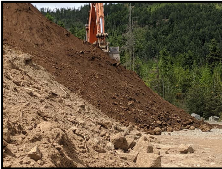
Picture # 4: View of the imported soil capping material. Some larger rocks and roots are present in the capping material. Contractor informed Islander (Joel Clarkston) that they will be removed prior to final placement.
