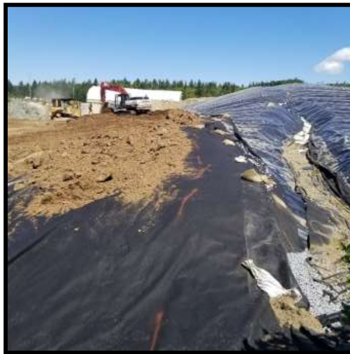
Picture # 4: Soil Placement on the North Face
