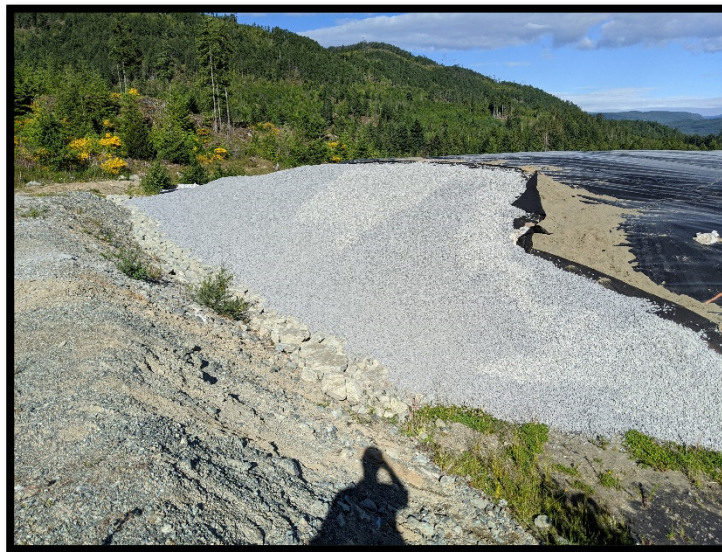
Picture # 4: Drain rock placed on south face of PEA.
