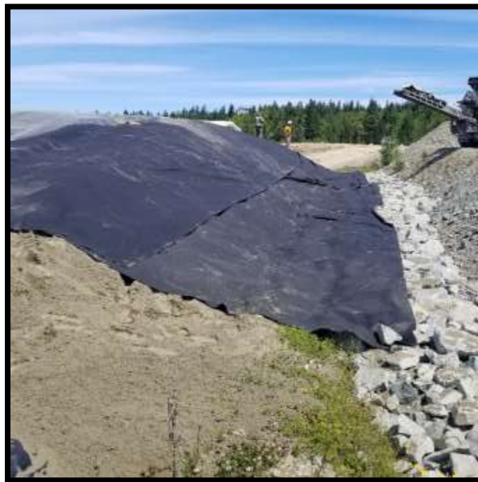
Picture # 2: South Face – Sand and Filter Cloth Placement
