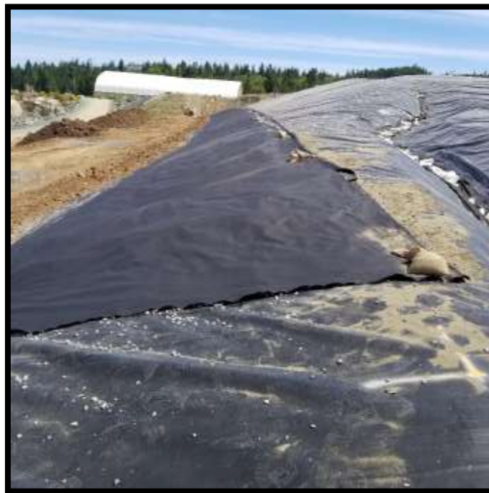
Picture # 4: North Face – Preparation for soil placement
