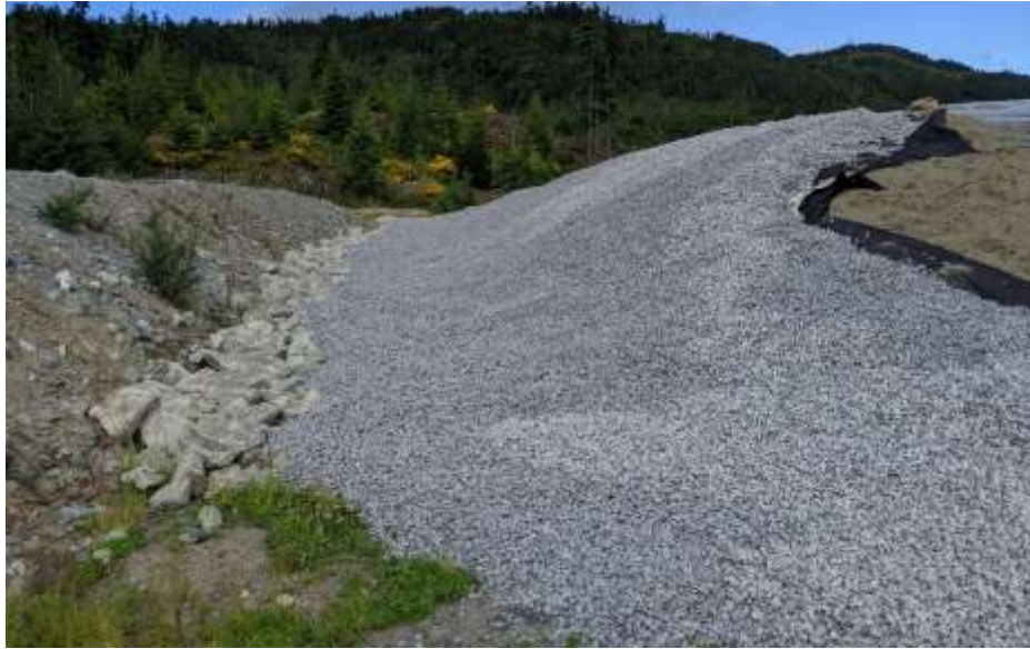
Picture #2: Drain rock on south slope of PEA
