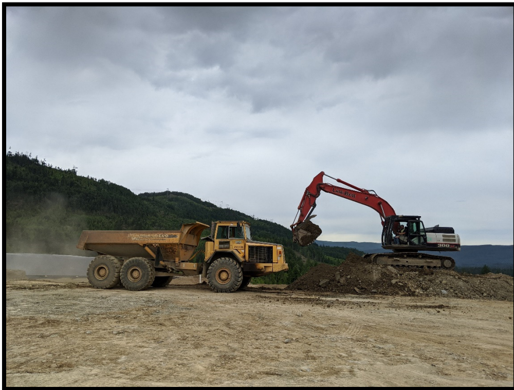
Picture # 4: Loading previously stockpiled soils from east of the PEA.
