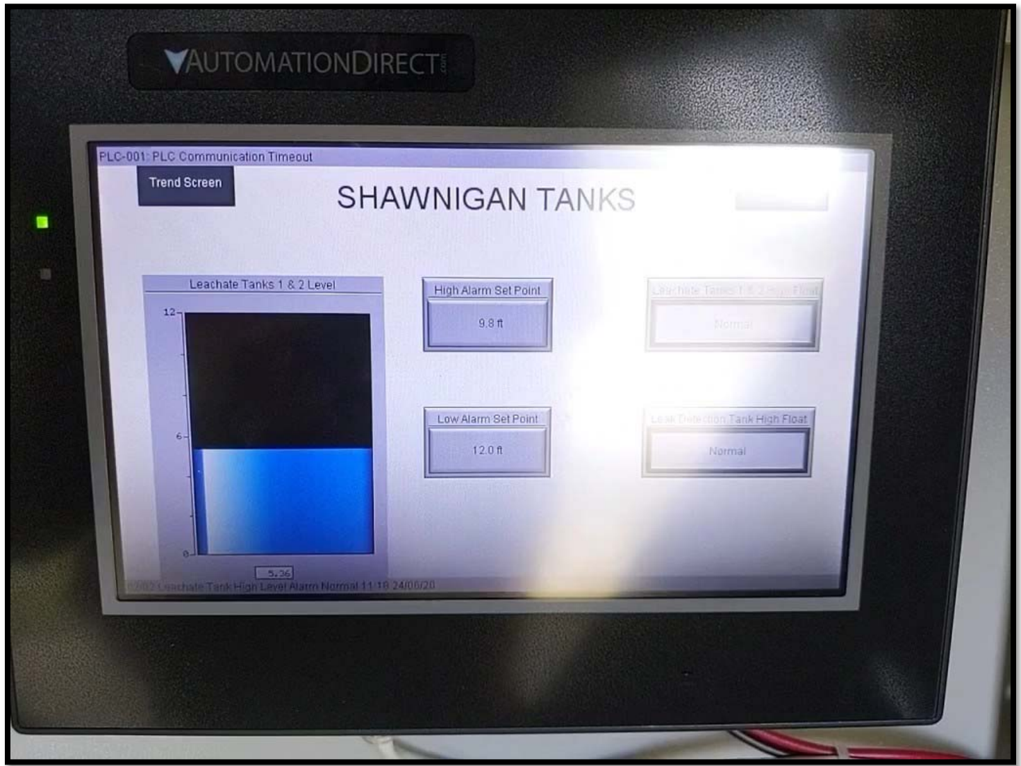
Picture # 5: Leachate display – 5.36 ft per tank.
