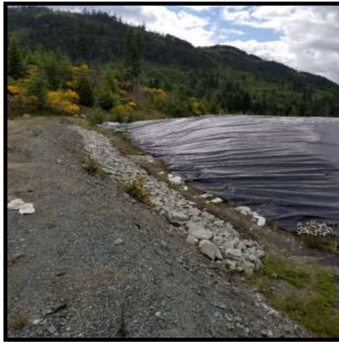
Picture # 1: Blast rock placed in East-West drainage ditch
