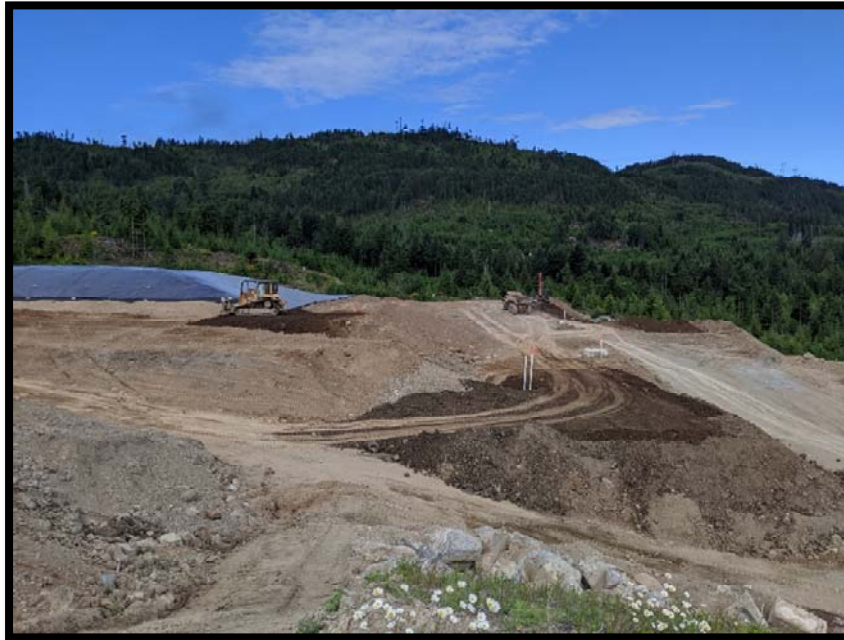
Picture # 1: Overview of construction progress, looking west. Previously stockpiled material on the north side of the PEA (excavator to right of the image) was hauled over to the east side of the PEA (bulldozer to the left of the image).
