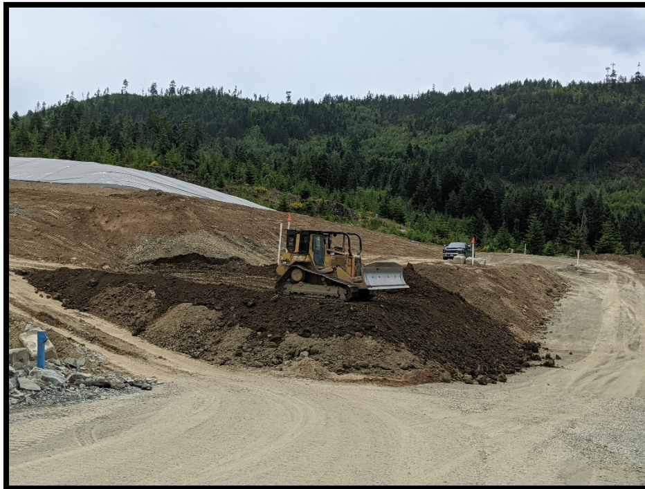
Picture # 2: D6 dozer track packing and distributing previously stockpiled soils.
