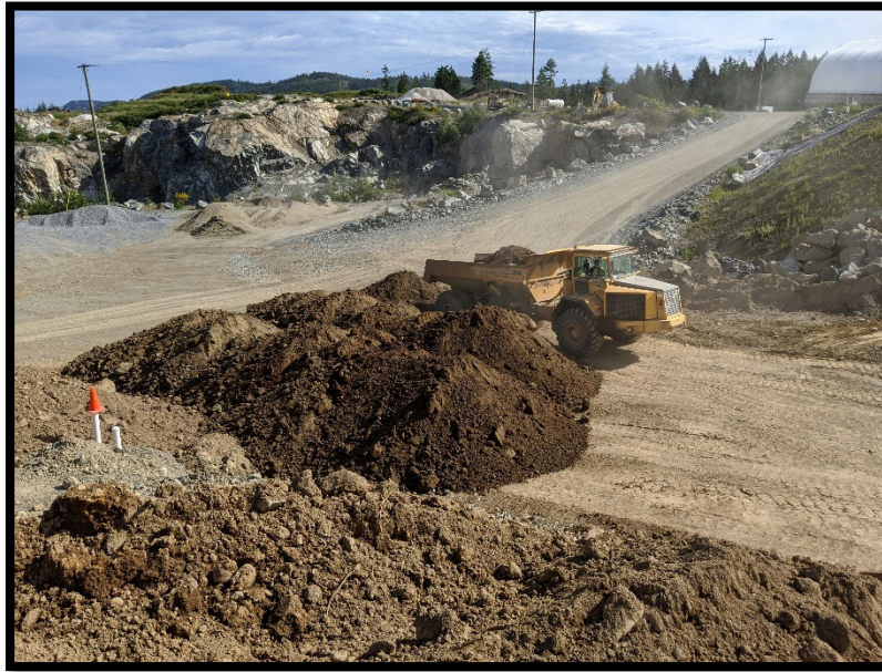
Picture # 5: Dumping of previously stockpiled soils at north east corner of PEA.
