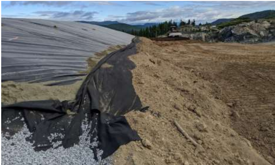
Picture #3: Soil stabilizing wedge at east side of PEA
