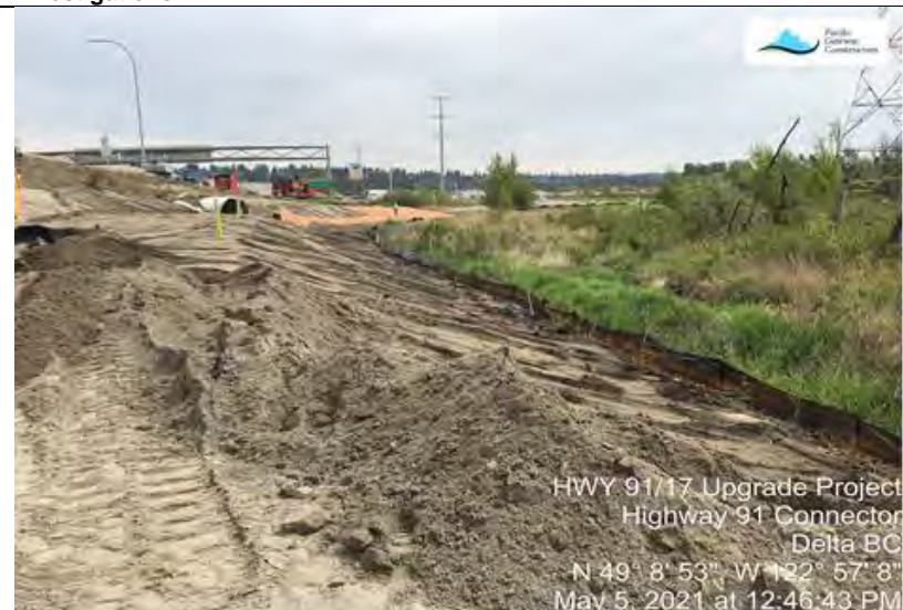
Photo 8. L550 (E), mitigation of steep slope and removal of sand migration in close proximity to the broject boundary. No sand was found in the stream and no instream works were done. ESC fences were inspected and found to be fully functional and keyed in.
