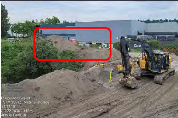
Photo 1: Excavated sand placed outside the project limits.
