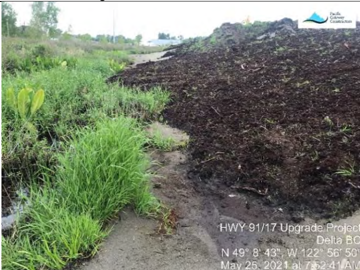
Photo 11. L1170, (F), peat placement on the sides of the embankment fill for bank stabilization.
