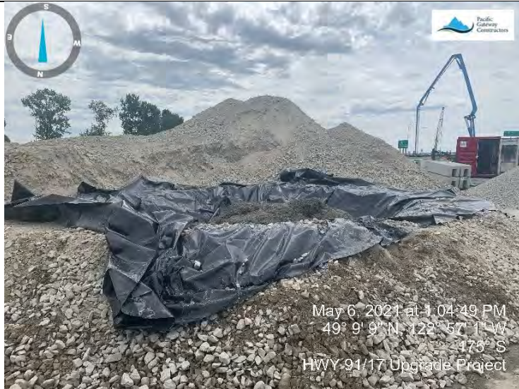
Photo 1. Section 1 Bridge west (C), temporary waste concrete management area.
