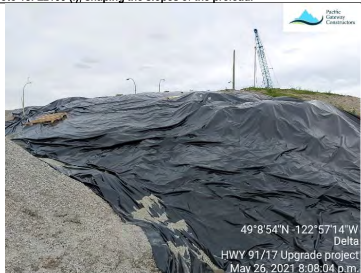
Photo 20. L550 (E), example of poly sheeting covering contaminated materials.
