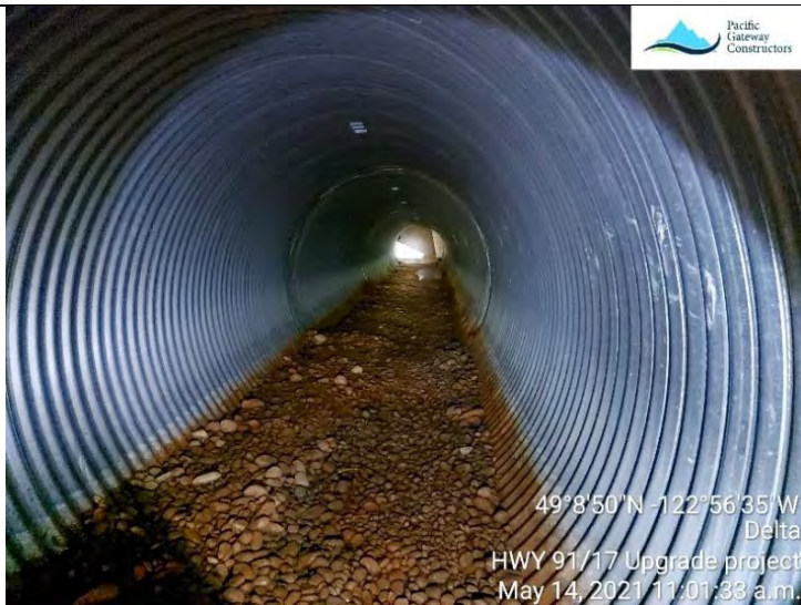
Photo 9. L550 (E), wildlife sweep at the old wildlife culvert prior to closure of the entrance with geo-textile fabric.
