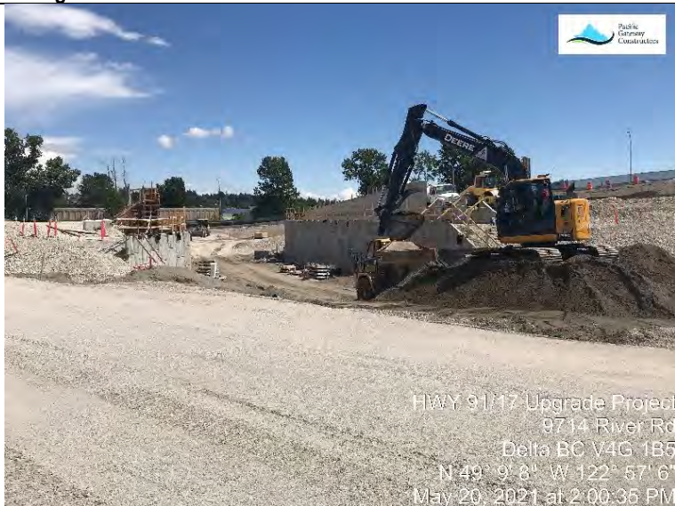
Photo 3. Section 1 Bridge (C), sand hauling and embankment fill placement.
