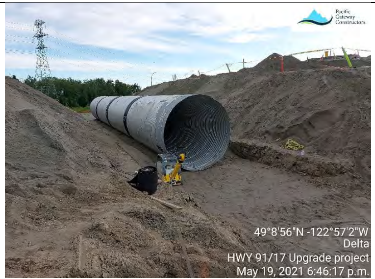
Photo 10. L500/L575 (E), general view culvert installation (wildlife crossing).
