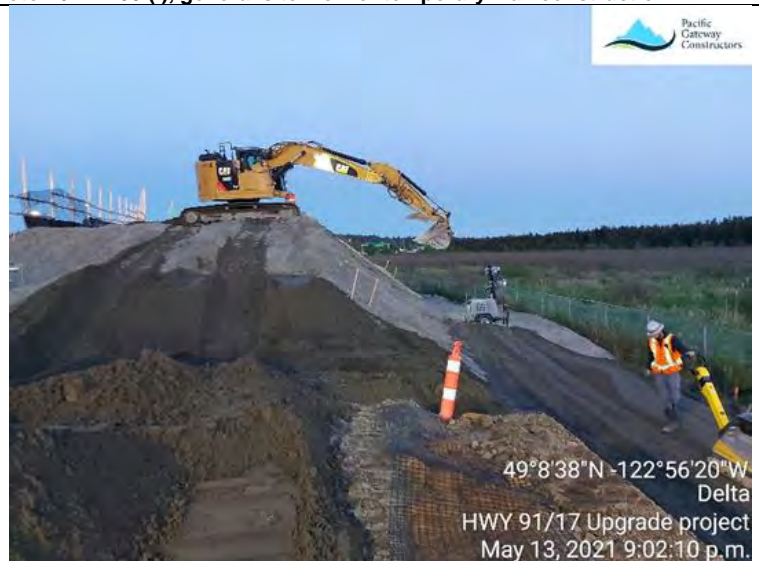
Photo 18. L2100 (I), shaping the slopes of the preload.
