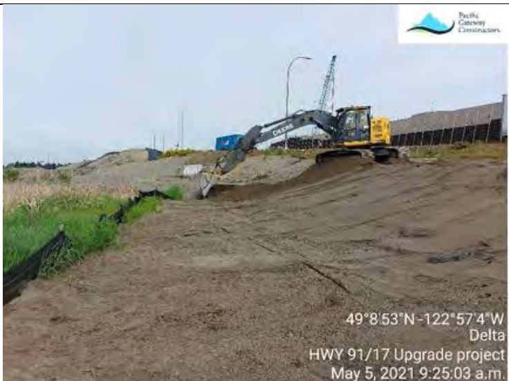
Photo 7. L550 (E), mitigation of steep slope and removal of sand migration in close proximity to the broject boundary. No sand was found in the stream and no instream works were done. ESC fences were inspected and found to be fully functional and keyed in.
