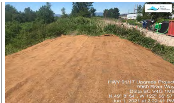
Photo 3: Excess material removed and exposed surfaces were stabilized with coco-matting
