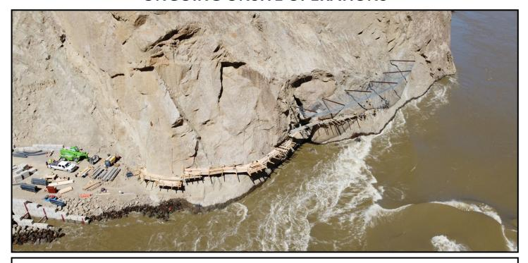
**PICTURED:** Work continues on the platform as part of the pneumatic fish pump system installation.
