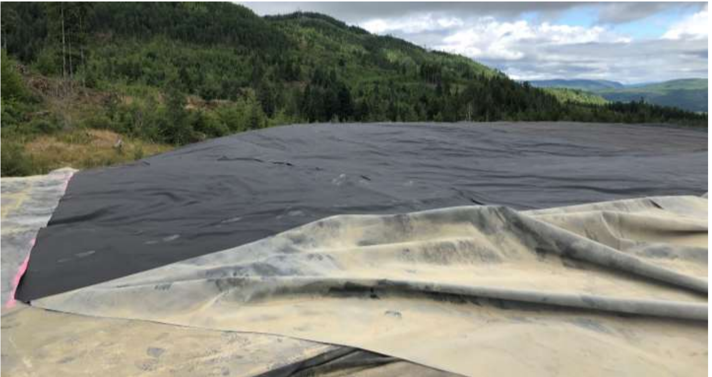
Picture # 4: 12 oz. geotextile deployed on crest of PEA (looking west).
