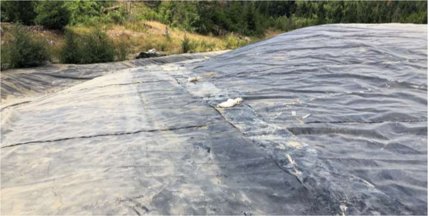
Picture # 3: Geomembrane patches placed on PEA crest.
