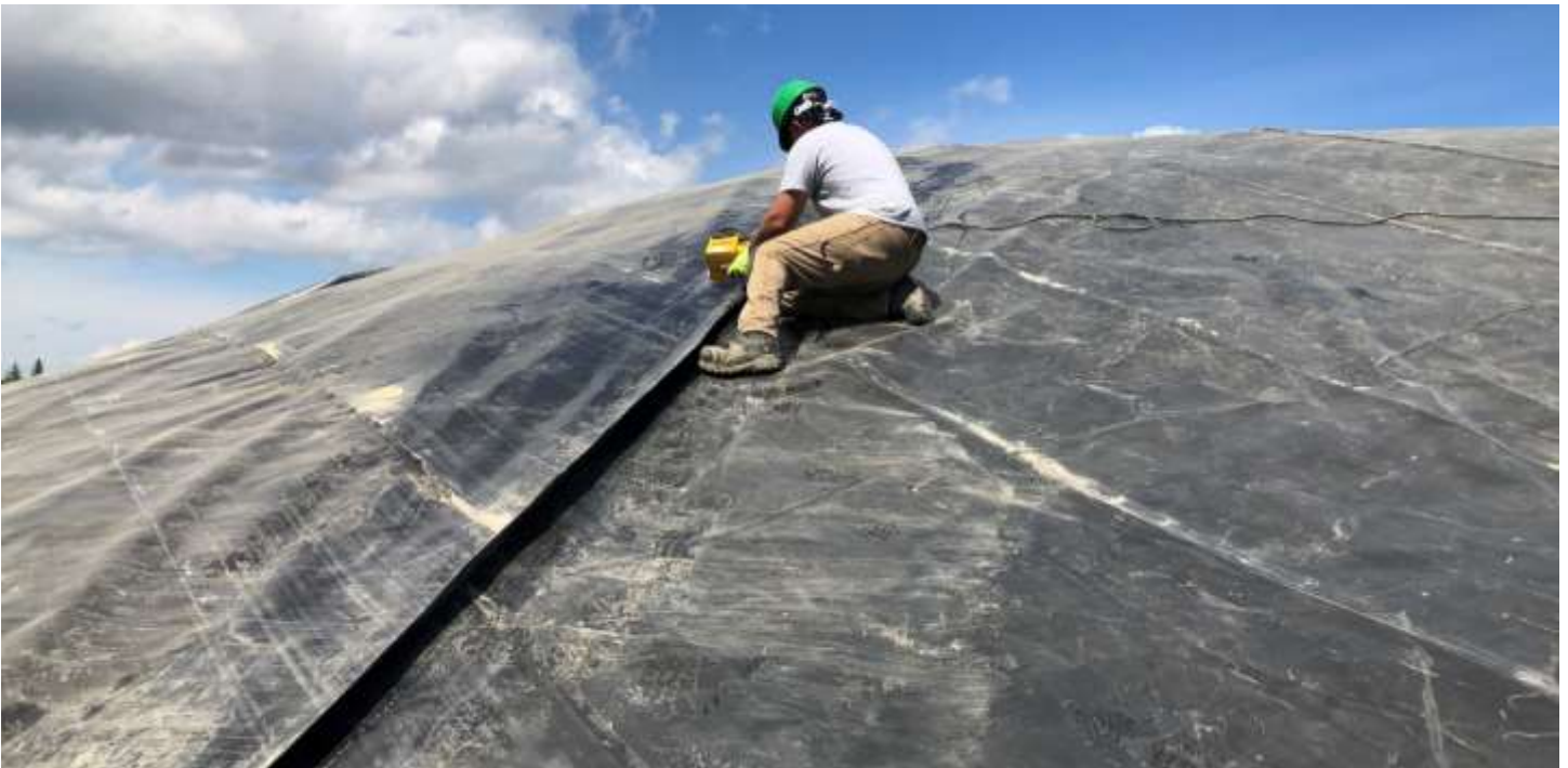
Picture # 12: WTL wedge welding previous wrinkle in geomembrane.
