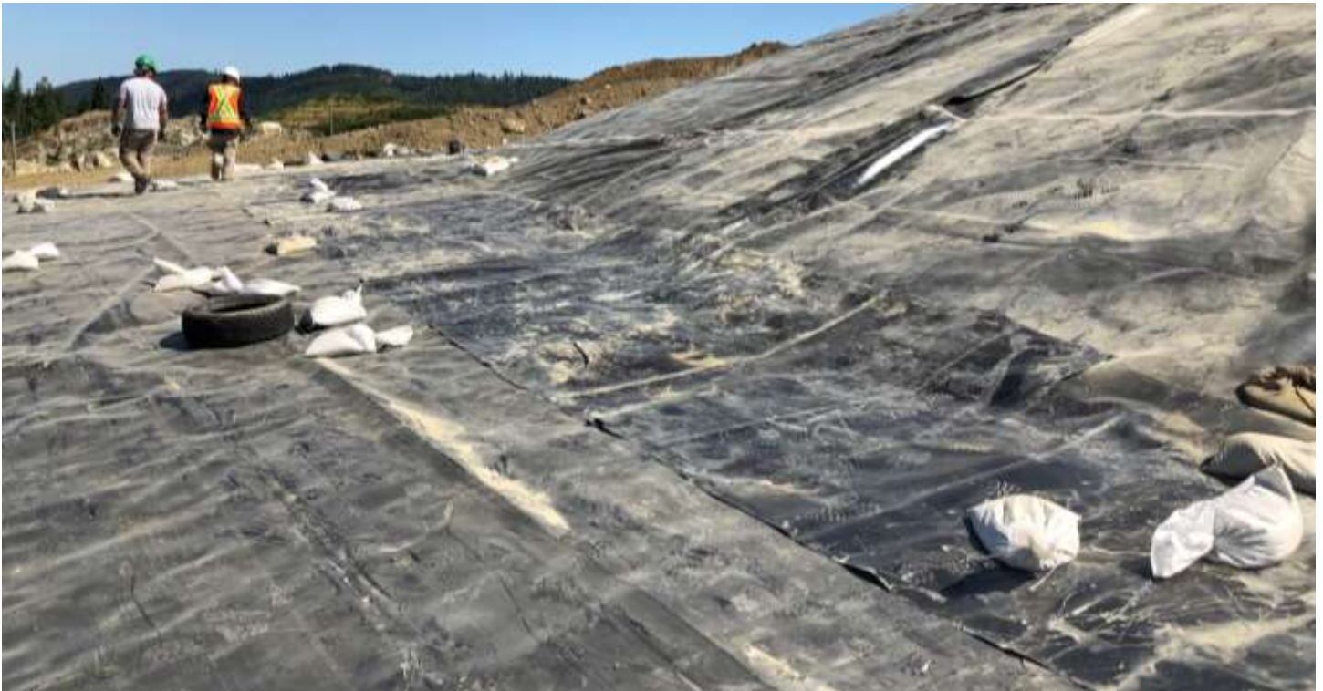
Picture # 9: Geomembrane patch on west side of PEA crest.
