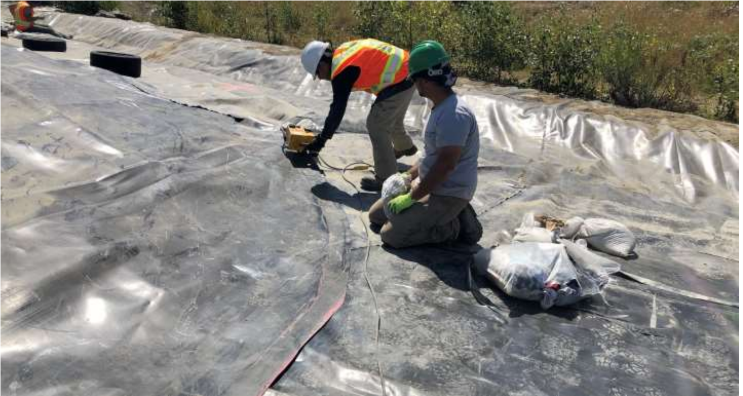
Picture # 11: WTL wedge welding patch on west side of PEA crest.
