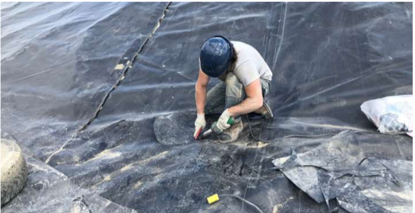
Picture # 6: WTL installing patch on geomembrane.
