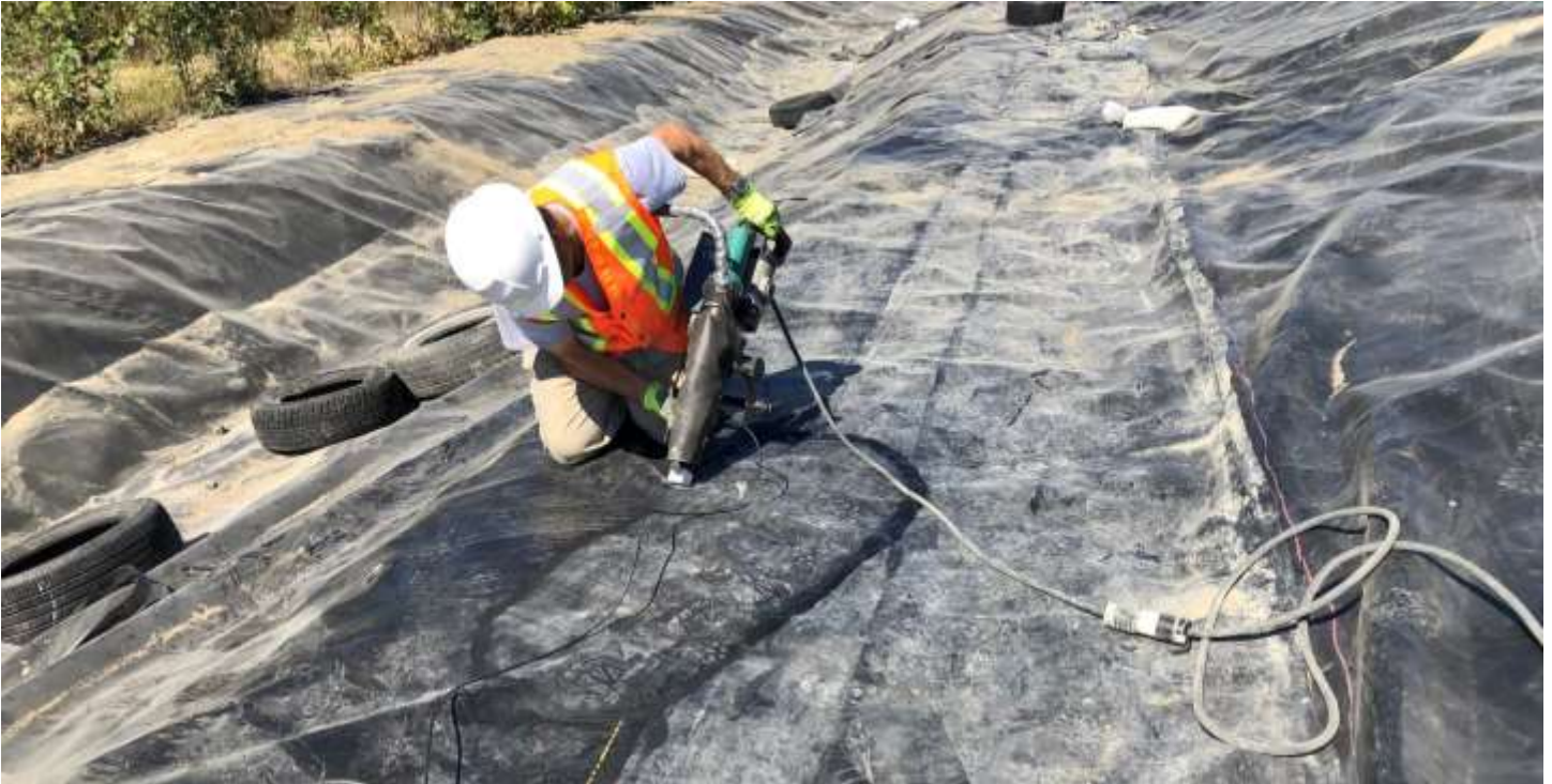
Picture # 9: WTL extrusion welding geomembrane patch on south crest of PEA.
