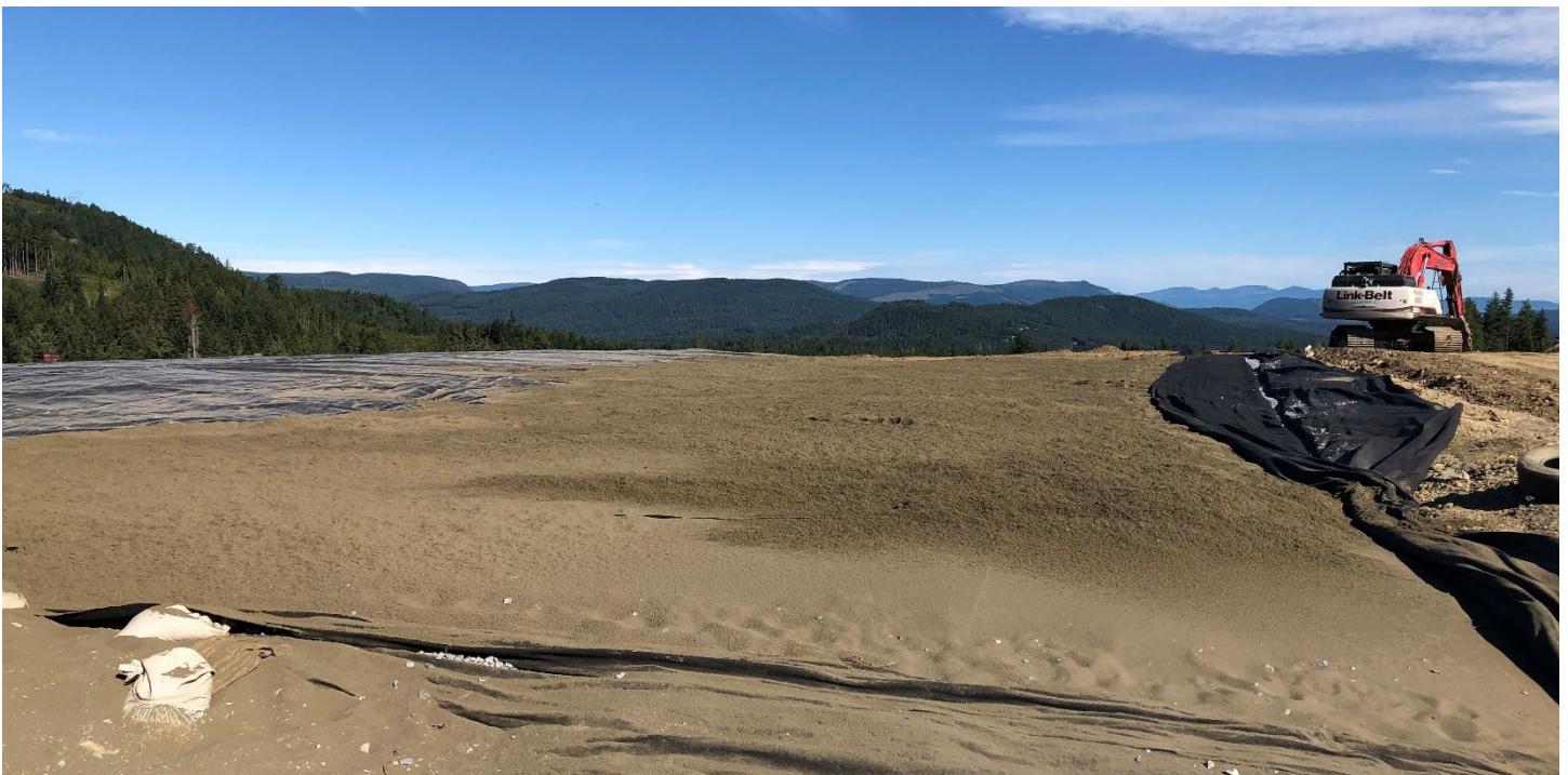
Picture # 2: 50mm thick sand layer placed on east crest of PEA.
