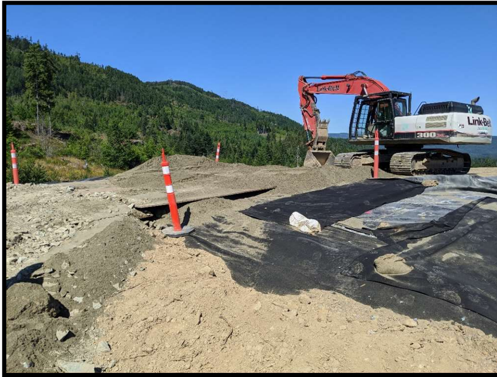
Picture #5: Sand bedding and road plates were used to create a bridge for hauling onto the exposed portion of the PEA.
