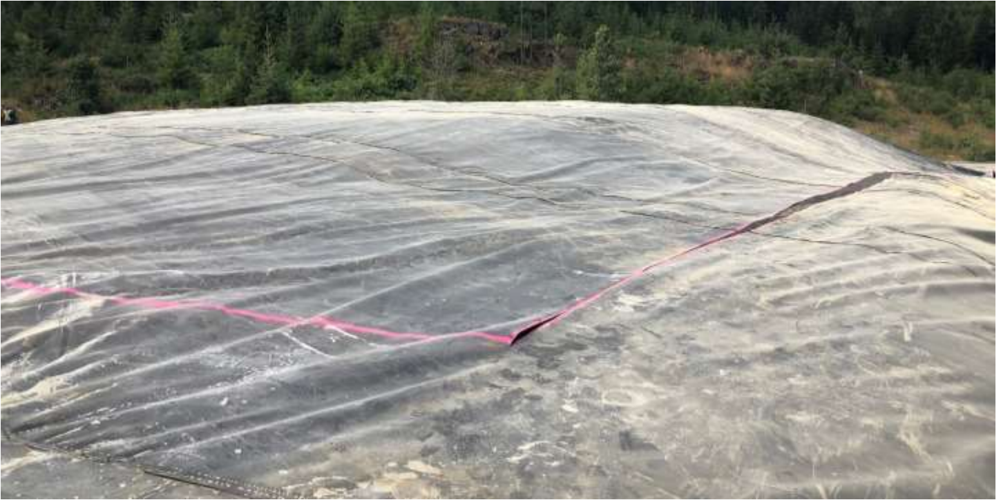
Picture #7: Geomembrane pulled back over crest of PEA.
