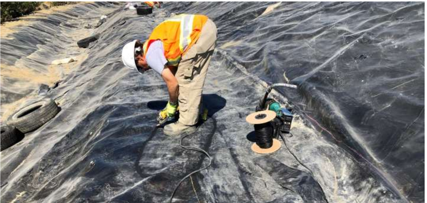
Picture # 8: WTL installing geomembrane patch on south crest of PEA.
