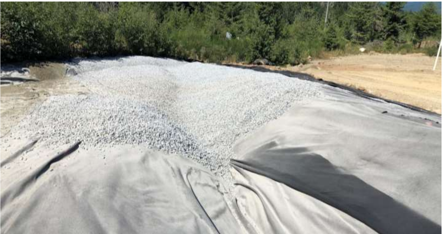
Picture # 16: Drainage gravel placed in northwest crest ditch above 12 oz. geotextile.
