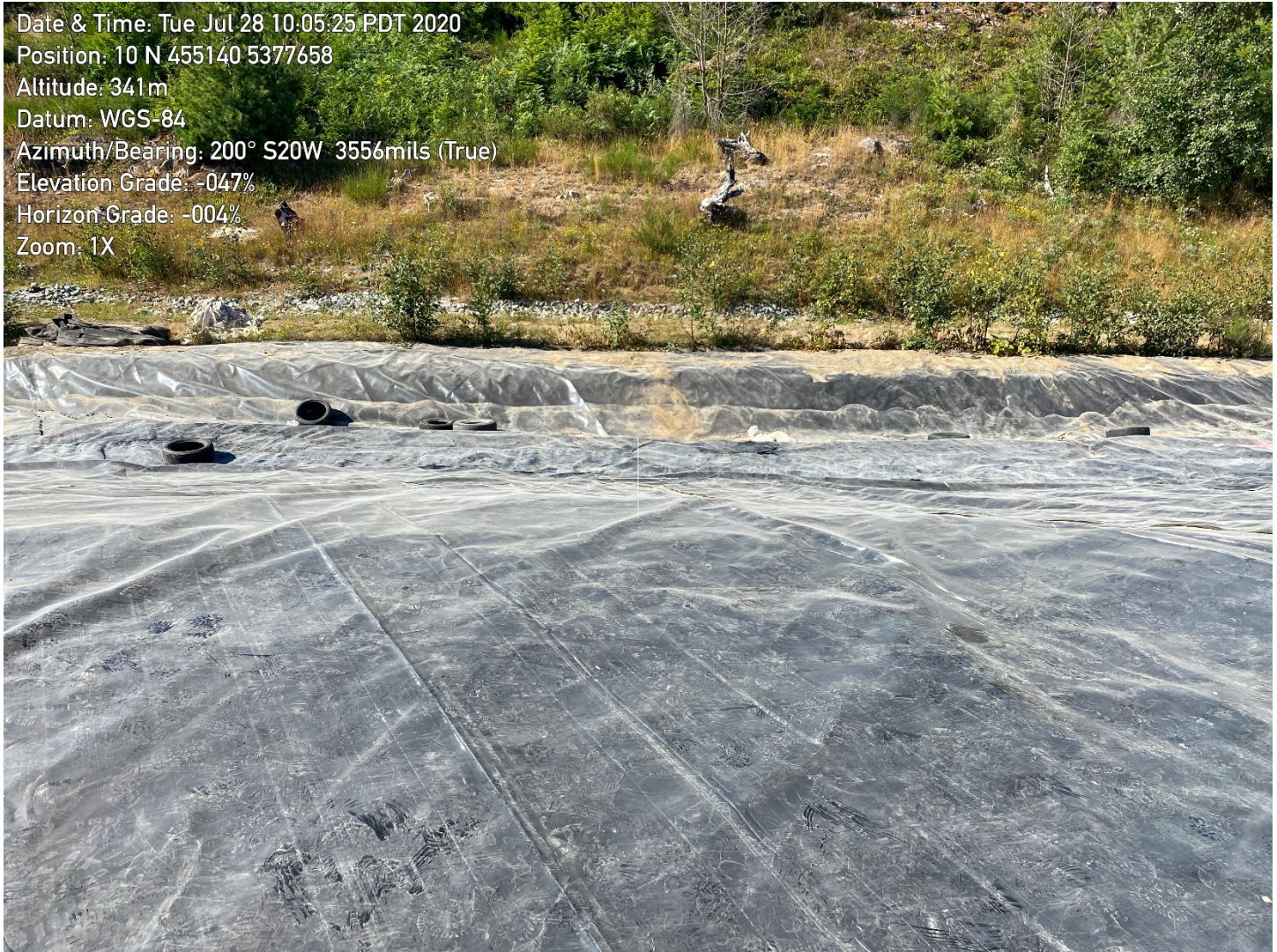
Picture # 10: Upon inspection of slope angles at the west and southwest sides of the crest of the PEA, it was found that the slopes are steeper than 3H:1V. SHA to discuss with Alterra design solution.
