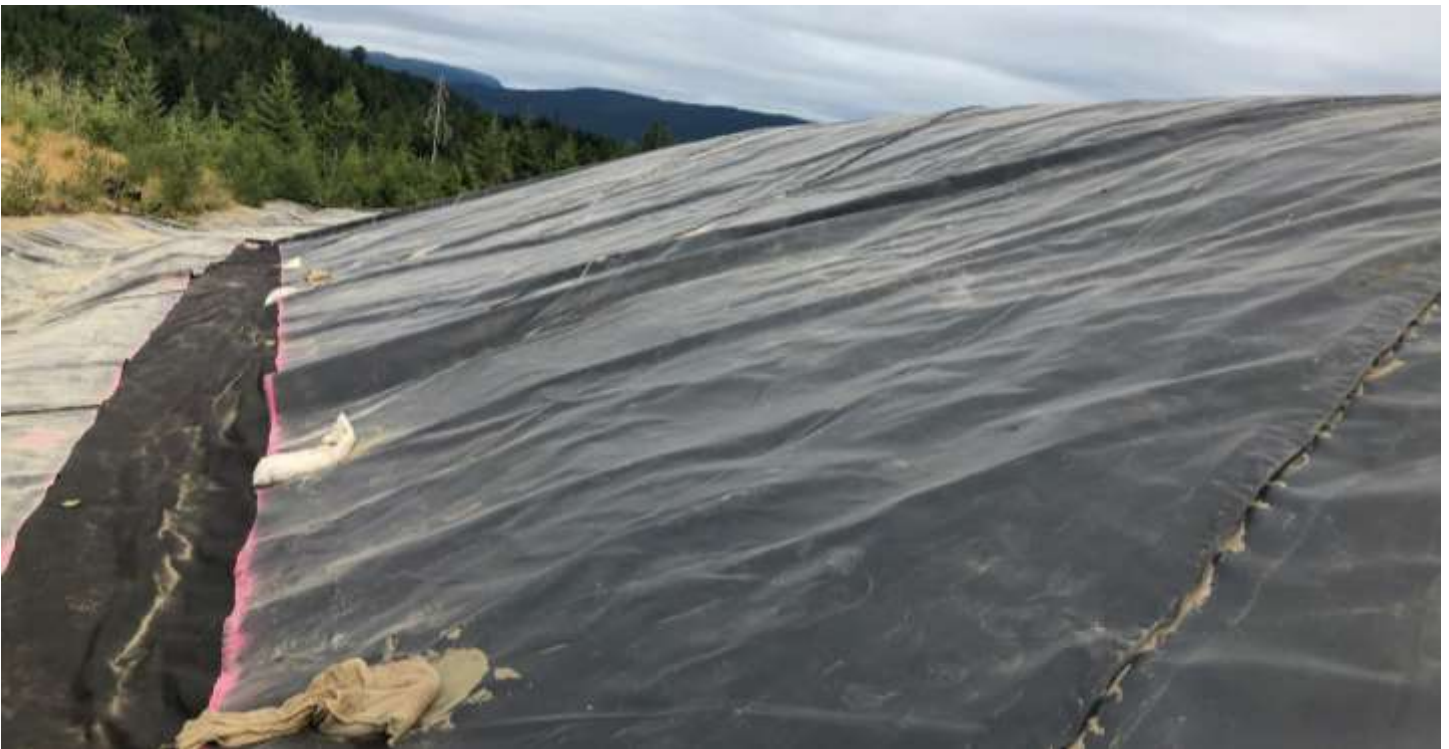
Picture # 10: Wrinkles in geomembrane at south side of PEA.
