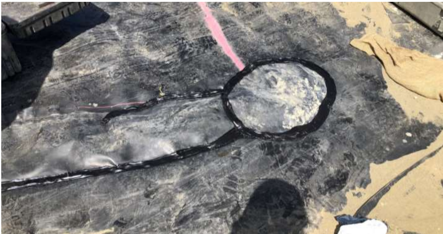
Picture # 13: Example of extrusion weld patch on geomembrane.
