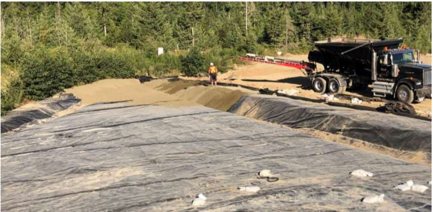
Picture # 12: Alterra using slinger to place 50mm thick sand layer on southwest crest of PEA. In some areas the sand was applied thicker than 50 mm so that it would not slide down the slopes of the ditch.
