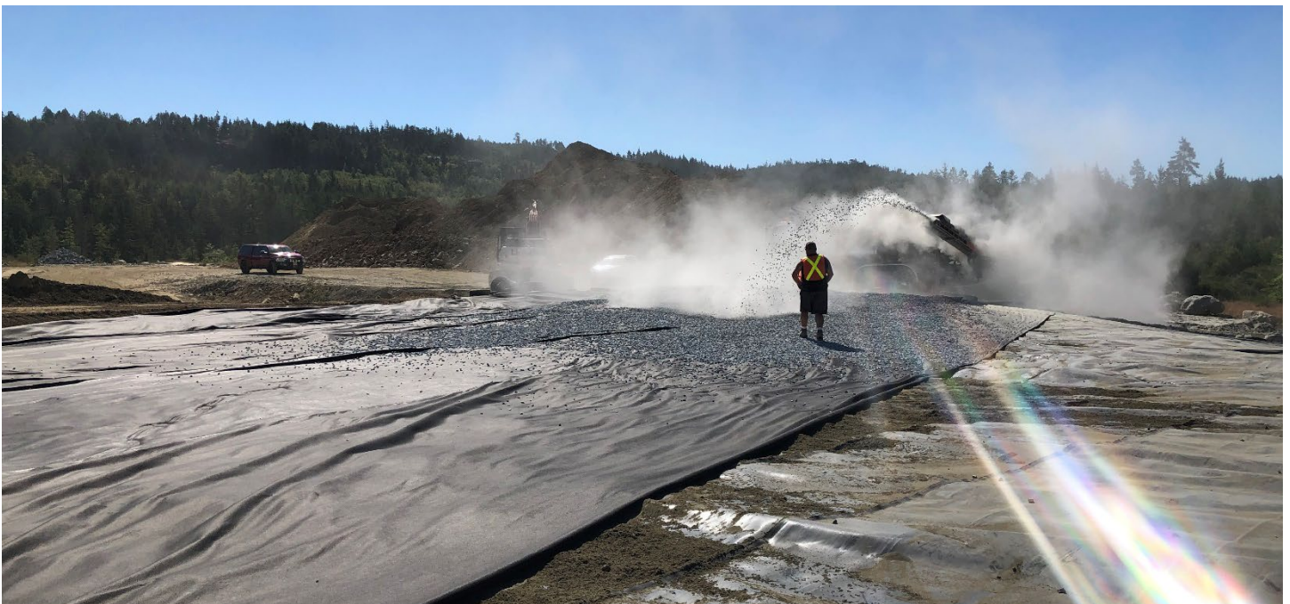
Picture # 5: Alterra using slinger to place 200mm thick layer of drainage gravel over 12 oz. geotextile on east crest of PEA.
