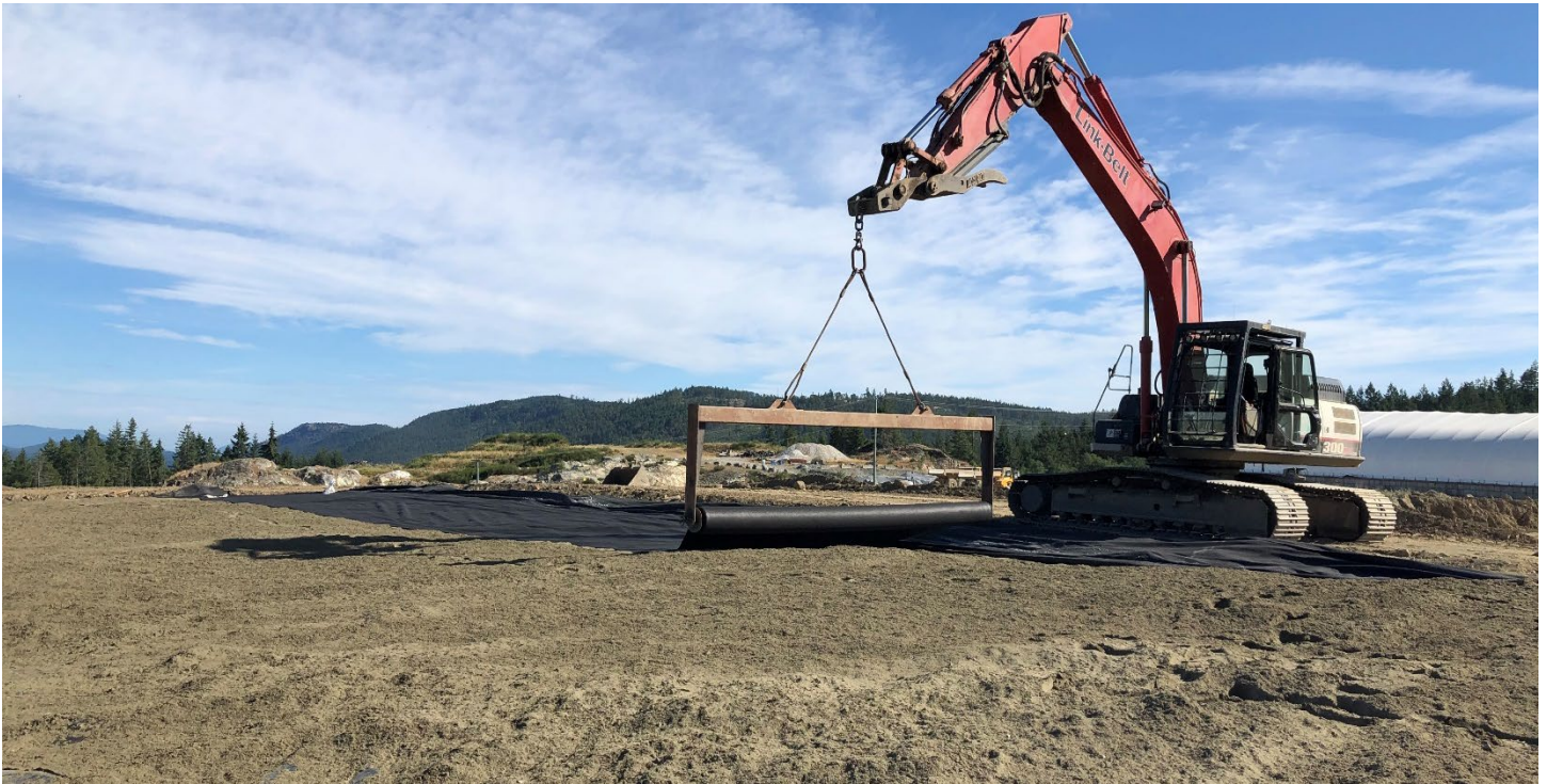
Picture # 3: Alterra deploying 12 oz. geotextile over sand layer on east crest of PEA.
