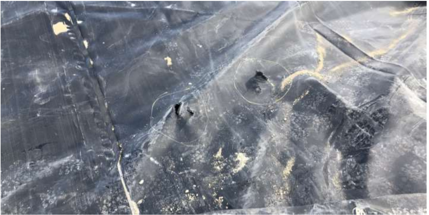
Picture # 5: Example of geomembrane damage requiring repair
