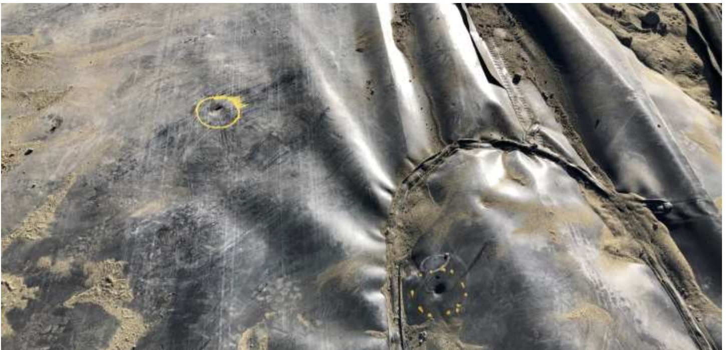
Picture # 4: Examples of geomembrane damage marked for repair
