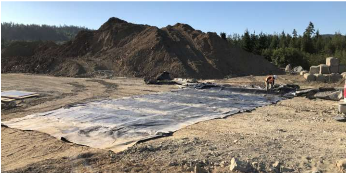
Picture # 1: Geomembrane used for patching geomembrane on PEA
