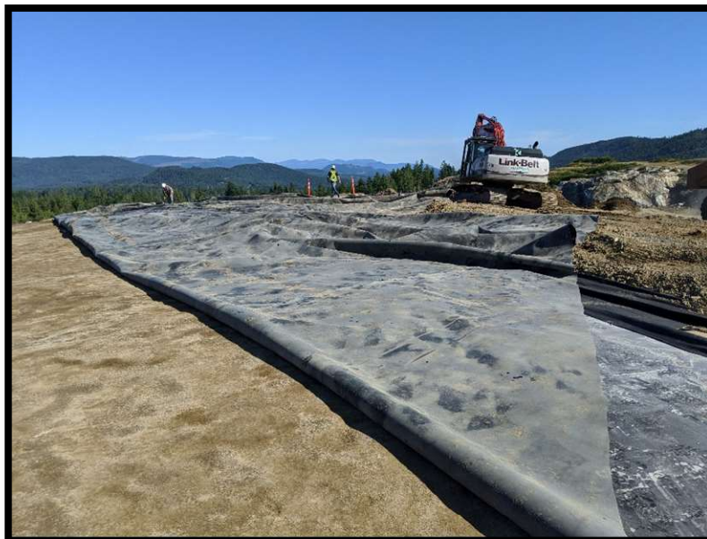
Picture # 1: Contractor began using quads to initially peel back the PEA membrane. The membrane was cut along three sides and peeled back in a single piece.
