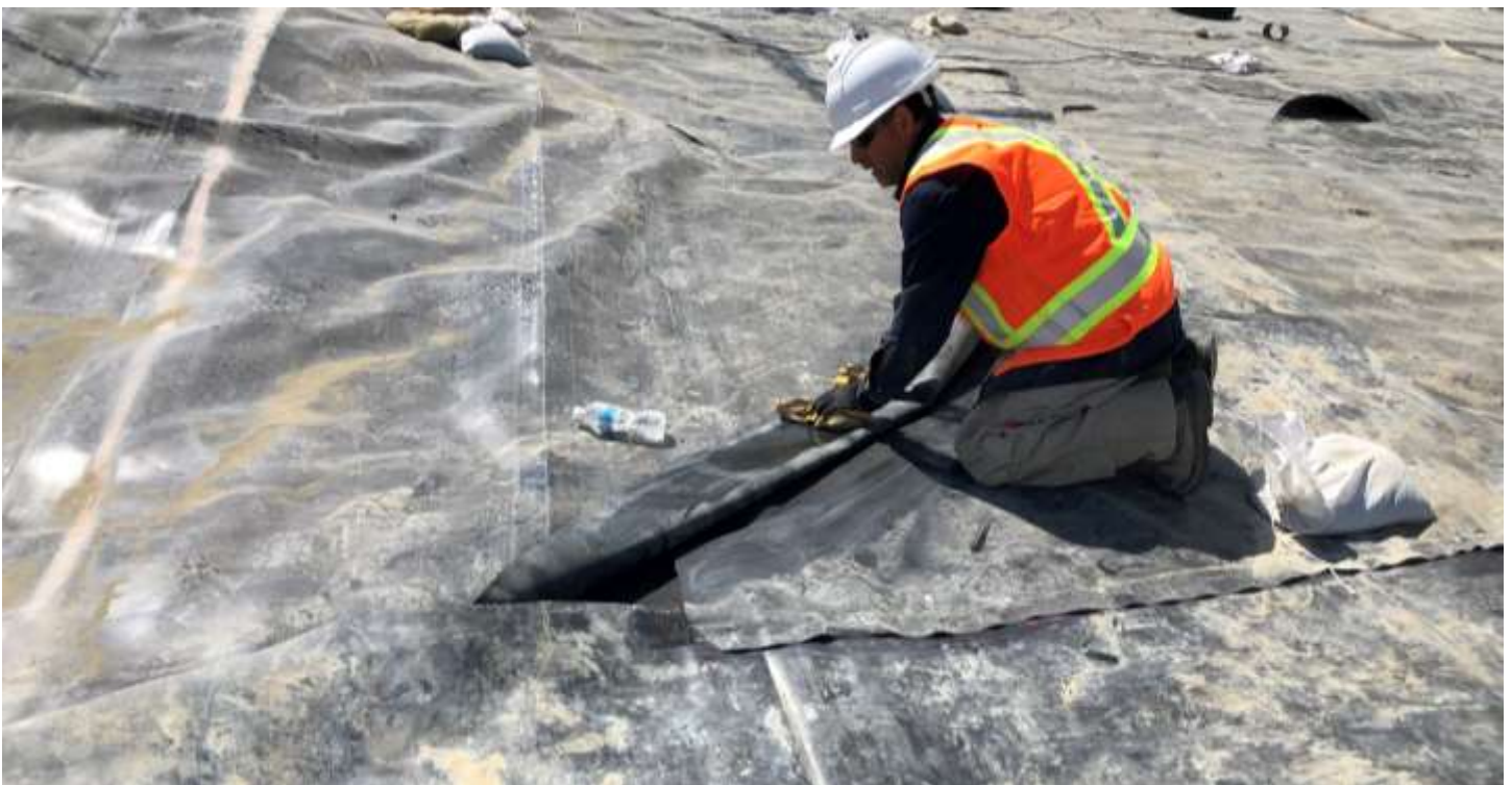
Picture # 10: WTL cleaning geomembrane prior to wedge welding to ensure integrity of weld.
