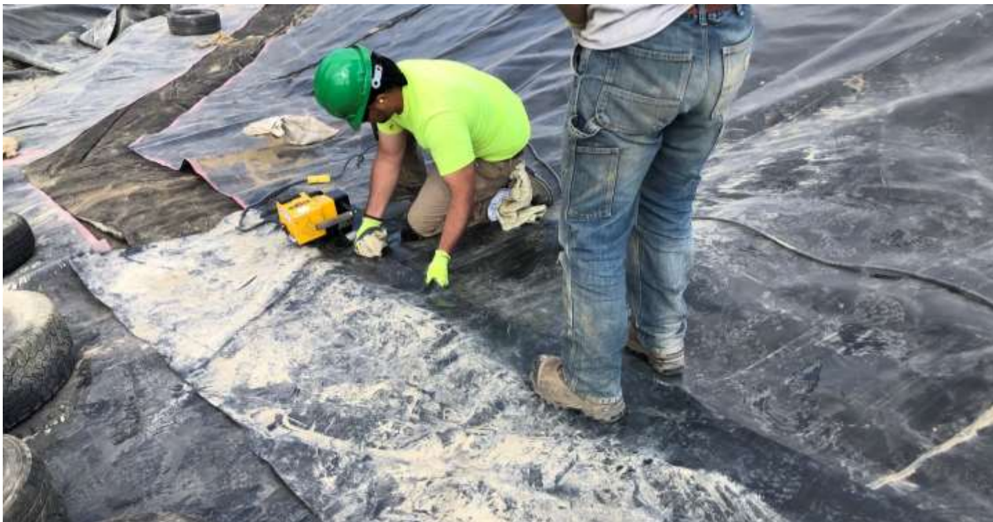
Picture # 3: WTL wedge welding geomembrane patch on crest of PEA.
