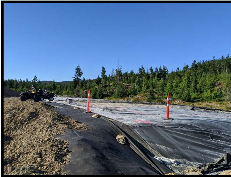
Picture # 1: Contractor began using quads to initially peel back the PEA membrane. The membrane was cut along three sides and peeled back in a single piece.
