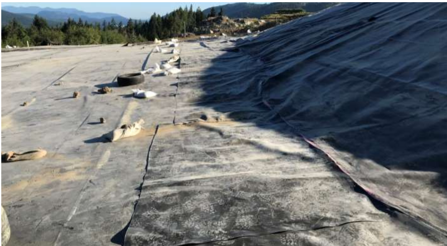
Picture #6: Geomembrane patch on west crest of PEA.
