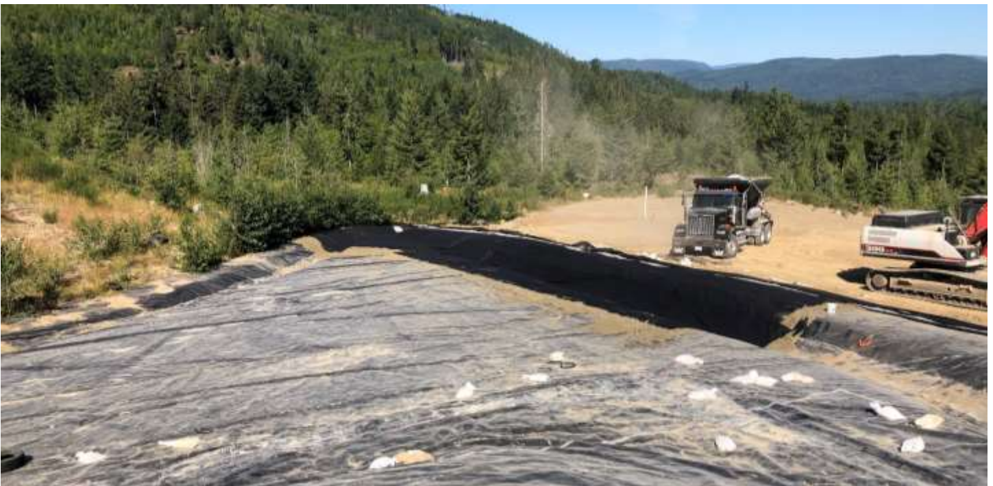
Picture # 14: Alterra deployed 12 oz. geotextile above sand layer at northwest crest ditch.
