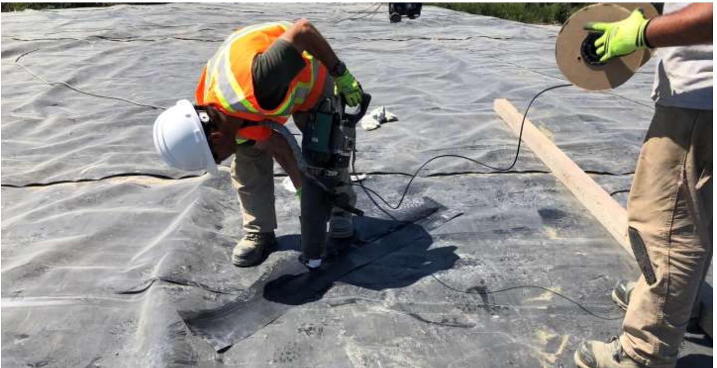
Picture #8: WTL re-qualifying the extrusion welder in the afternoon due to high outdoor temperatures.
