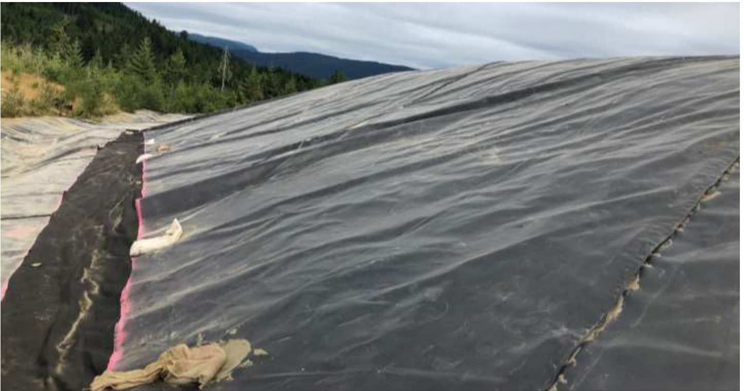
Picture #8: Gap between geomembrane after pulling back over crest of PEA.
