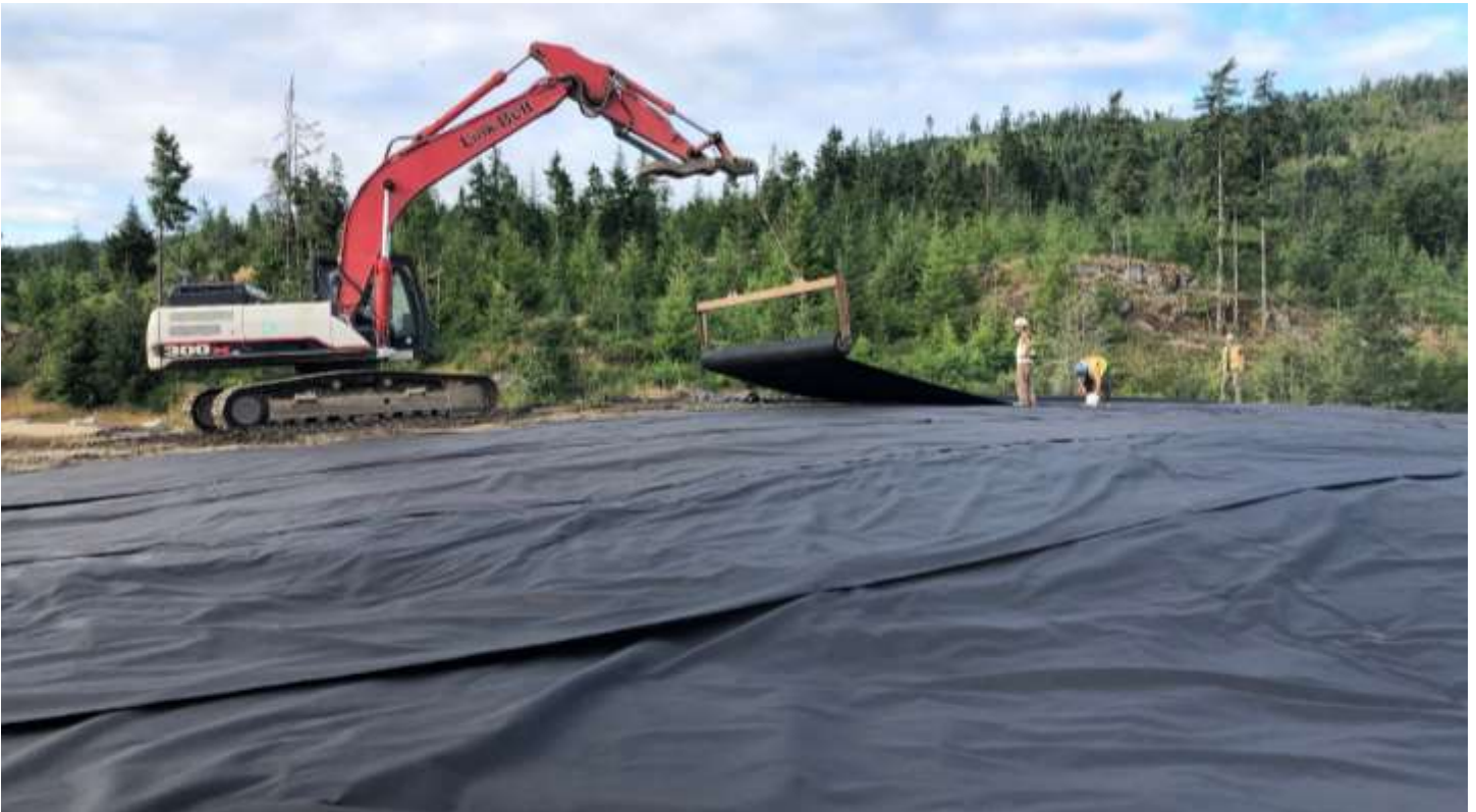
Picture # 2: Allterra deploying 12 oz. geotextile on crest of PEA.
