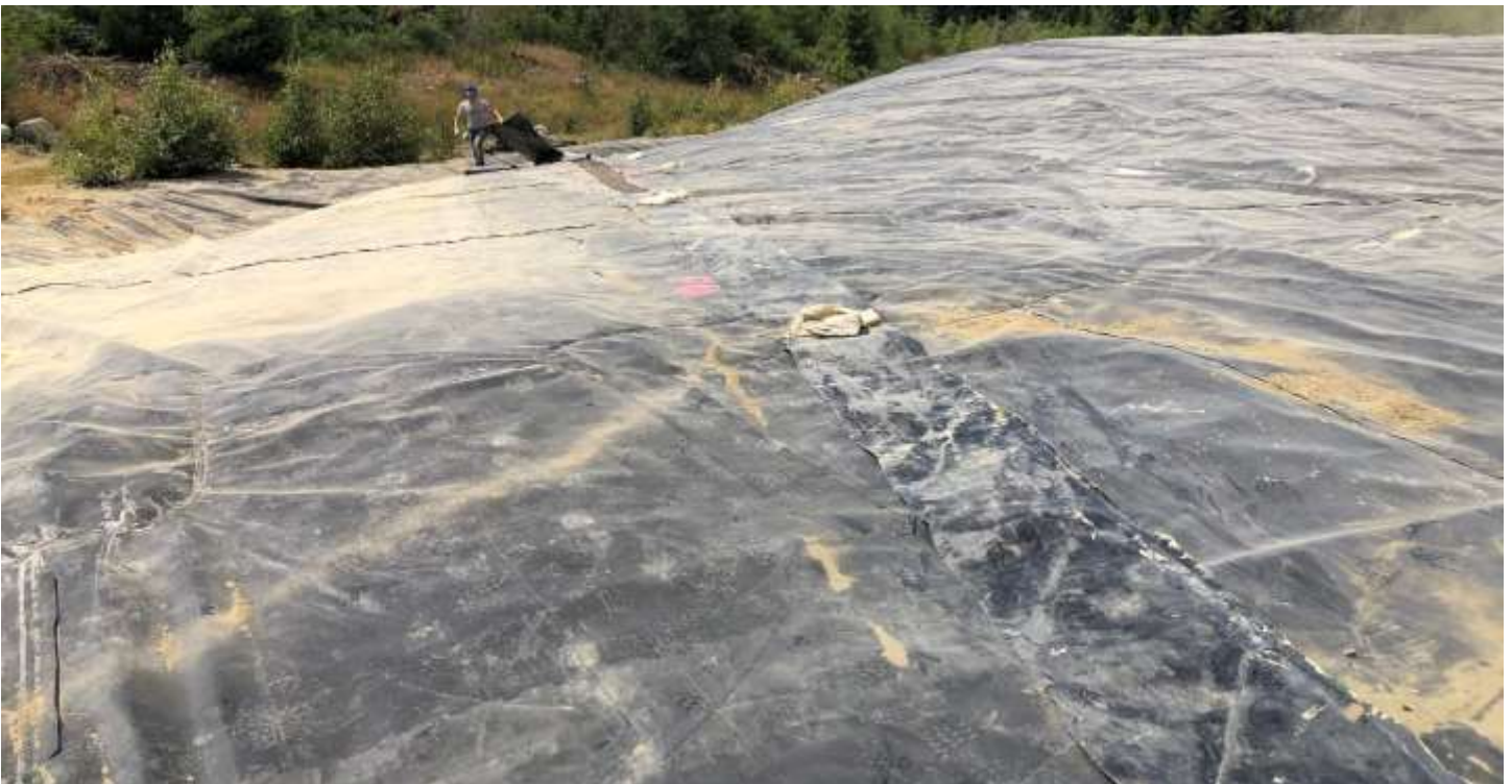
Picture # 2: Geomembrane patches placed on PEA crest.
