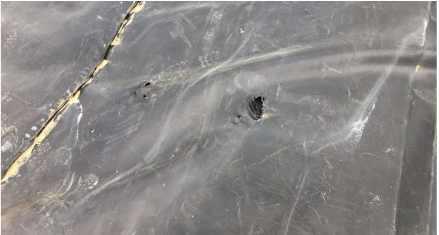
Picture #9: Example of damage to geomembrane from pulling over crest of PEA. Damages were identified for repair.
