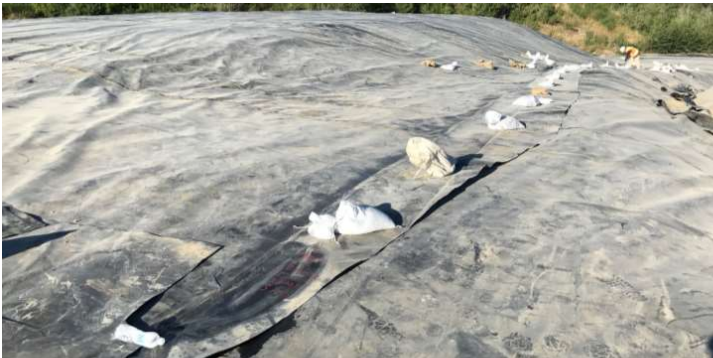
Picture # 5: Geomembrane patch on north crest of PEA.
