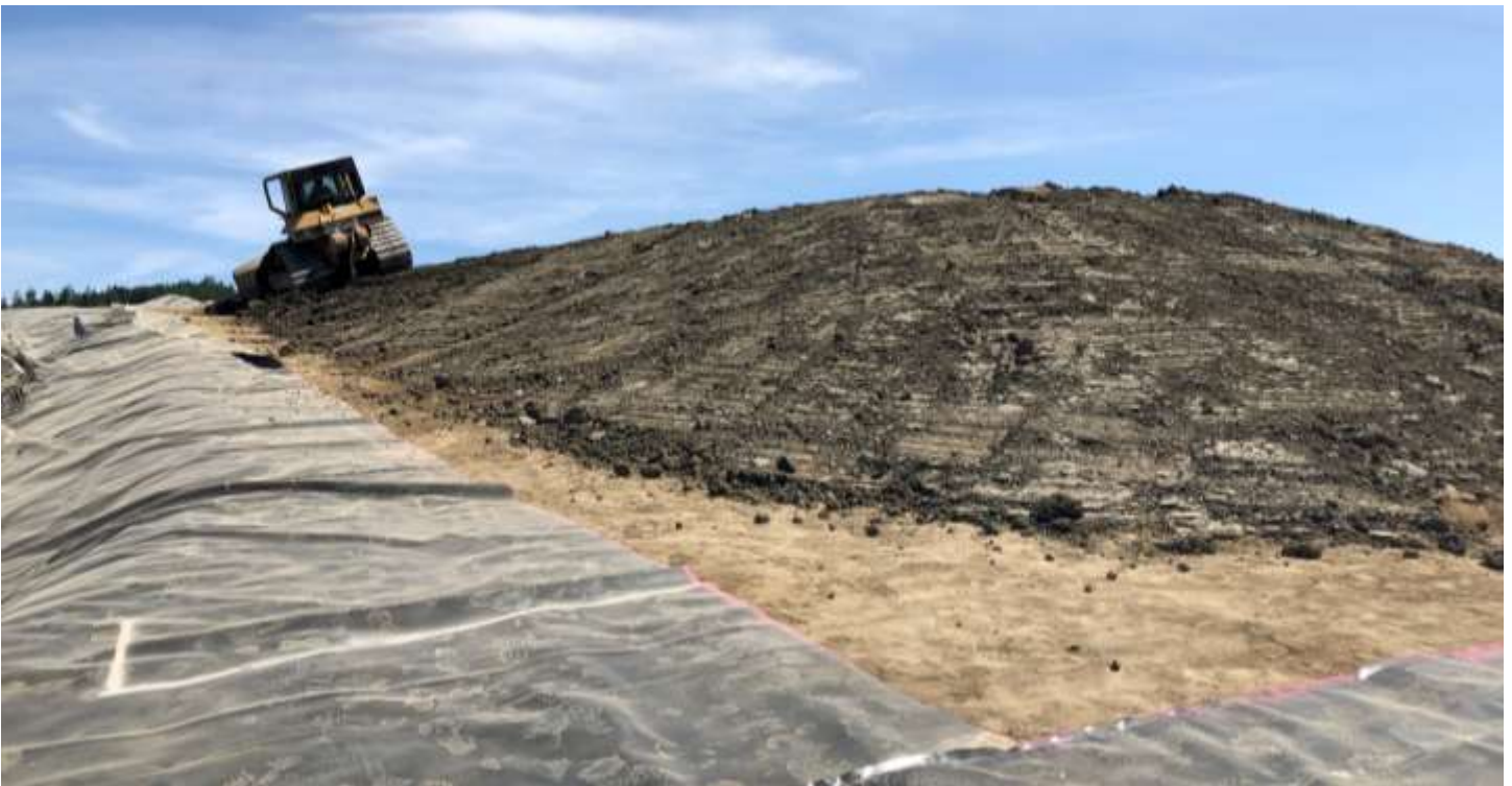
Picture #6: Allterra grading waste soils on crest of PEA.
