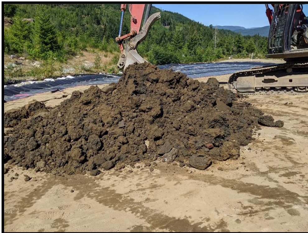
Picture #6: Previously stored on-site contaminated material was transferred to the exposed portion of the PEA. Hauling of the on-site contaminated material occurred throughout the day.
