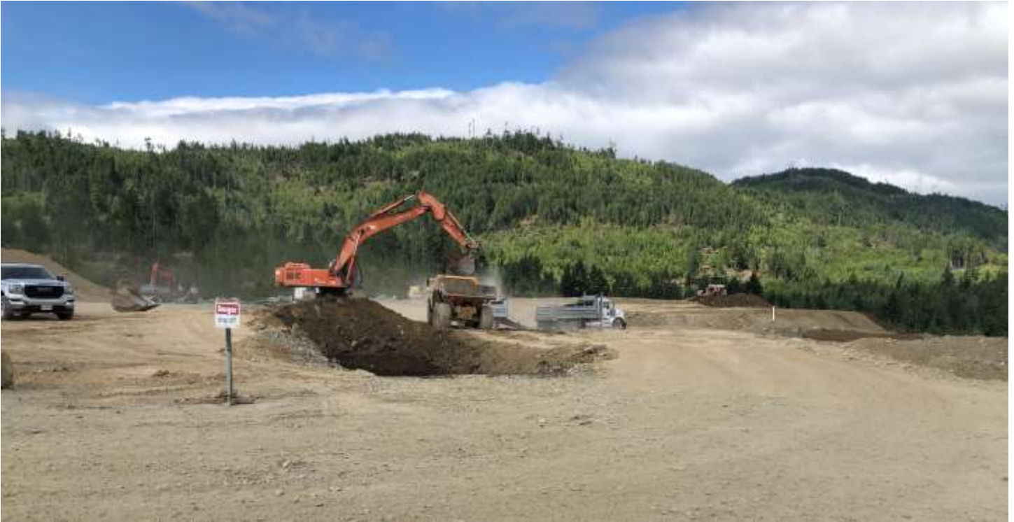
Picture # 7: Alterra excavating and relocating on-site soils
