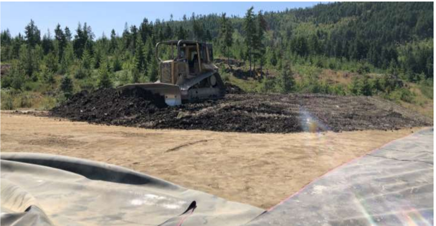
Picture # 4: Allterra spreading waste soils on crest of PEA.
