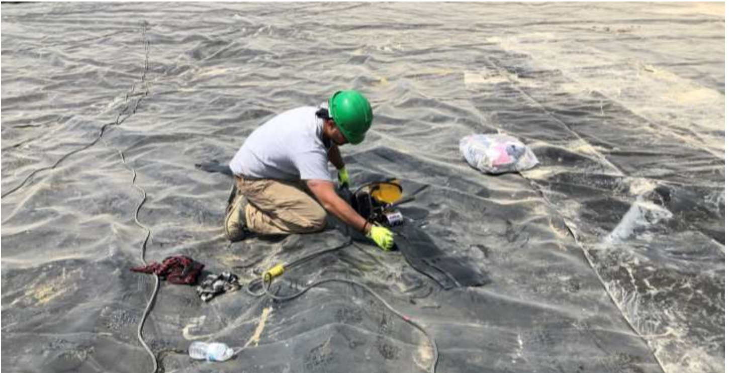
Picture # 5: Western Tank & Lining (WTL) qualifying wedge welder by welding test strips.
