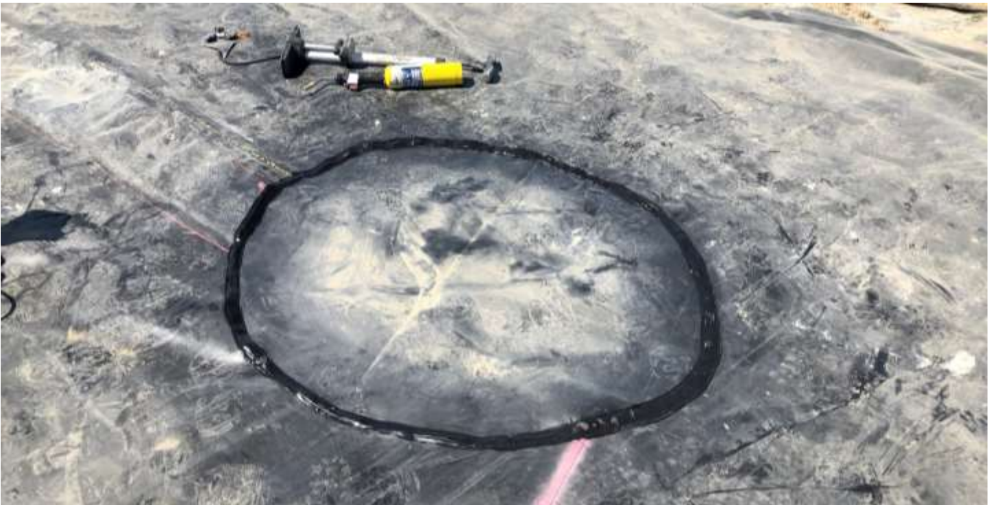
Picture #10: Example of extrusion welded patch on geomembrane.
