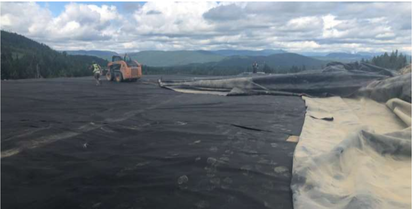
Picture # 6: Alterra pulling geomembrane back over crest of PEA.
