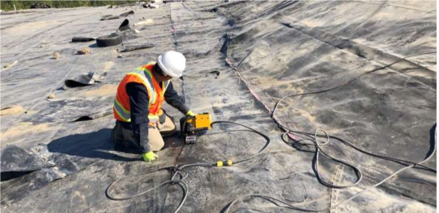
Picture # 7 : WTL wedge welding geomembrane on west crest of PEA.
