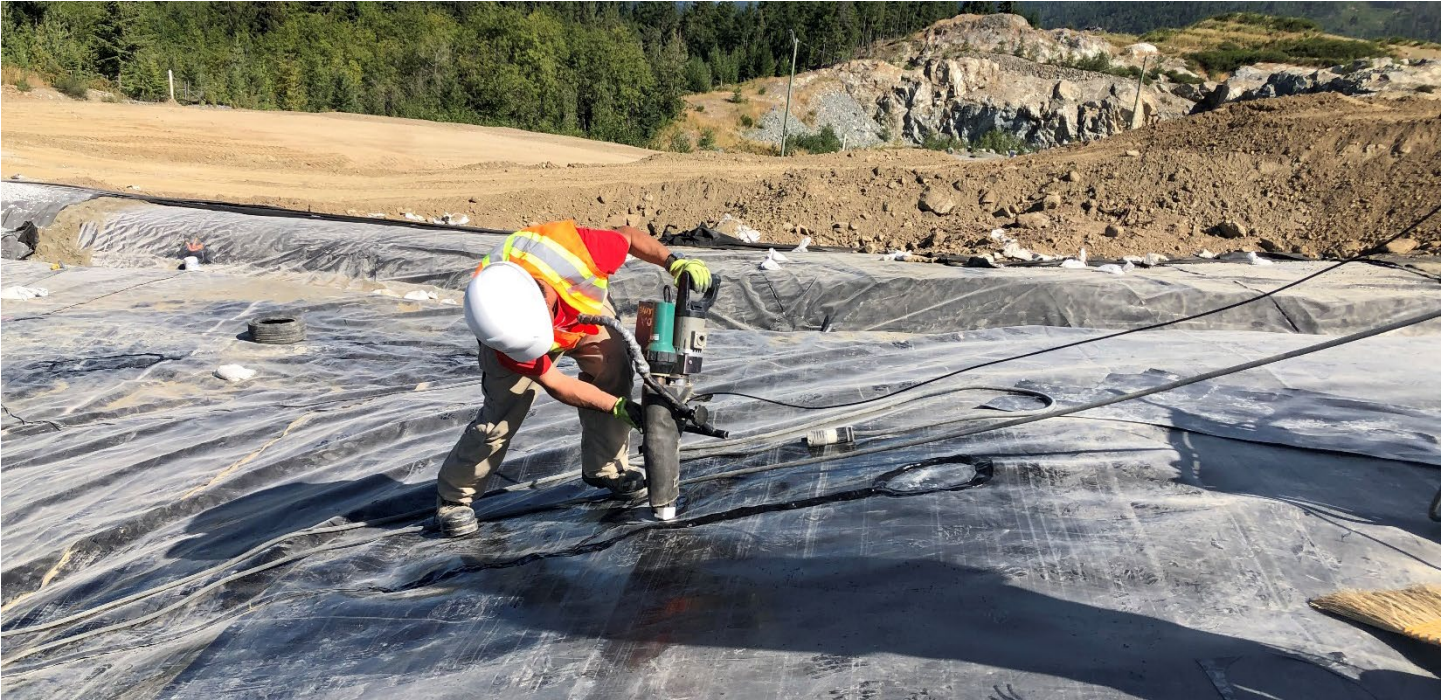
Picture # 6: WTL extrusion welding repair on geomembrane on crest of PEA.
