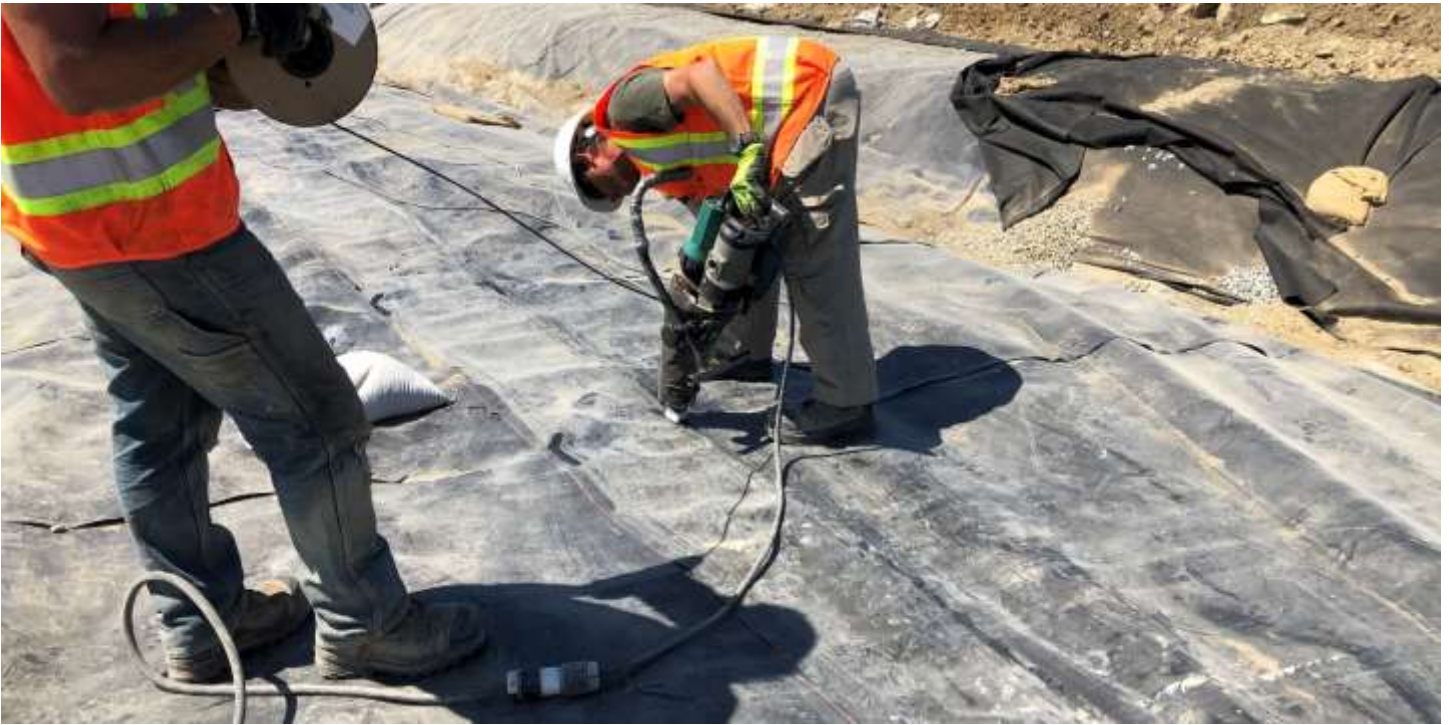
Picture #9: WTL performing extrusion weld.
