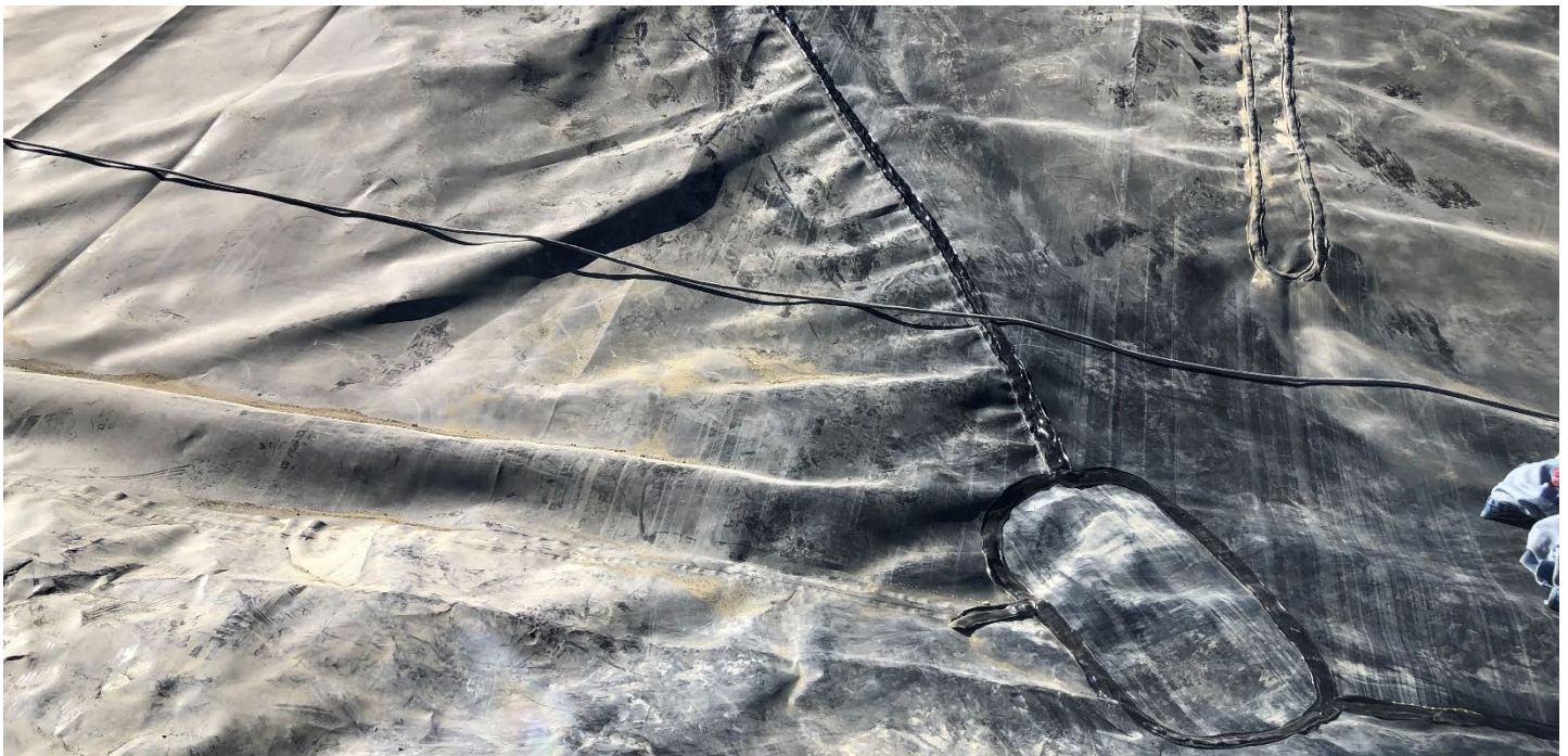
Picture # 7: Extrusion welded repair on geomembrane.
