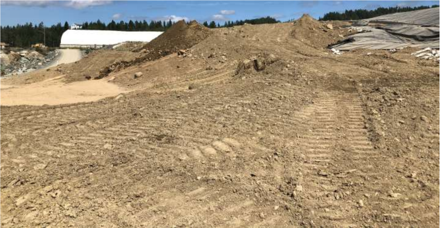
Picture # 15: Alterra relocated common fill to north side of PEA.
