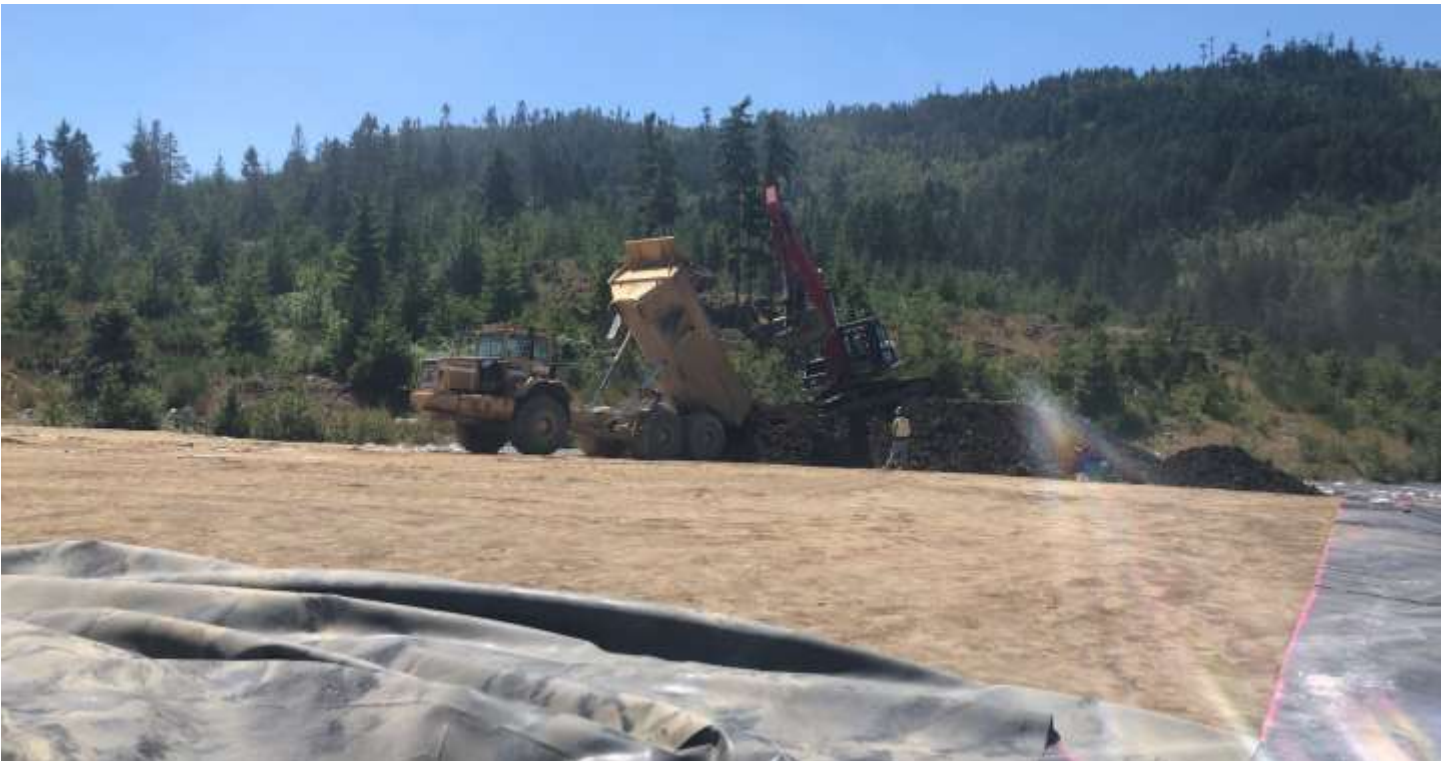
Picture # 2: Alterra dumping waste soils on crest of PEA.
