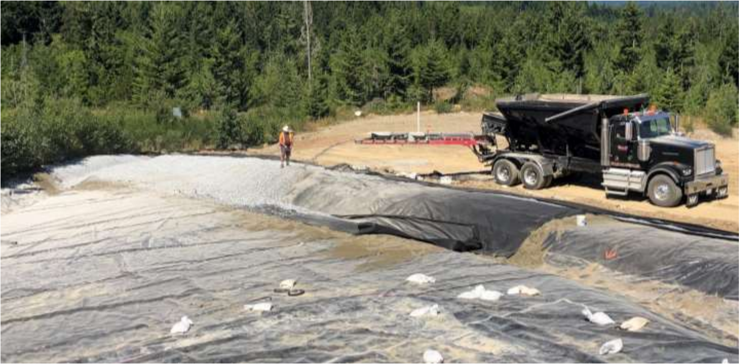
Picture # 15: Alterra placing 200 mm thick layer of drainage gravel in northwest crest ditch above 12 oz. geotextile.
