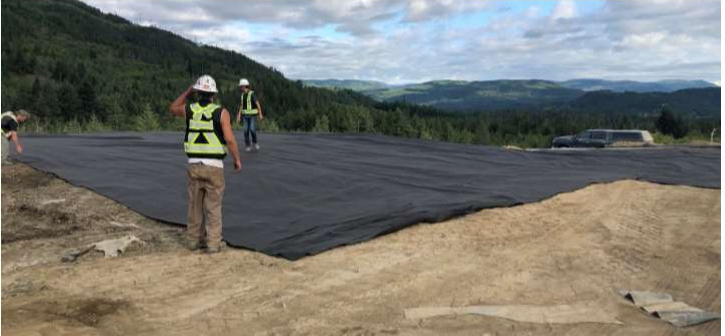
Picture # 1: Allterra deploying 12 oz. geotextile on crest of PEA
