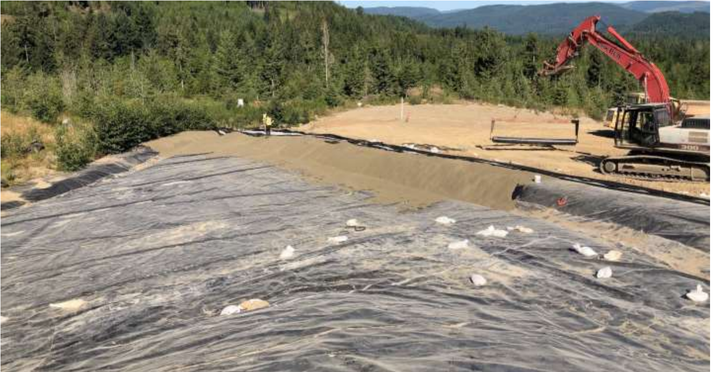
Picture # 13: Sand placed in ditch at northwest crest of PEA.
