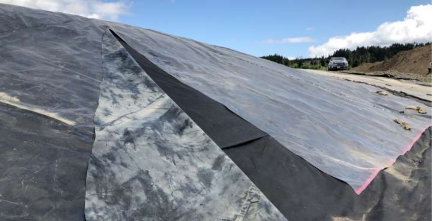
Picture # 11: The wrinkles in the geomembrane were cut so that the geomembrane could be welded such that the geomembrane would lie flat.
