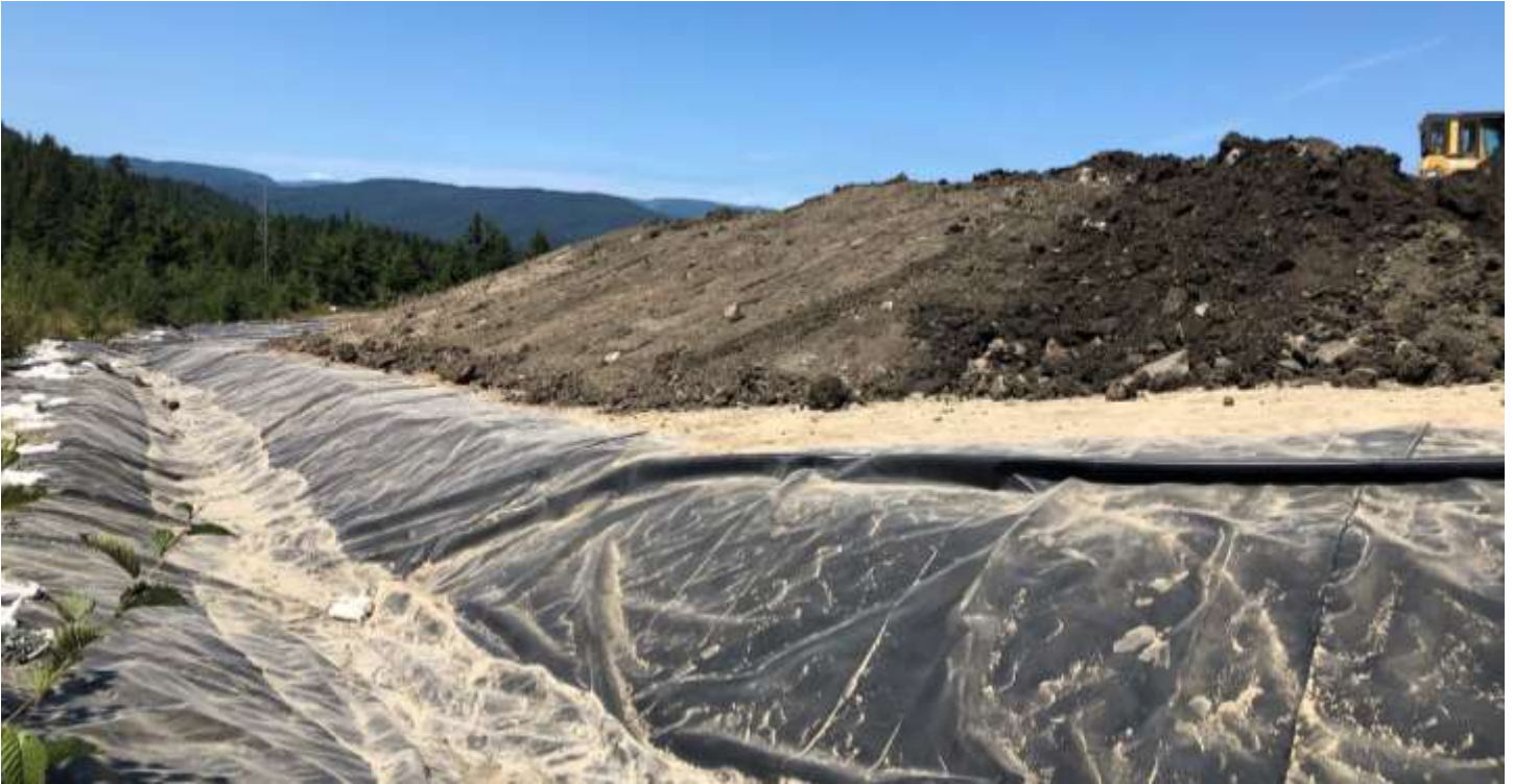
Picture #5: Allterra grading waste soils on crest of PEA.
