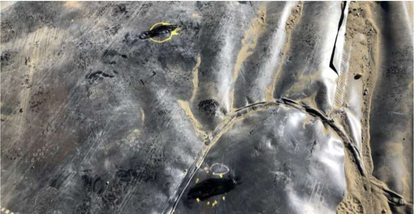
Picture #5: Small repairs with extrusion welder on geomembrane liner.
