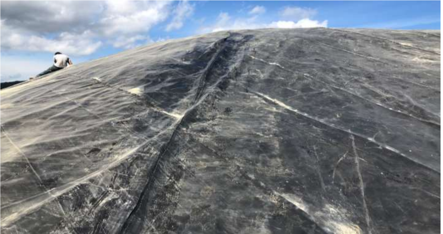
Picture # 13: Completed wedge weld.
