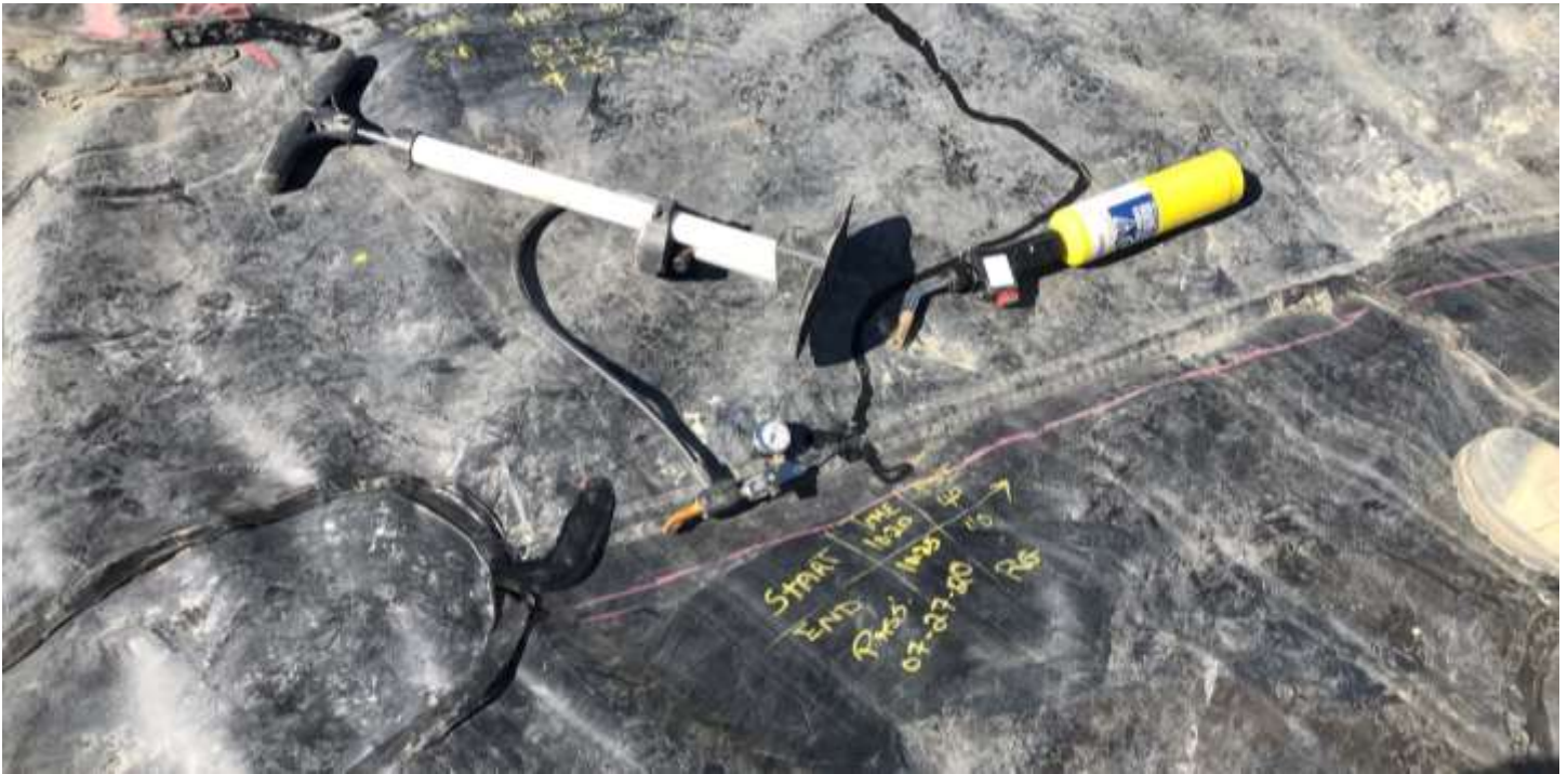
Picture #7: Example of air test results. Pressurized to 40 psi for 5 minutes. Passed.
