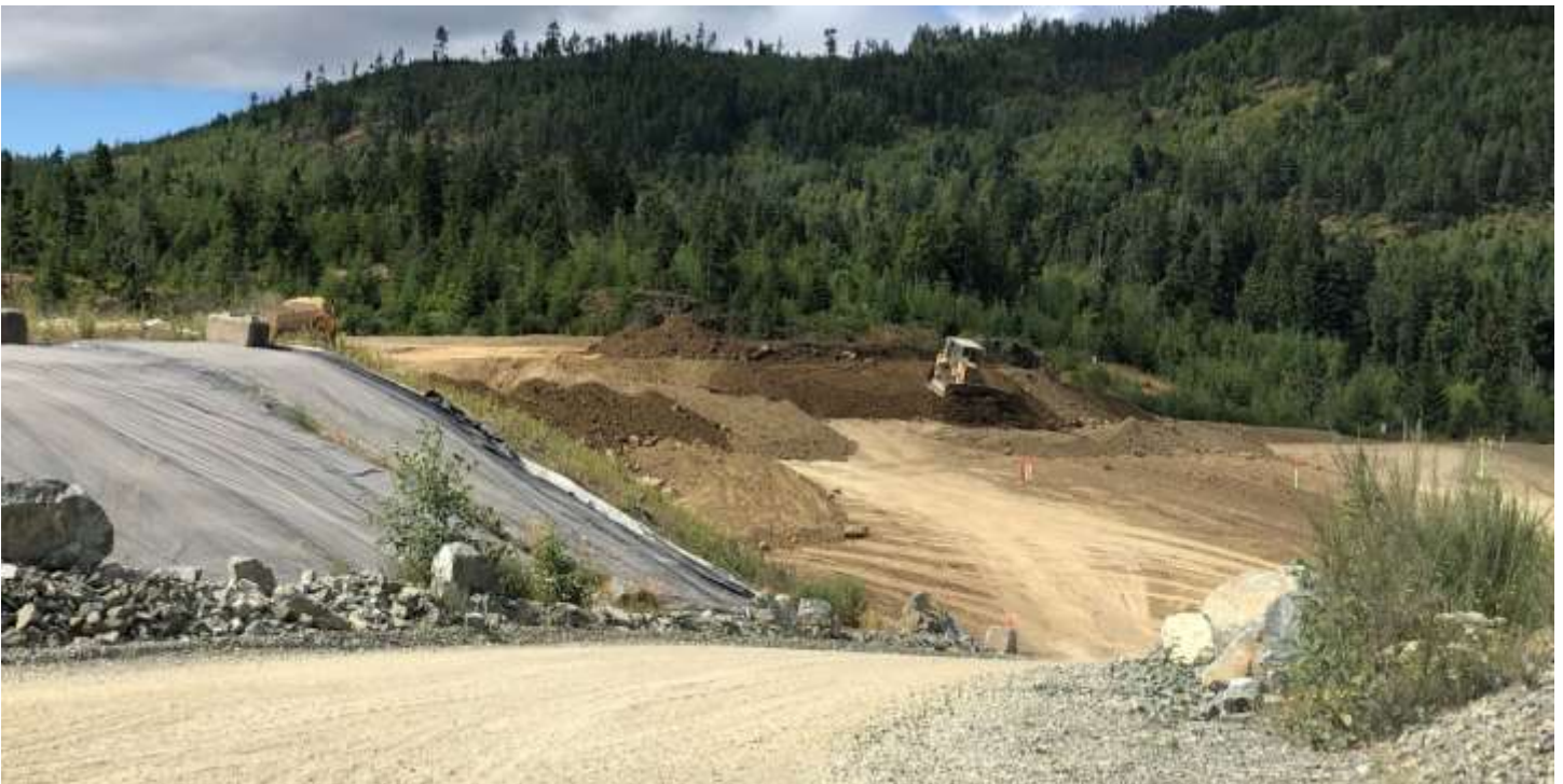
Picture # 8: Alterra grading soils on north slope of PEA
