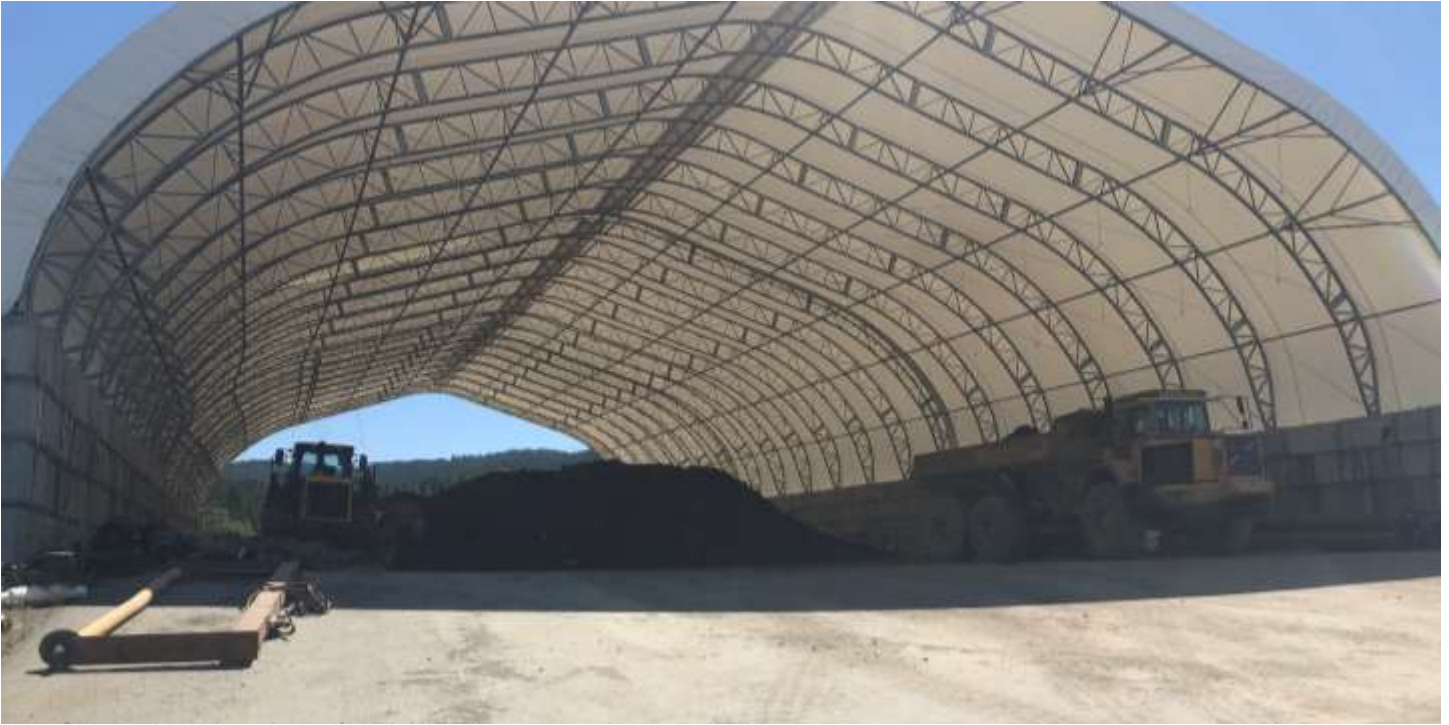
Picture # 1: Alterra loading rock trucks with waste soils from the soil management area (SMA) to relocate to crest of permanent encapsulation area (PEA).
