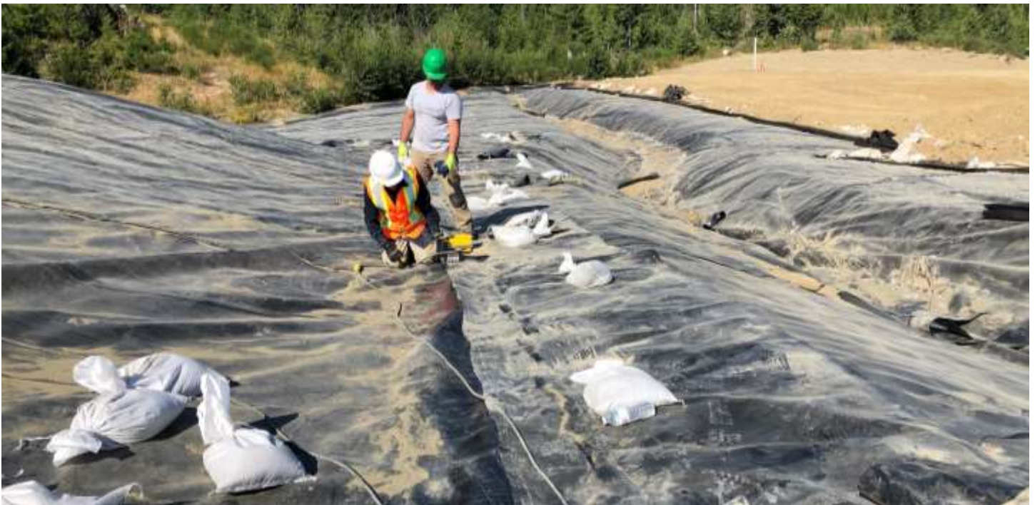
Picture # 8: WTL wedge welding patch on north side of PEA crest.
