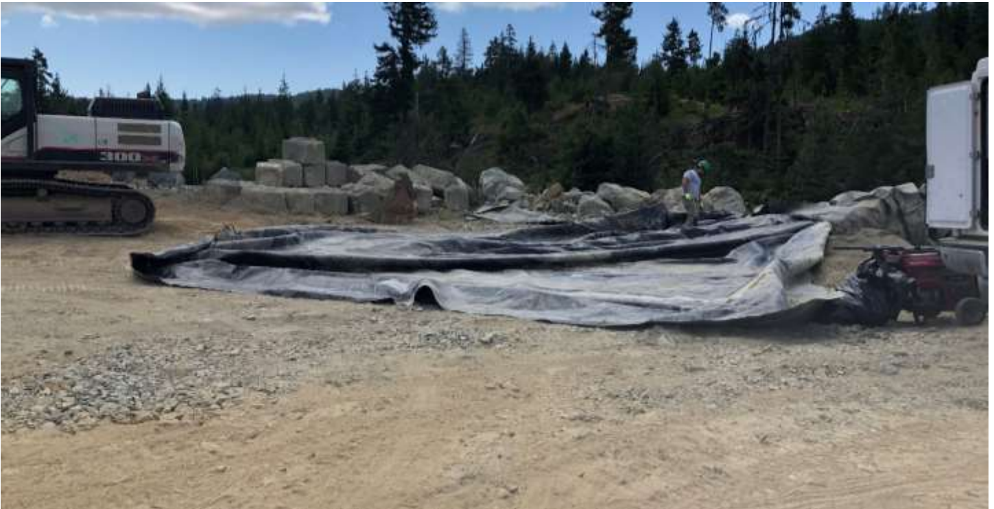
Picture # 1: 40 mil. LLDPE geomembrane on site used for patching and repairs of geomembrane on PEA.
