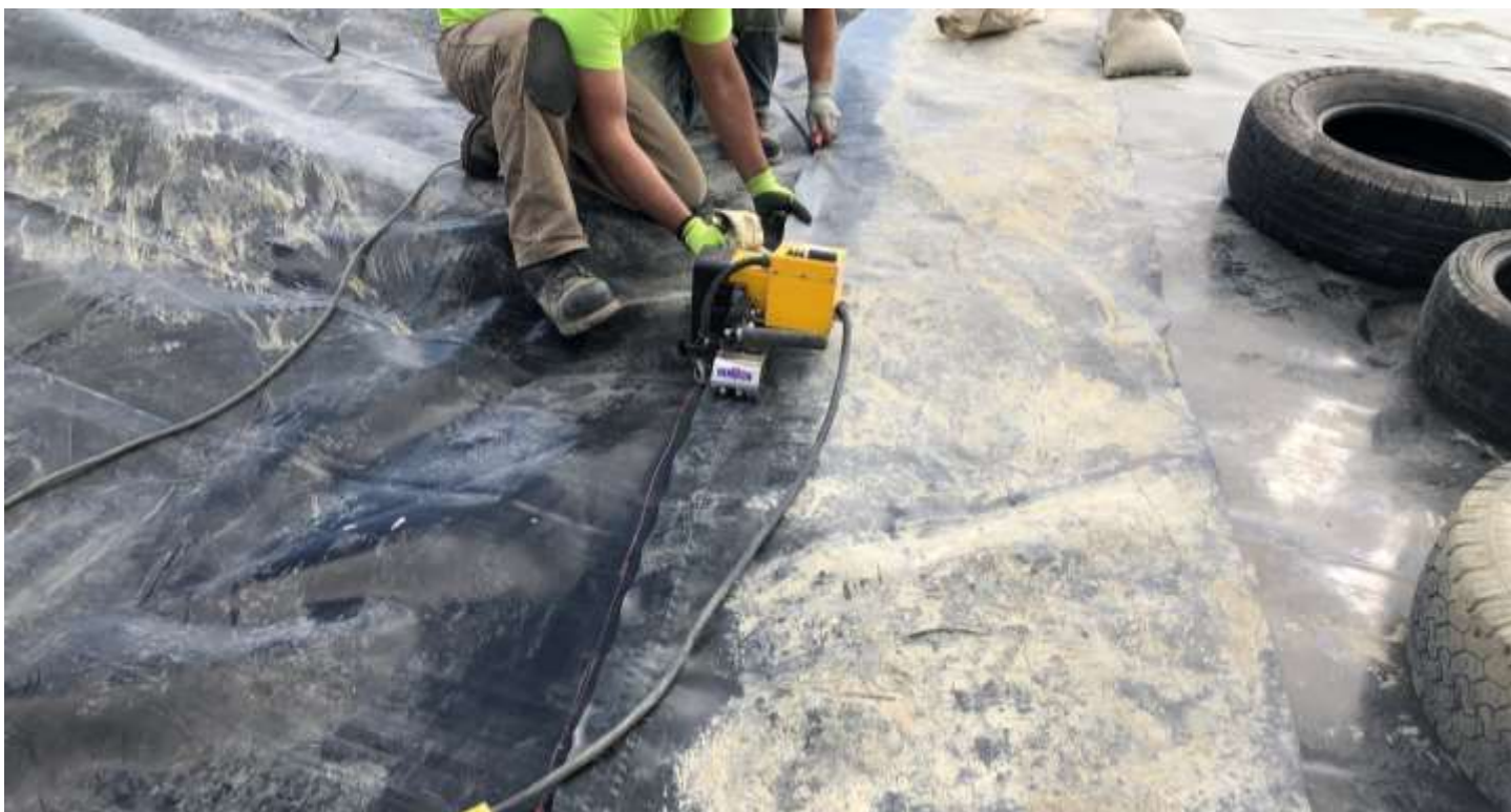
Picture # 4: WTL wedge welding geomembrane patch on crest of PEA.
