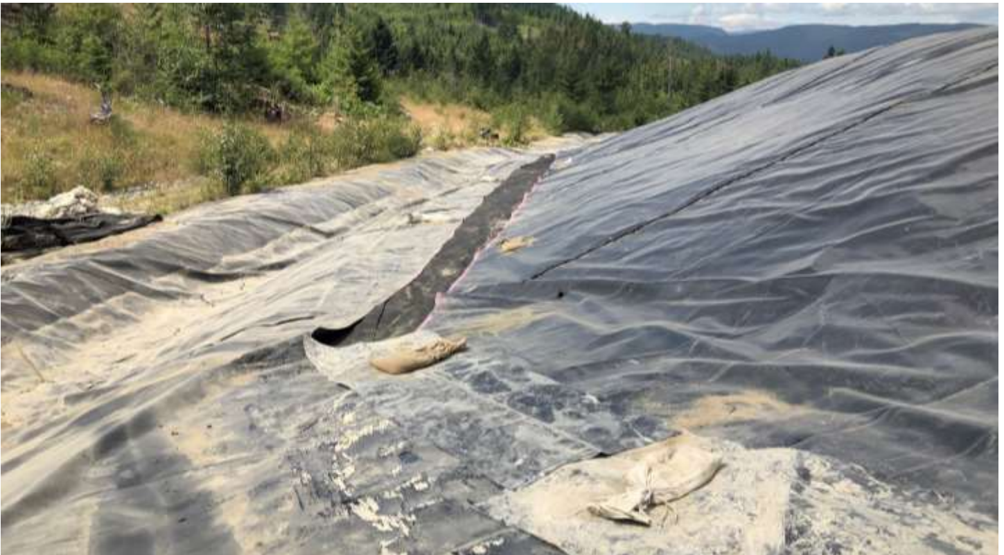
Picture # 4: Strip requiring patching on east side of PEA.
