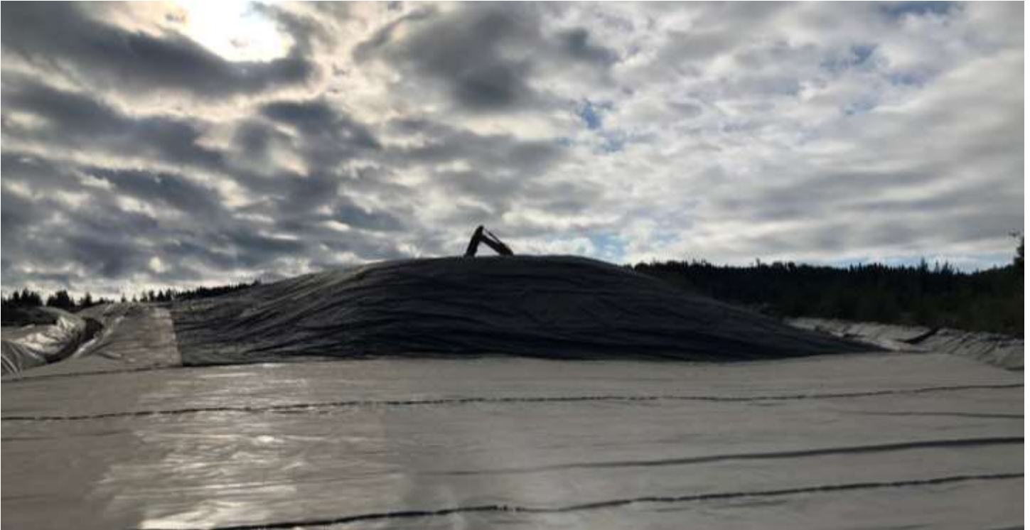
Picture # 5: 12 oz. geotextile deployed on crest of PEA (looking east). The geotextile was tucked under the existing geomembrane by 0.5 m.
