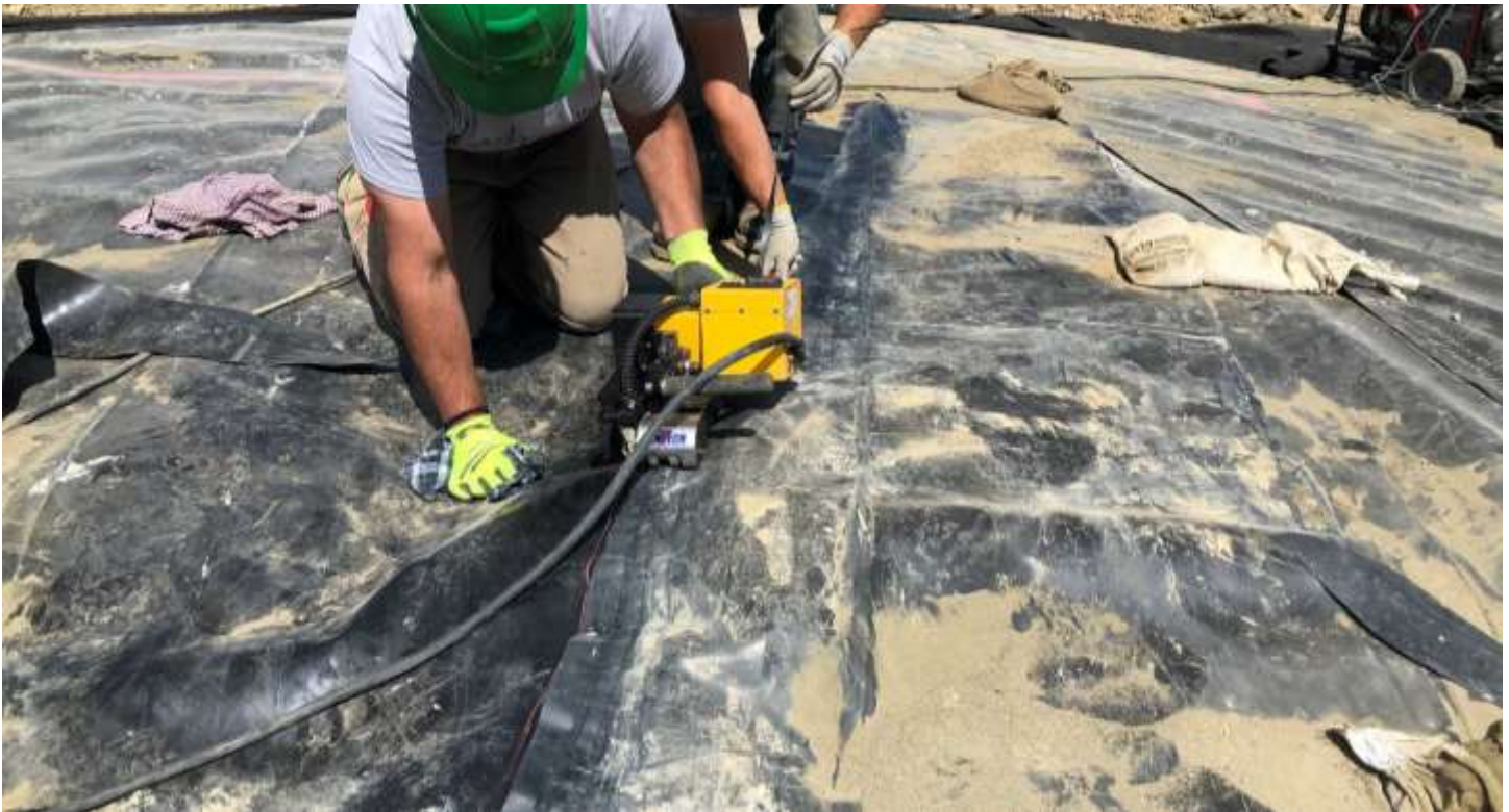
Picture # 8: WTL performing wedge weld on geomembrane patch on PEA.
