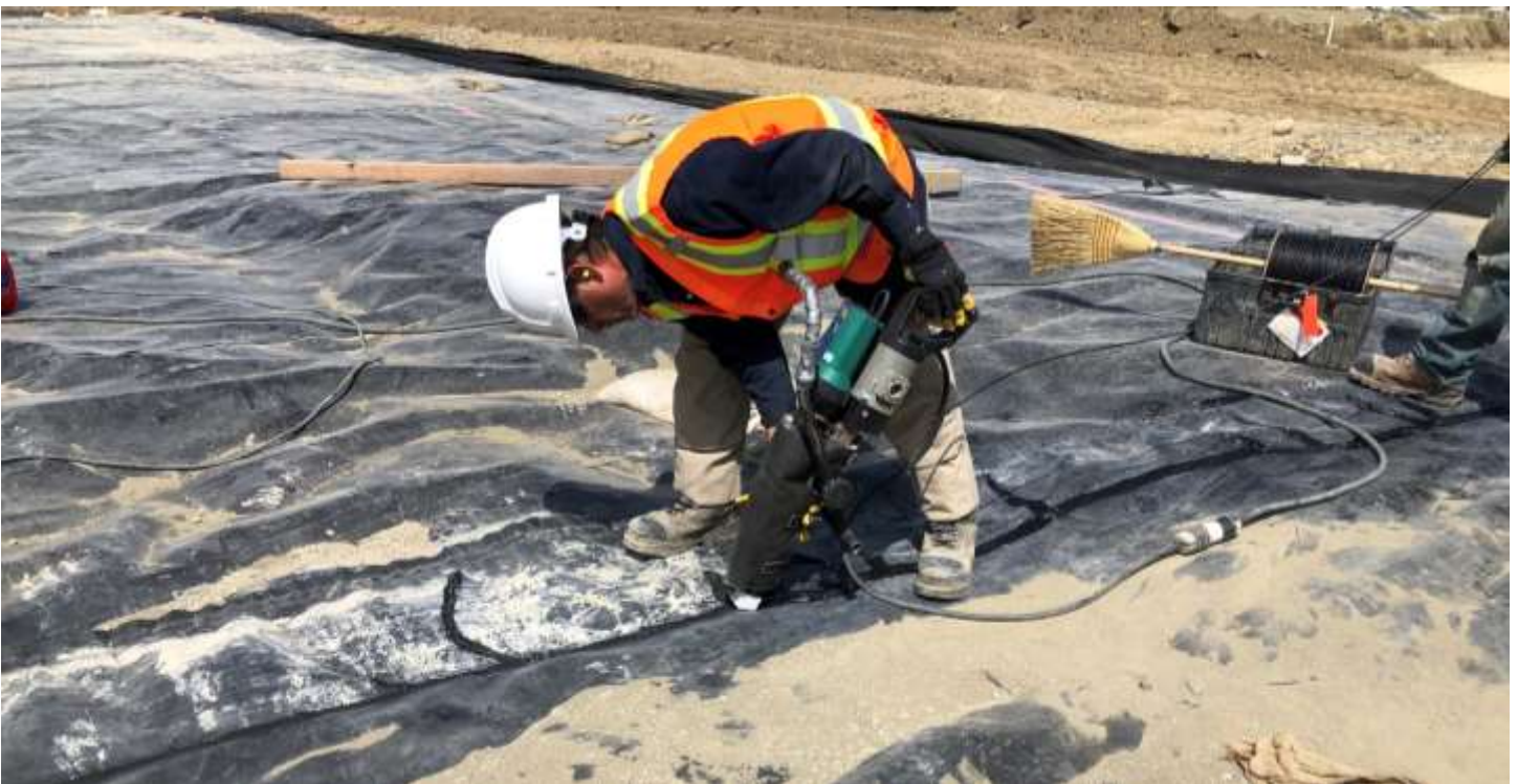
Picture # 12: WTL extrusion welding patch on southeast side of PEA crest.
