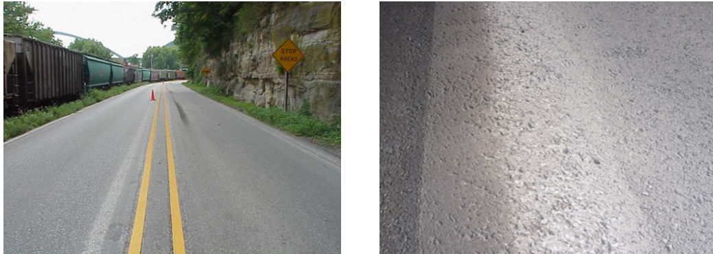
Figure 4.2: Poor Eradication of Temporary Pavement Markings
