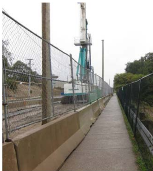
Chain Link Panels on Concrete Roadside Barrier
