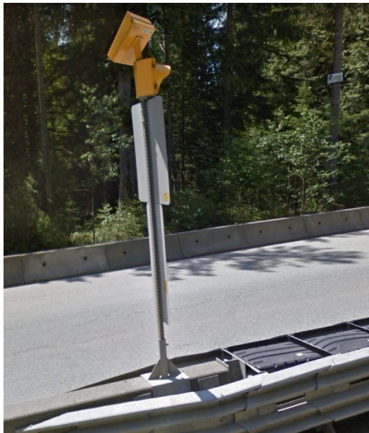
Figure 4.1 B: Barrier Mounted Sign Supports – Saddle Brackets
