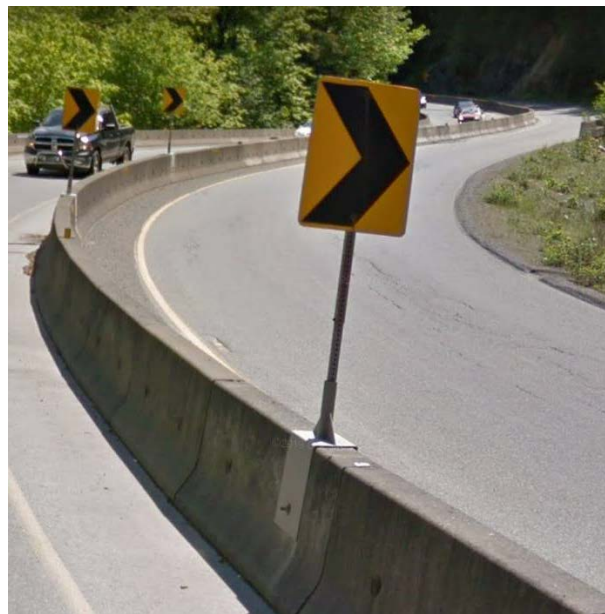
Figure 4.1 B: Barrier Mounted Sign Supports – Saddle Brackets
