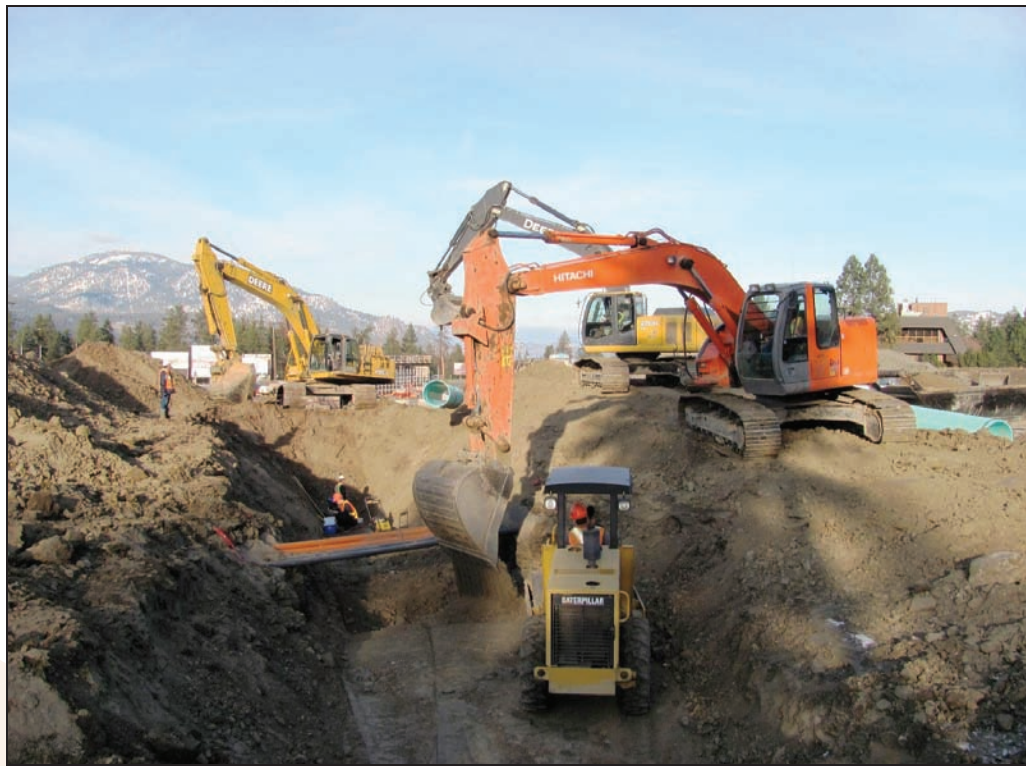
Photo 12.1 – New utility conduit conflict during installation of 750 storm line Dec. 02 2010
