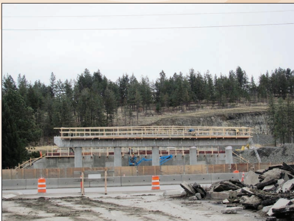
Photo 12.6 – Ledcor back to work, preparing pier for girder installation Jan. 26 2011
