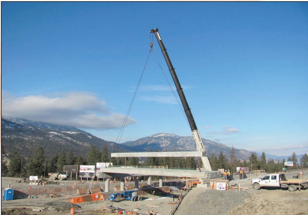
Photo 12.8 – East span girder installation Feb. 01 2011
