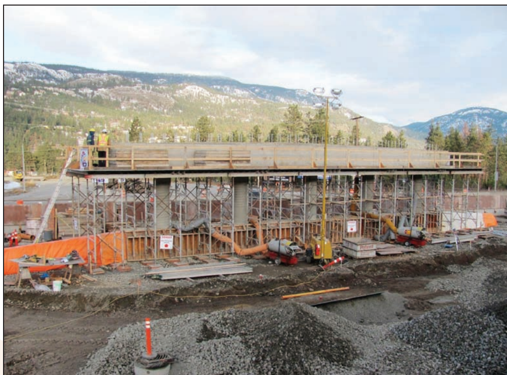
Photo 12.5 – Pier cap formwork removed, dismantling falsework Dec. 15 2010
