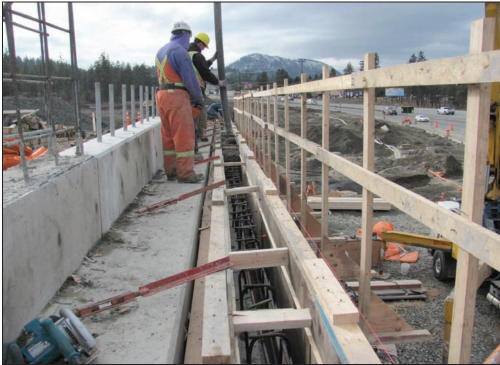
Photo 12.7 – Placing concrete for the coping on MSE Wall “C” Jan. 28 2011
