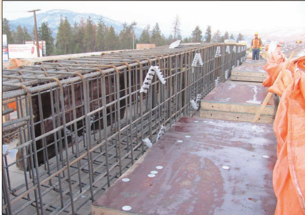
Photo 12.2 – Installation of pier cap reinforcing steel December 06 2010
