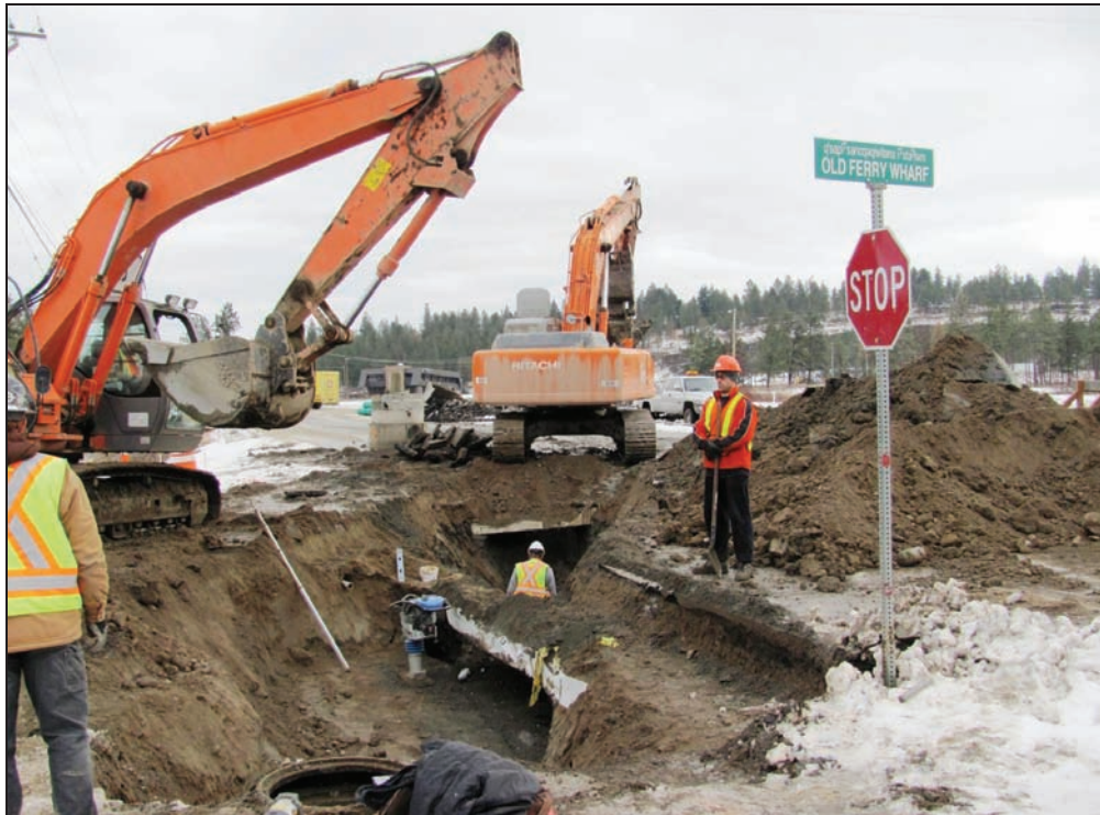
Photo 12.3 – Complex storm line installation due to utility conflicts Dec. 13 2010
