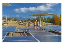
photovoltaic panels mounted on 96 solar trackers that track the sun in two dimensions and produces power for 200 to 300 homes. The power is sold to BC Hydro through a 25 year contract.
