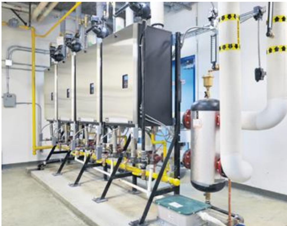
Figure 4: High Efficiency Condensing Boilers (IBC) Installed in Heating Plant Upgrades
