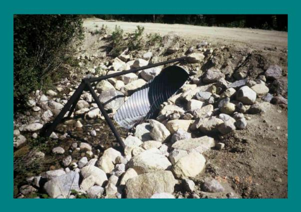
Culvert should be cleared of debris as soon as possible
