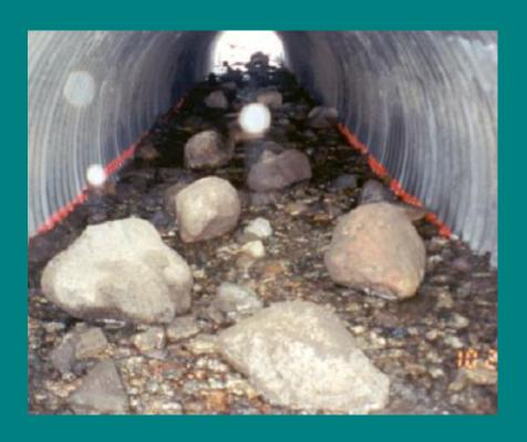
Fines may have to be washed into substrate and/or downstream weir installed
