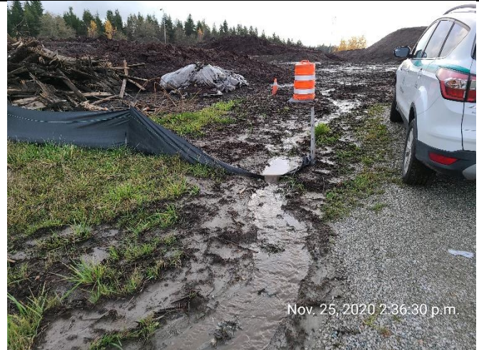
Photo 18. Drainage issued identified near the L2500. Flows overtopping sediment fencing.
