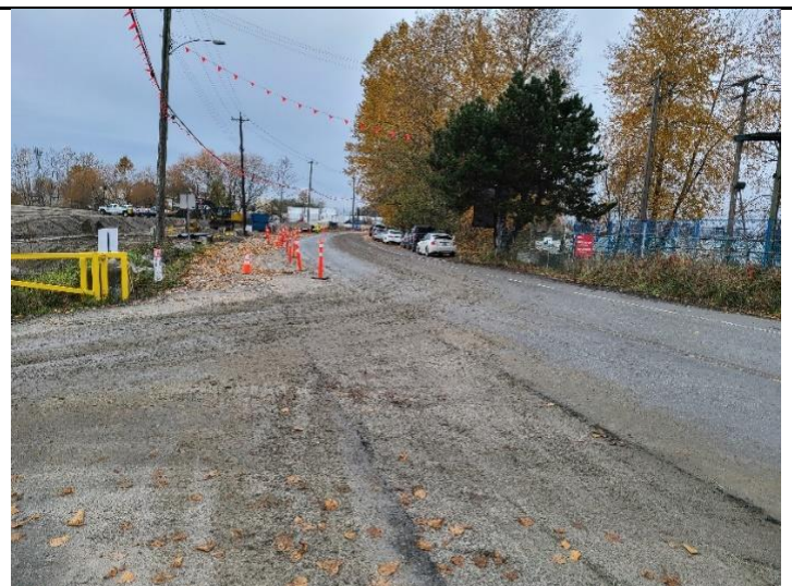
Photo 16. Track out was observed onto River Road West.
