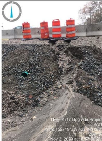
Photo 13. Sand slope washout at Area D east of W01.
