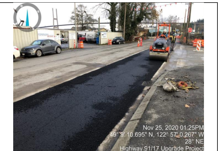
Photo 2. Paving and compacting asphalt on River Road over completed watermain work.
