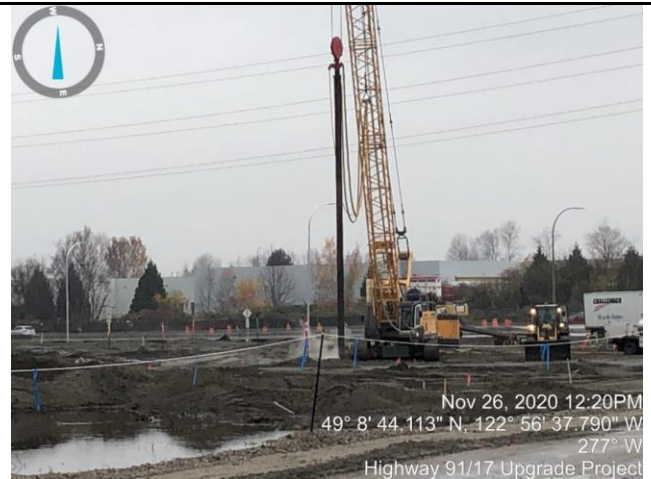
Photo 8. Menard continuing stone column excavation at Area F.
