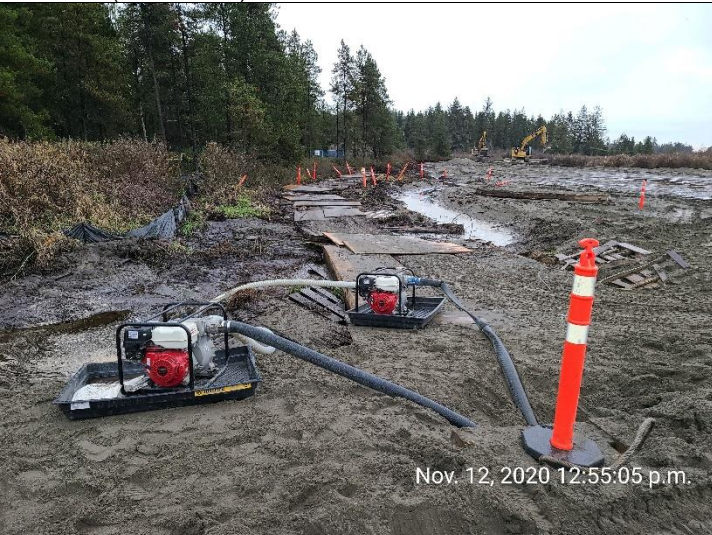
Photo 19. Working surfaces and haul roads were beginning to deteriorate (near L2500).
