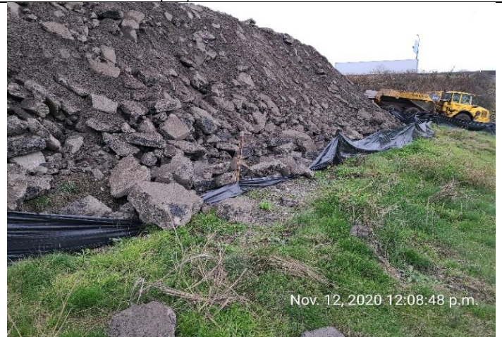
Photo 14. Some sediment fencing had been damaged and needed repairs.
