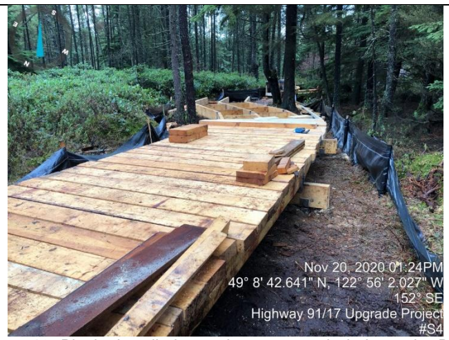
Photo 10. Planks installed on stringers at north tie-in on the DNR Boardwalk.
