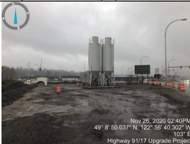
Photo 7. Cematrix mobilizing batch plant for lightweight concrete pour next week (at Area H).
