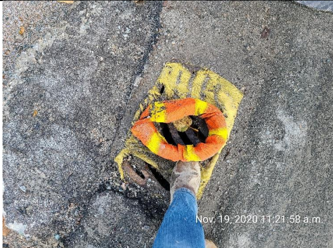
Photo 17. Damaged inlet protection on River Road West (Area C).
