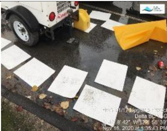
Photo 11. Diesel residue sheen cleanup in the truck parking area.
