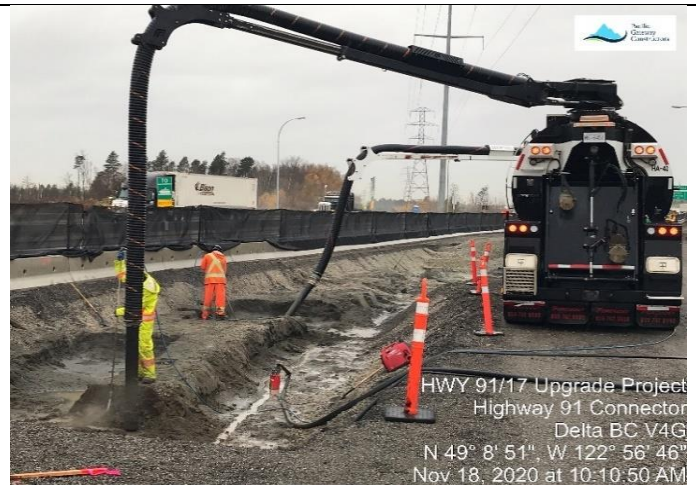
Photo 6. Removal of sand and gravel above the Fortis BC gas line at Area H.
