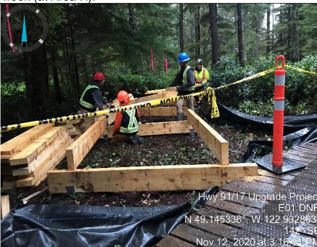
Photo 9. Installing beams and stringers on top of pile caps near the north end of the existing boardwalk.
