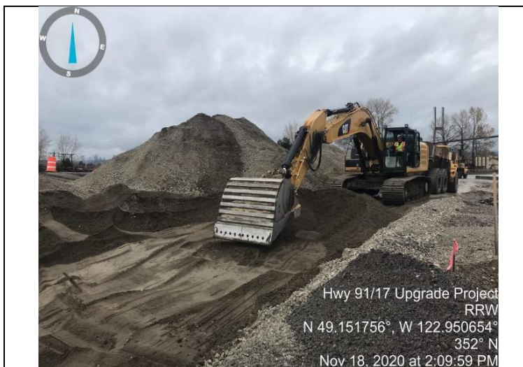
Photo 1. Sand excavation of Hwy 17 off-ramp at Area C. Material to be placed at preload below for L225.
