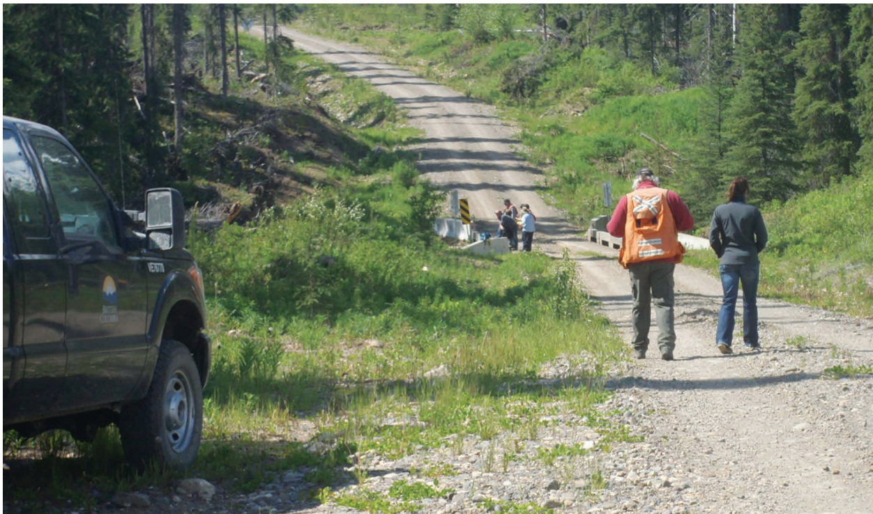
Very low sediment generation potential road surface. Photo Credit: Brian Carson
