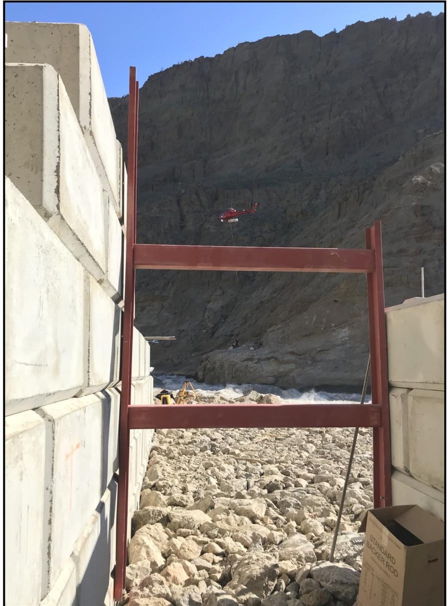
**PICTURED:** Construction continues on the creation of a concrete block fish ladder to guide fish into the pneumatic fish pump system.
