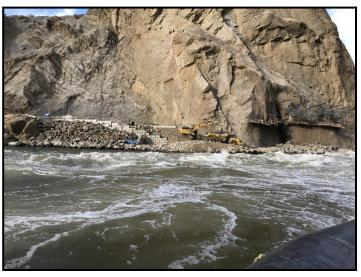
**TOP:** Larger boulders were blasted and broken up into manageable rip rap material for placement.
