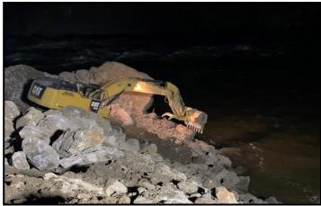
**LEFT:** Two excavators drilling and breaking up large boulders into rip rap material for use along the access route. **RIGHT:** An excavator removing existing rip rap material from West Beach during a night shift operation.
