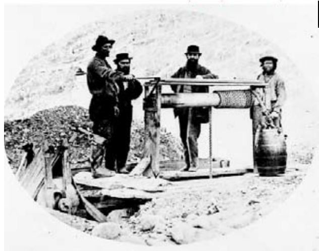
The windlass was used to bring gold-bearing gravel from the bottom of a vertical shaft dug down to bedrock. A-03858
