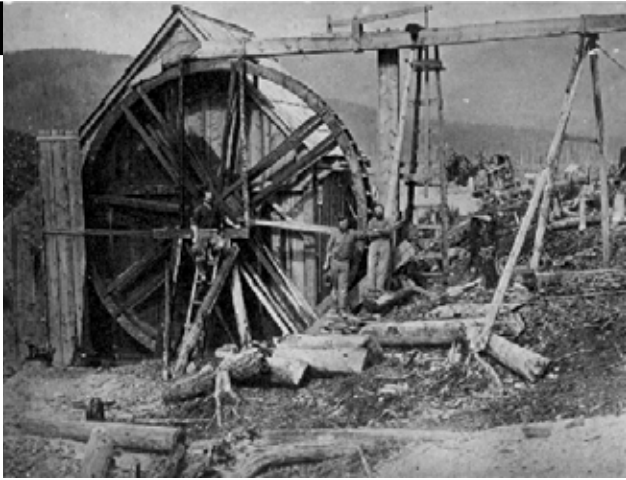
The water wheel was used to bring water or gravel up from shafts dug down to bedrock or to get water to a sluice box to wash the gravel. A-00558
