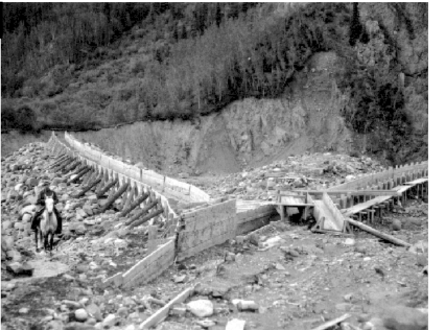
Water was brought down to the creek bottoms by a system of flumes to wash the gravel banks down to get at the gold. E-01107
