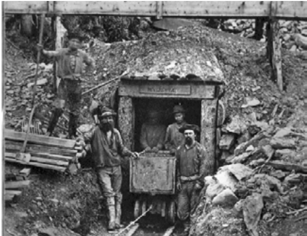
Horizontal tunnels were possible along the sides of creek bottoms to search for the gold in the gravel. A-00937
