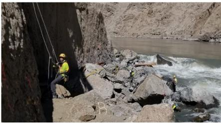
Rock scalers work at the bottom of the west canyon wall and manipulate rock at river level to maximize successful passage of salmon.
