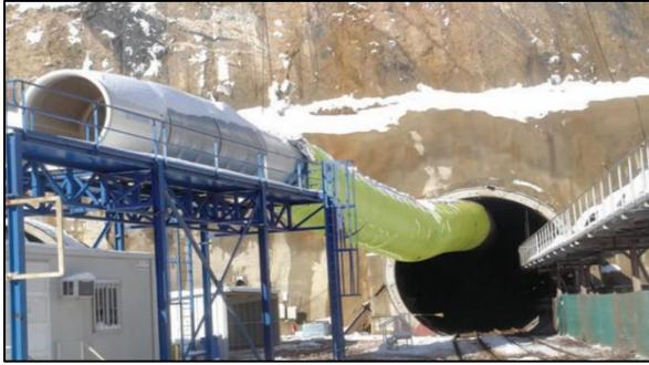
**Positive pressure ventilation** uses a fan to create a high-pressure zone. In underground operations, this is done by placing a fan at the entrance of a tunnel, facing inwards. The high-pressure air in front of the fan will flow to the lower pressure areas further from the fan. The scooping action of the fan blades prevents the air from flowing back through the fan.
