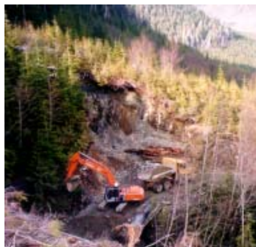
Near Block B102A on P-29 road, a Hitachi EX300 excavator works removing an old bridge as part of road deactivation. The company spent $711,110 on road deactivation in the TFL during the year.
