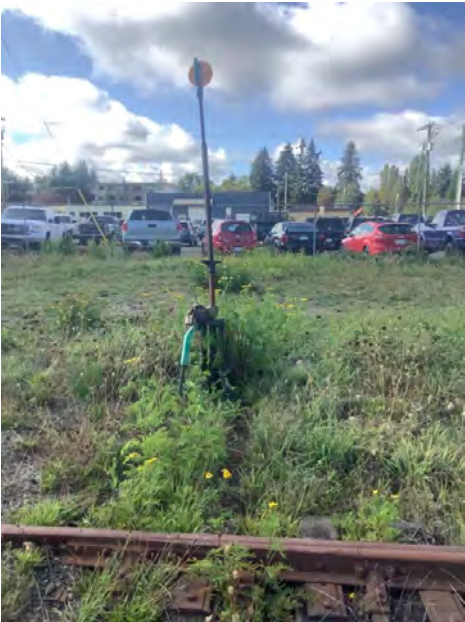
Additional Photo 1 Description Switch stand
