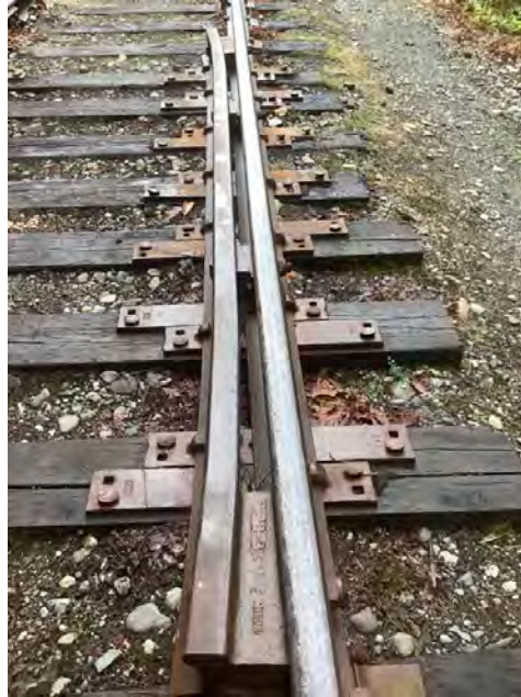
Additional Photo 2 Description Guard Rail
