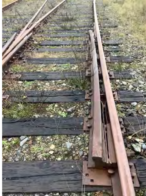
Additional Photo 2 Description Diverging gourd rail
