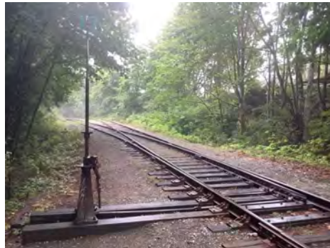
Additional Photo 3 Description Switch Stand
