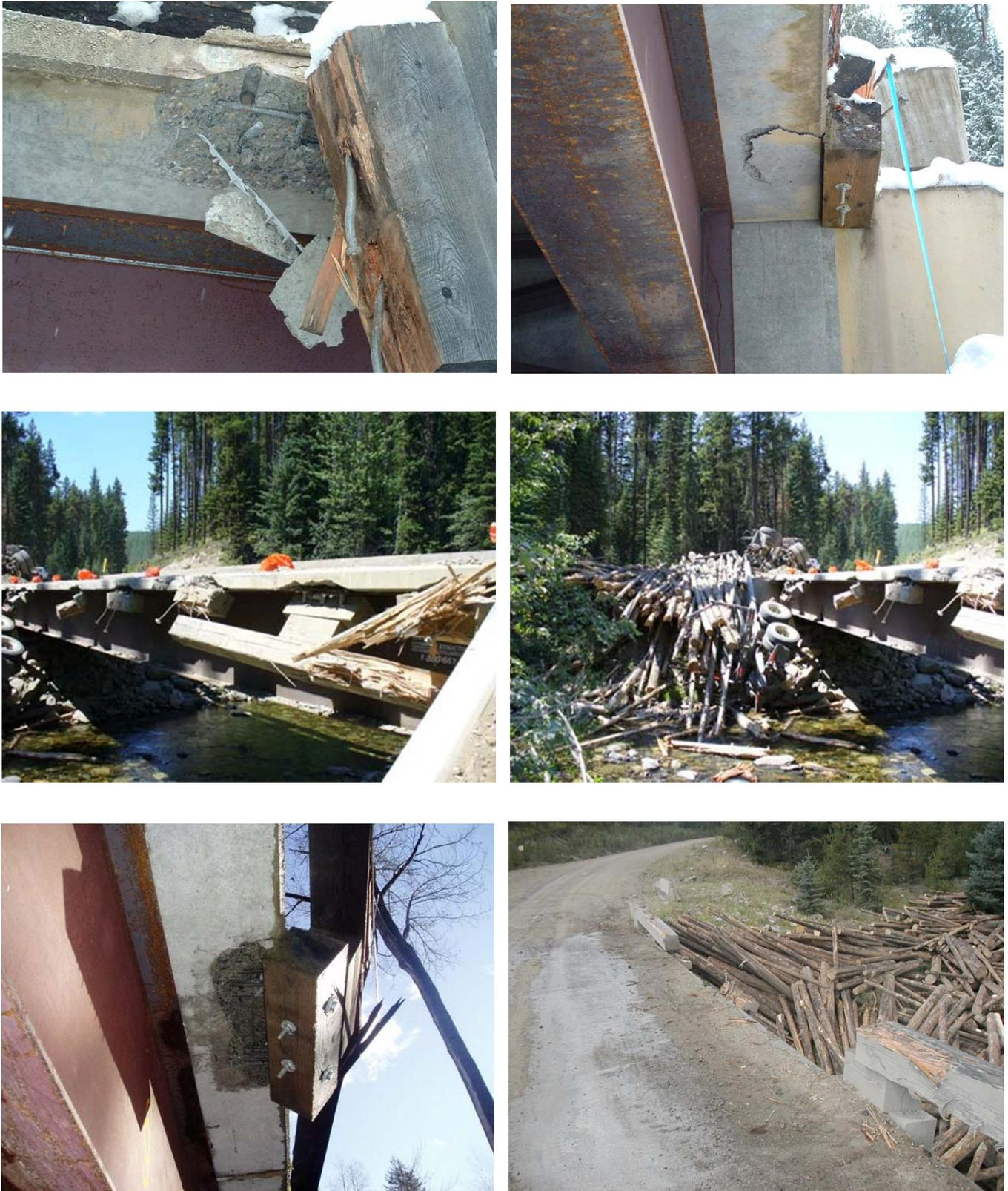
Figure 1: Photos from Actual Field Failures of Various Barrier Types, Group 1
