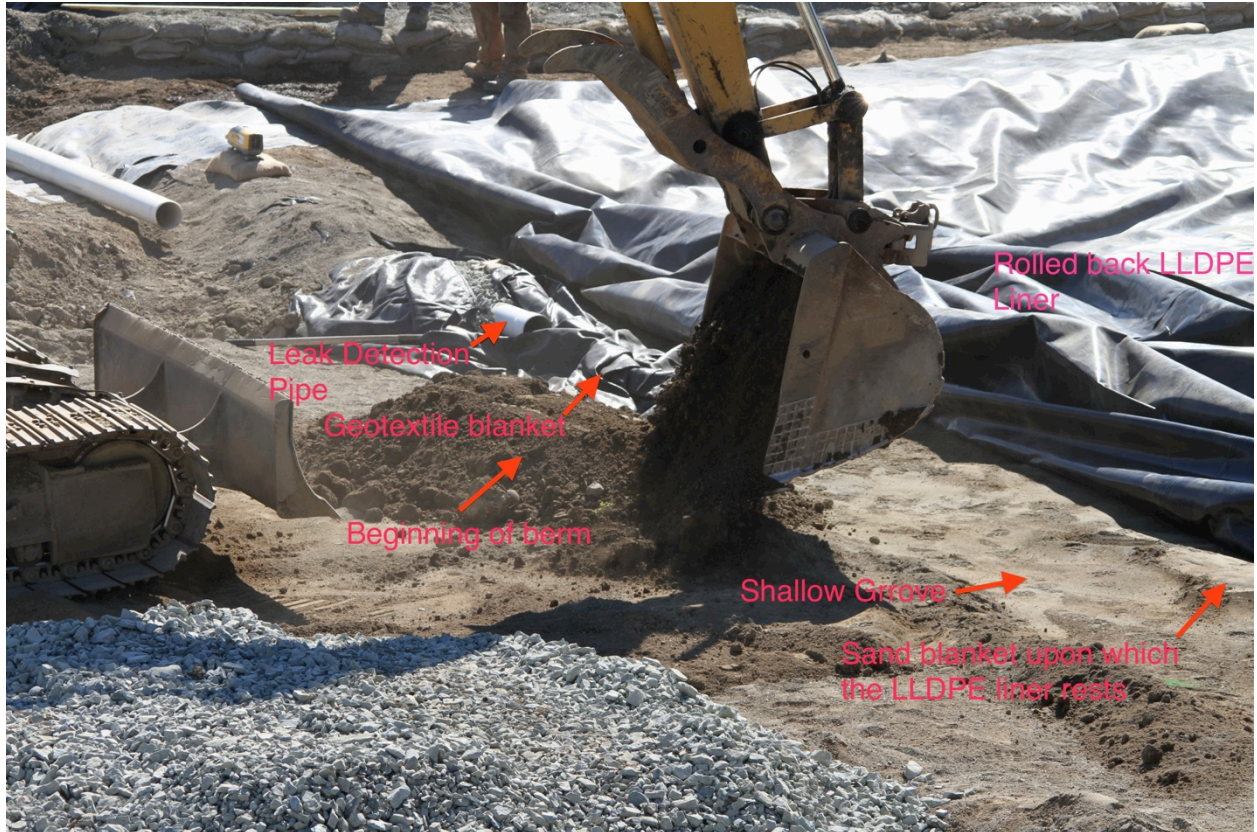
Figure 2. Early stage of [REDACTED]'s leak detection system construction.
