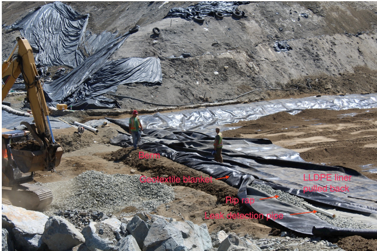
Figure 4. Demonstrates the 'leak detection' system extending further in the westerly direction.
