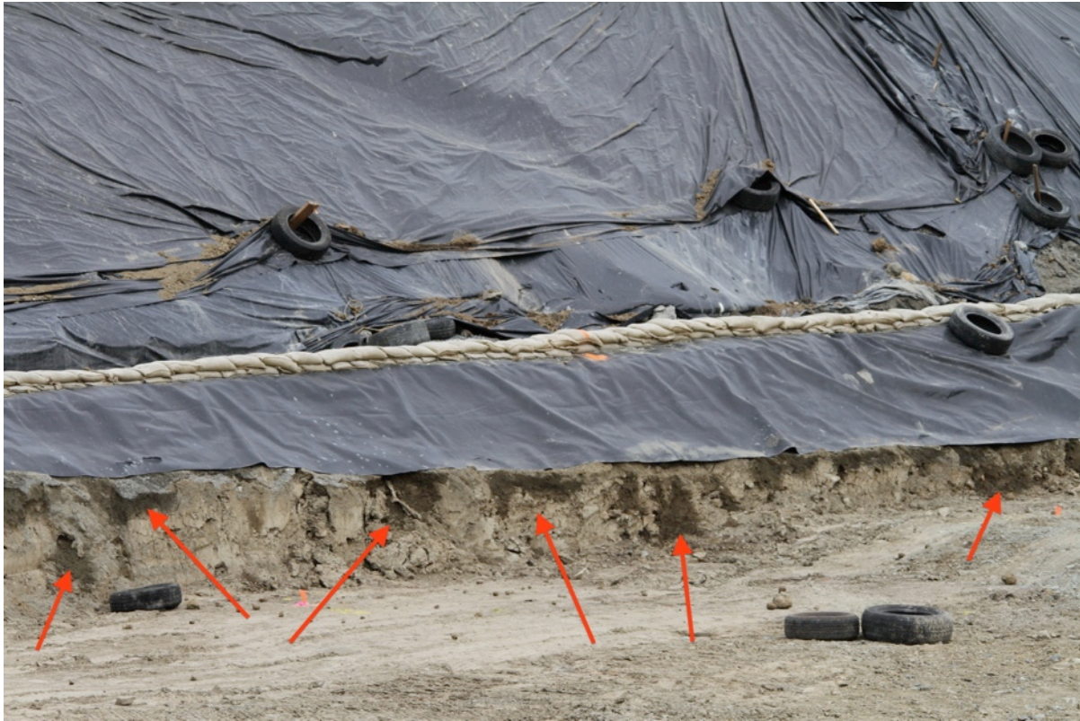
Figure 8. Photo taken in May 2016 of the original Contaminated Soil Containment Area #1 after more than a month without rain. This is a view of the westerly face of the landfill. Clearly seen are wet areas in several locations in the clay berm that lies below the LLDPE liner. Similar wet areas persist to the present day, although now hidden by the newly established unfinished Contaminated Soil Containment Area #2.
