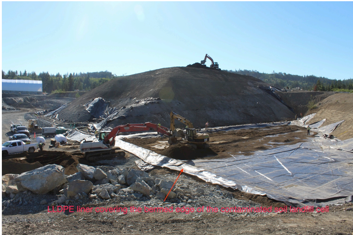
Figure 6. Once the 'leak detection' system is completed work will start on the leachate detection system.
