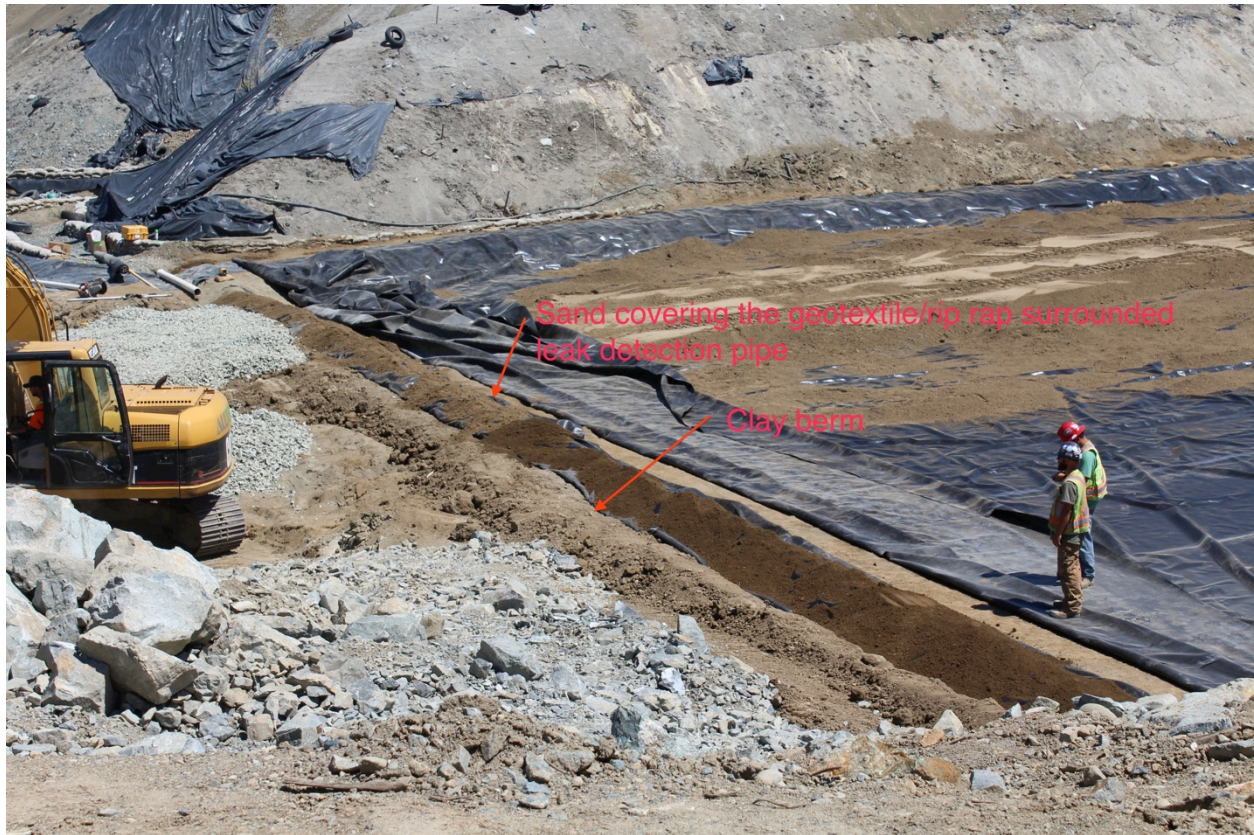
Figure 5. Covering the ‘leak detection’ system with sand.
