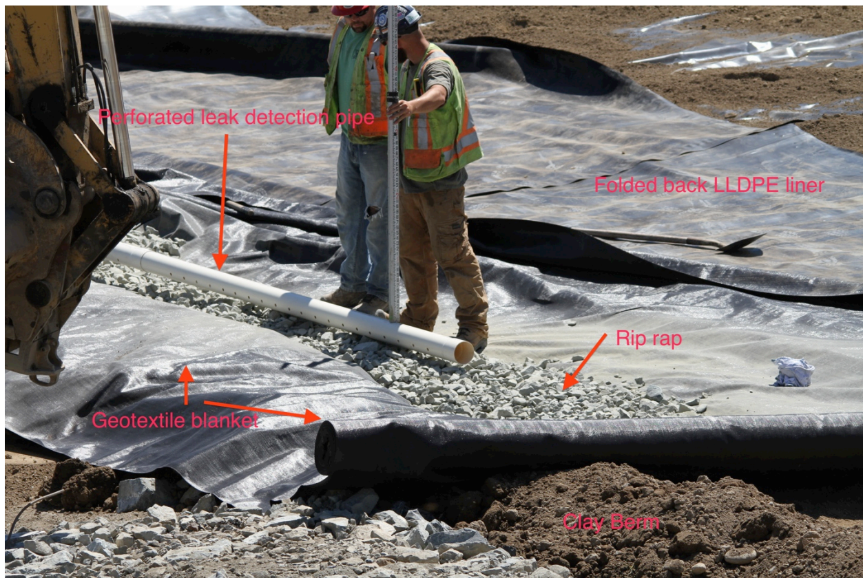
Figure 3 illustrating how rip rap is placed around the leak detection pipe.
