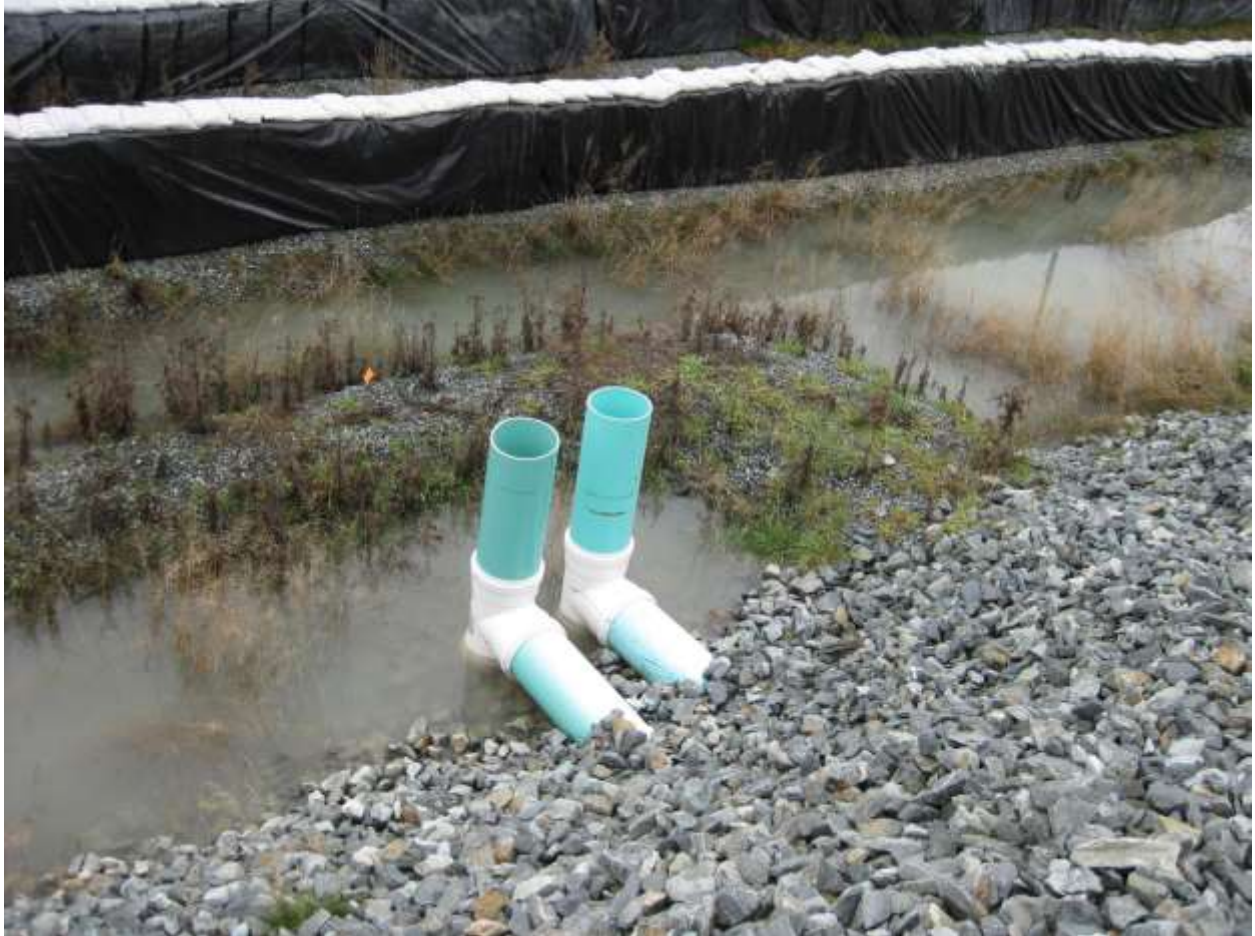
Photo 5: Close up of outlet pipes of sedimentation pond.
