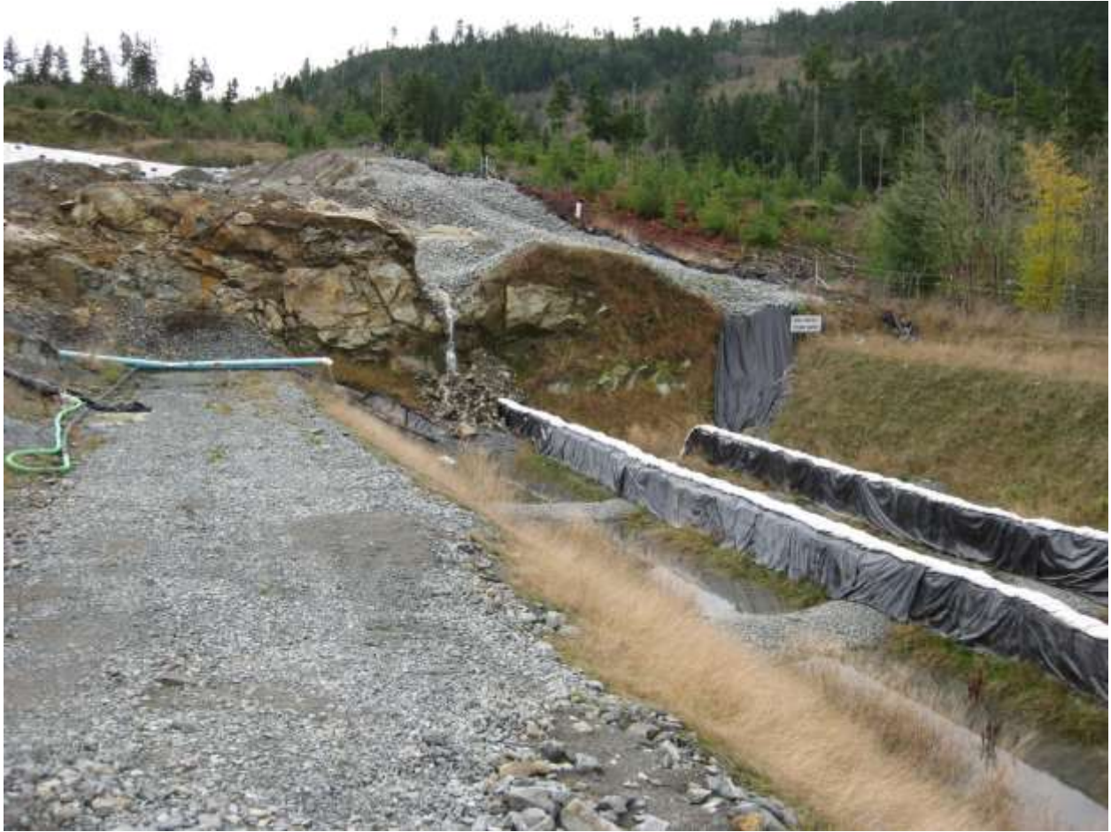
Photo 3: Close up of inlets for sedimentation pond. Looking South
