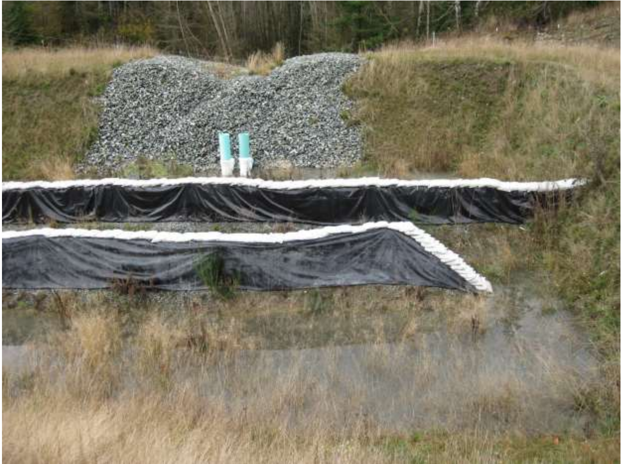
Photo 4: Close up of outlet and overflow of sedimentation pond. Looking West.
