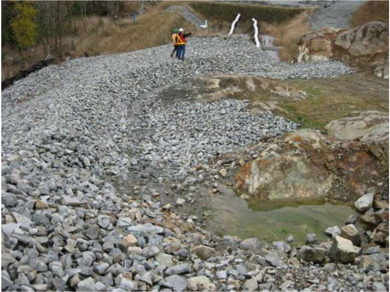
Photo 6: West ditch to sedimentation pond. Looking North.
