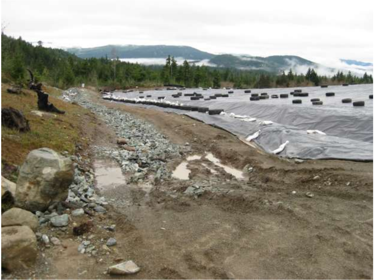
Photo 7: Upstream end of East-West Ditch with encapsulation cell. Looking West.
