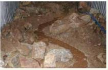
The natural establishment of a non-peak flow channel may occur next to the culvert wall. To promote more area of the channel to be exposed to a natural substrate (i.e., away from the culvert wall), triangular gyrons constructed of aggregate have been used to force the low-flow channel to meander through the culvert.
