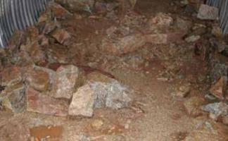
Large boulders help anchor the imported material within the culvert and help prevent it from being easily eroded. This D90-sized material should be placed at various depths within the delivered material as well as along the surface. The surface material will help prevent material from eroding as well as provide velocity shadows for fish passage during high flows.
