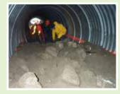
A conveyor system provides a means for infill material to be delivered into the culvert.
