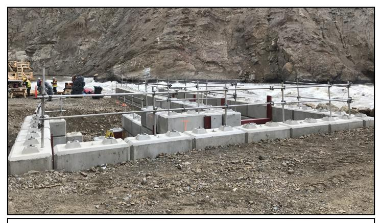
PICTURED: Guardrails being installed around the now-completed concrete fish ladder
