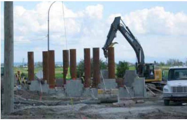
North abutment MSE wall construction
