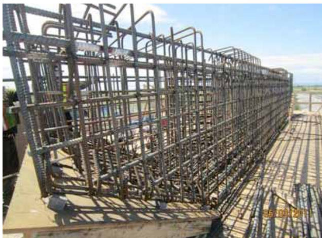
Pier – installation of cap reinforcement
