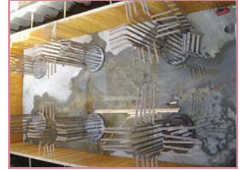
Pier 2 – Forming up the pile cap
