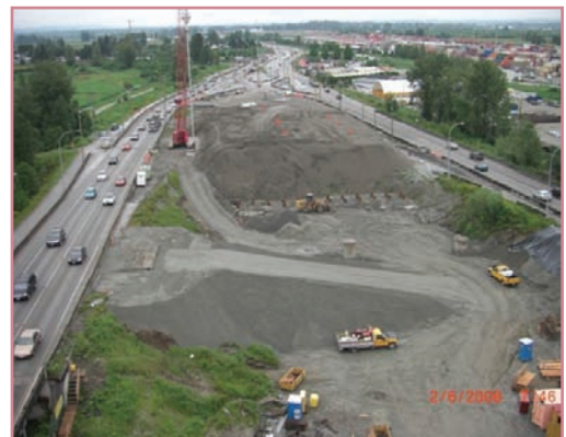
View of preload at east end. Piles for Abutment can be seen at base of preload. Crane at left side of screen is carrying out installation of stone columns to improve seismic stability of soils.
