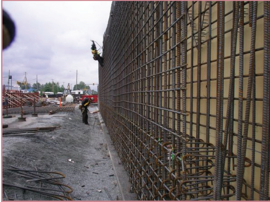
Erection of north abutment for interchange structure
