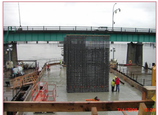
Start of pylon erection at W1
