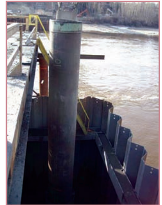
Pier 3 – Rock sockets to downstream piles
