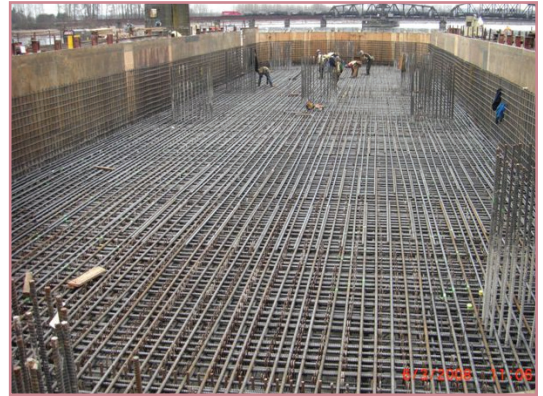
W1 pile cap prior to placement of concrete.
