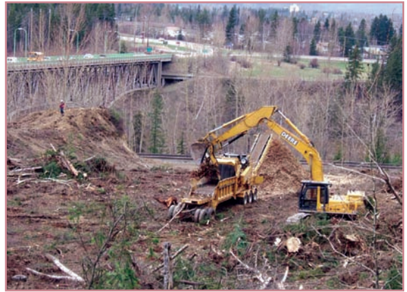
South approach – clearing grubbing, tree mulching
