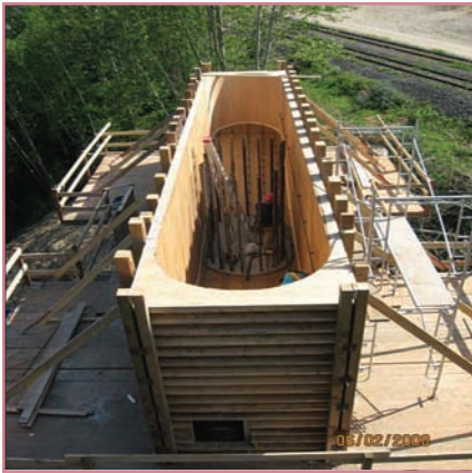
Form work for Pier 1 cap
