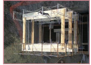
Pier 1 – Support and access tower viewed from the existing bridge
