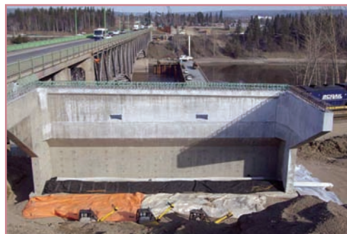
Bridge endfill activities suspended at the Southern Abutment due to freezing temperatures
