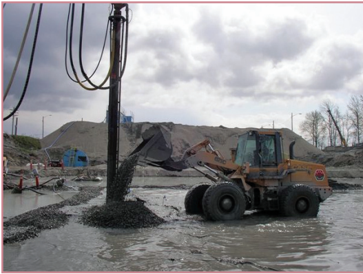
Installation of stone columns on west side.
