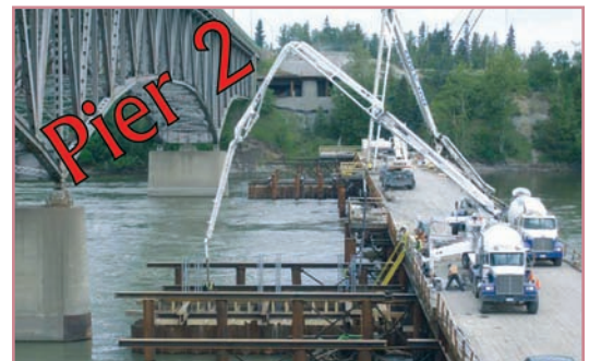
Pier 2 – Concrete placement with two pumper trucks on temporary structure
