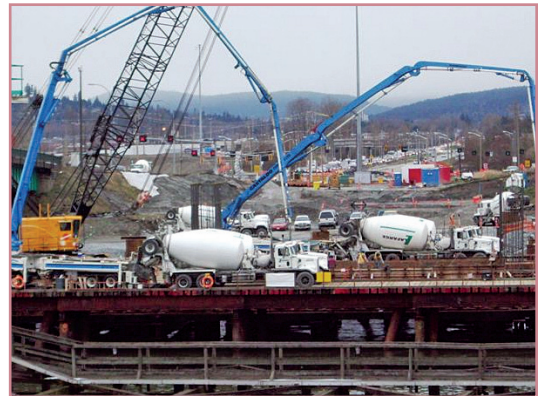
Pouring of concrete at W1 pile cap
