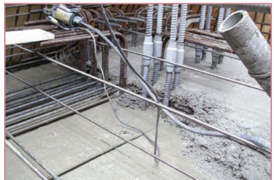
Pier 2 – placing concrete on top of construction joint
