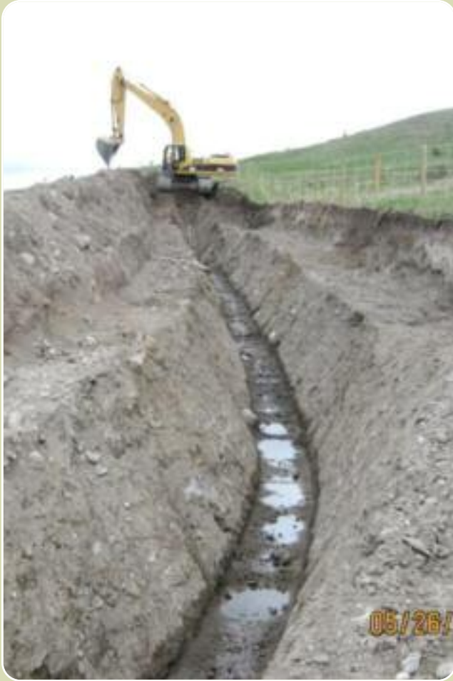
Cutting ditch for subdrain along top of cut at Sta. 132 area.
