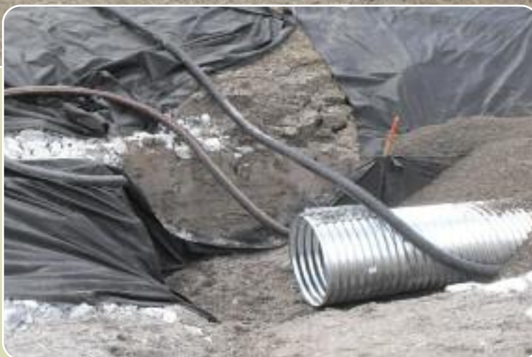
Installation of culvert and sub-drain pipes at slope failure west of McBride Timber Road
