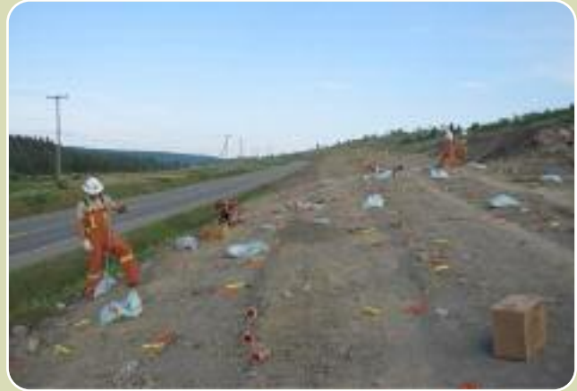
Loading for blasting Type A material Sta. 132 to 133+50 area
