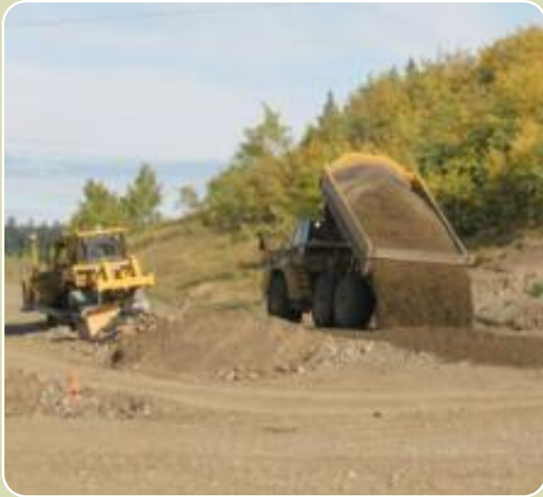
SGSB placement on re-constructed existing road between the L200 and L250 Lines
