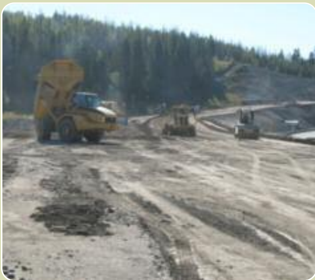
Subgrade Construction
