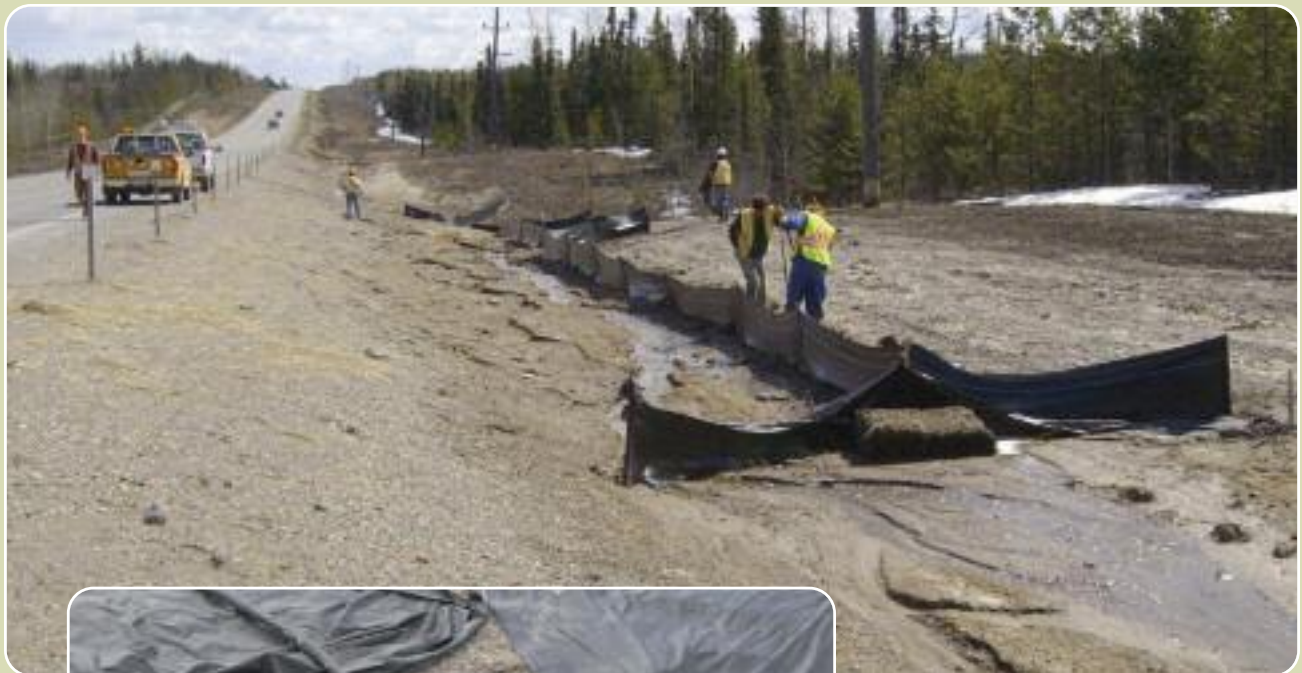
Reinstalling silt fencing
