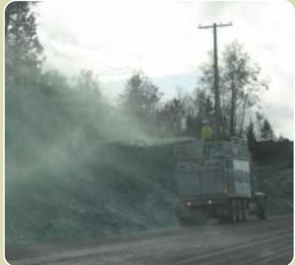
Sta. 121 – Hydro seeding cut slopes
