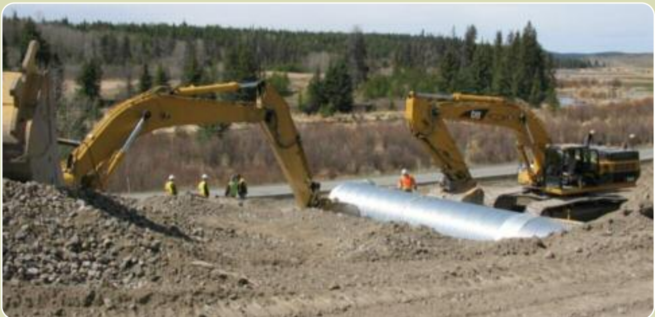
Installation of 2000mm Wildlife Culvert
