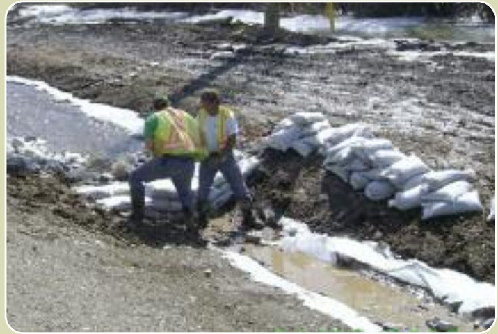
Sandbag ditch blocks diverting water in culvert
