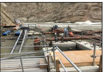
**TOP:** Construction of a new elevated pad for Whooshh<sup>™</sup> control system container.
