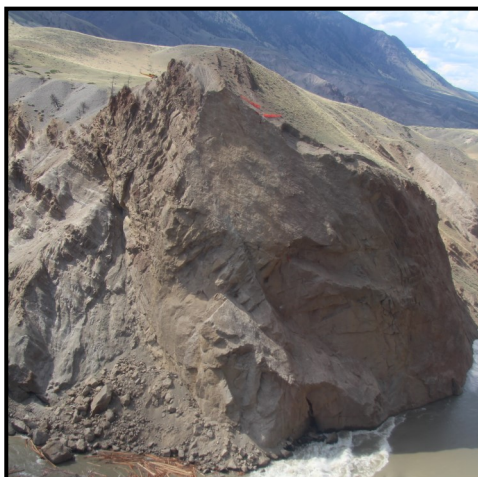
Figure 5. The landslide face after the controlled blasting operation.
