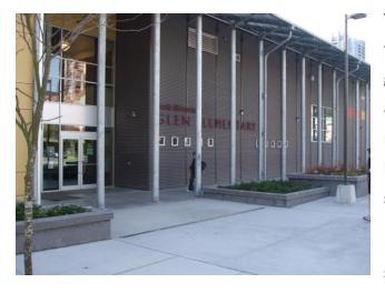
The New Glen Elementary School was completed with the consideration of the LEED Silver standards as a guideline. The new school introduces a passive heating and ventilation system with radiant floor heating for maximum efficiency. Large volume of glazing for day lighting opportunities and enhanced building envelope strategies were considered throughout the design.
