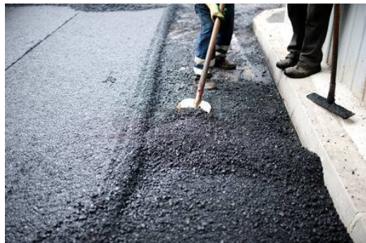
Figure 2 - Asphalt being used during road construction (Hoda 2017)
