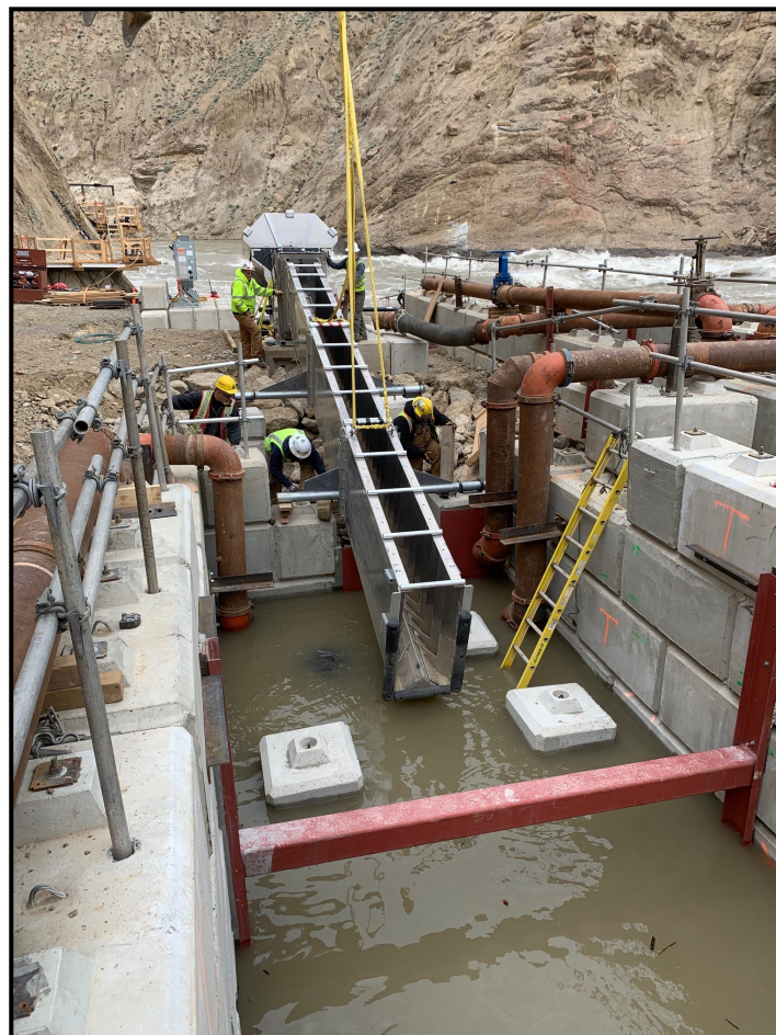
PICTURED: Installing a Whooshh Passage Portal™ component inside the concrete fish ladder
