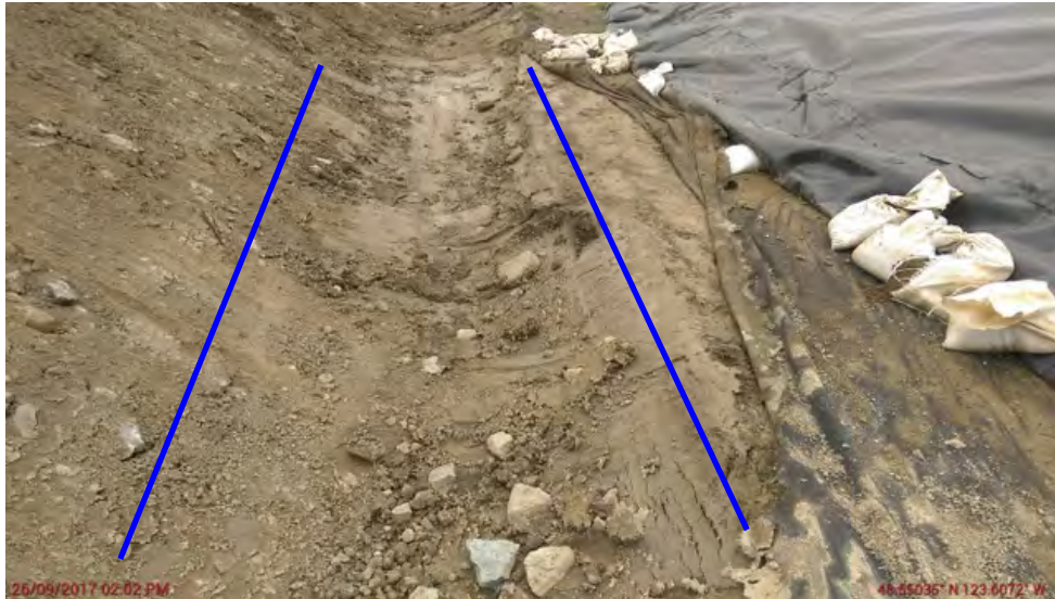
Photo 1.5 – Clay observed under south perimeter ditch. Blue lines represent approx. edges of observed clay.
