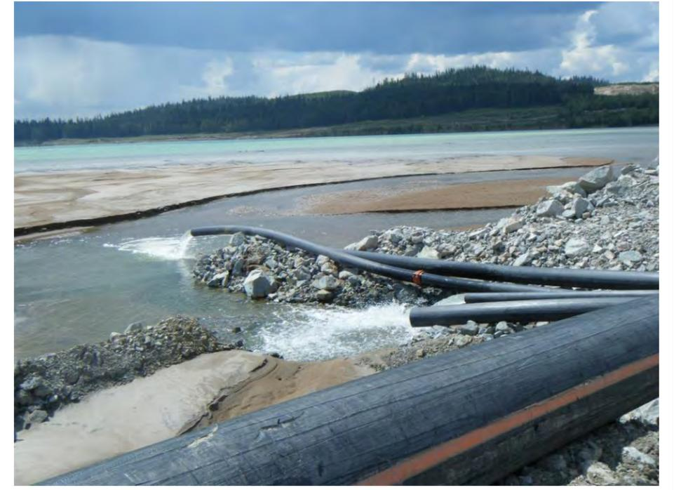
Photo 15: Perimeter seepage pond discharge into the TSF.
