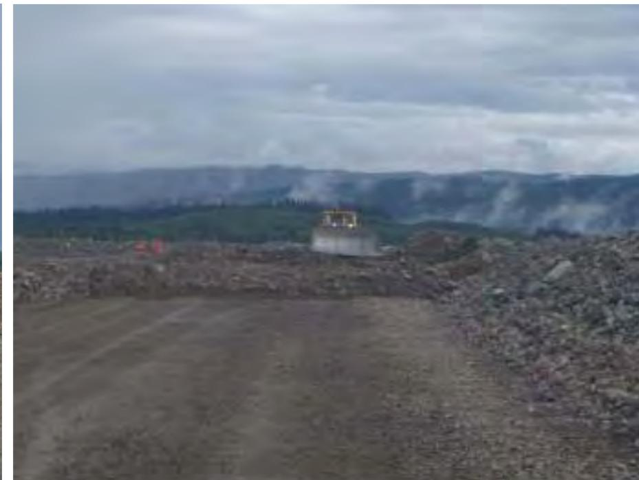
Photo 33: Zone C placement along the south embankment.
