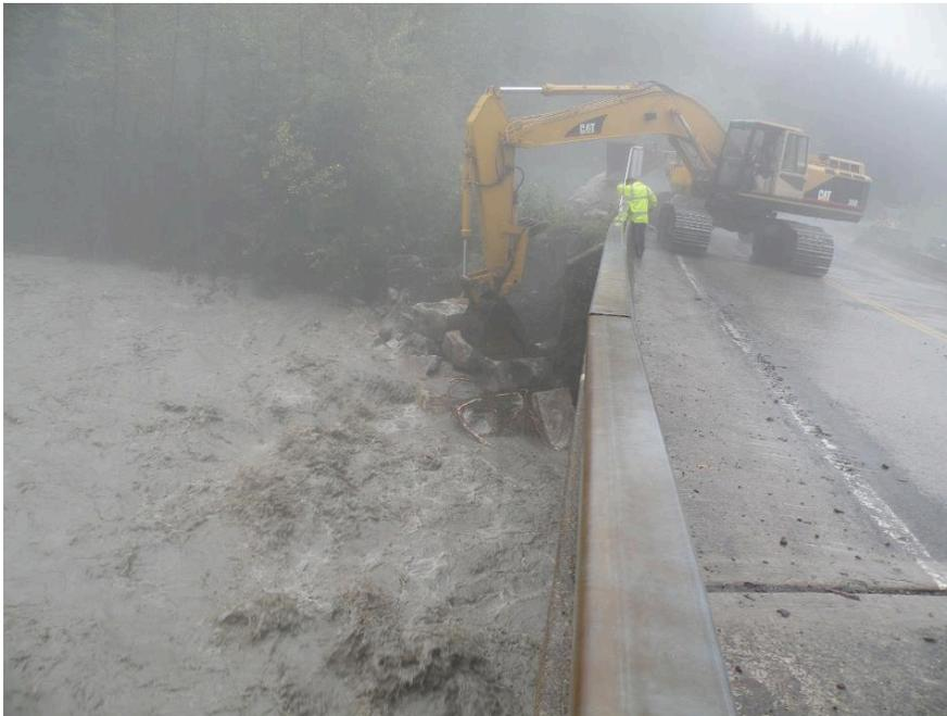
**Photo 4:** Emergency protection being placed at the west abutment of Bitter Creek Bridge shortly before the bridge was washed out (September, 2011).
