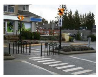
Many countermeasures help protect pedestrians. For example, Danish Offsets at the middle of a multilane crossing provide refuge for pedestrians and ensure they are facing the traffic before crossing the second half of the roadway.
