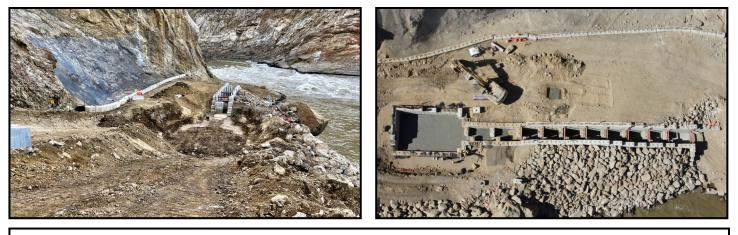
**PICTURED:** Crews excavated the area to the west of the concrete fish ladder to extend it for "trap and transport" operations this year.
