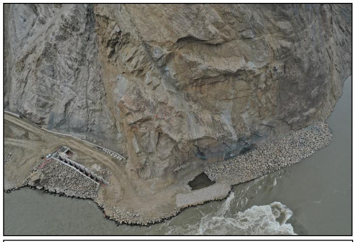
PICTURED: Aerial view of the concrete fish ladder (left) and the "nature-like" fishway (right) on West Beach.
