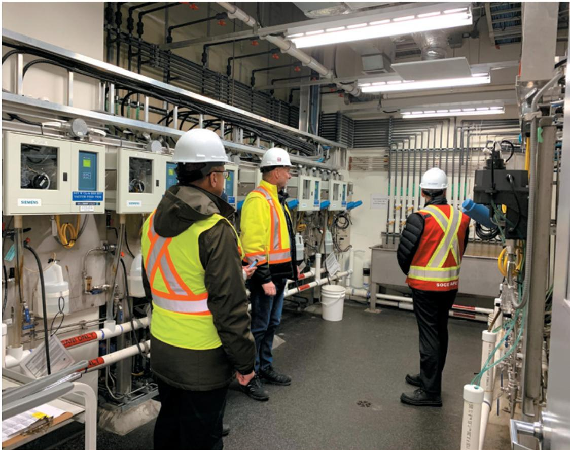
A certified EOC Operator providing a tour of the analyzer/sampling room of the Seymour-Capilano Water Filtration Plant in North Vancouver. Water from different stages of the water treatment process are plumbed to this room for easy dedicated sample collection and to online analyzers for chlorine residual, pH, conductivity, and UV transmittance.
