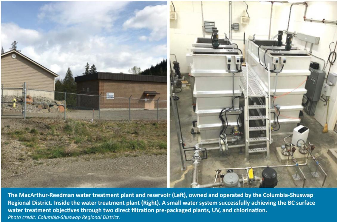
The MacArthur-Reedman water treatment plant and reservoir (Left), owned and operated by the Columbia-Shuswap Regional District. Inside the water treatment plant (Right). A small water system successfully achieving the BC surface water treatment objectives through two direct filtration pre-packaged plants, UV, and chlorination.
