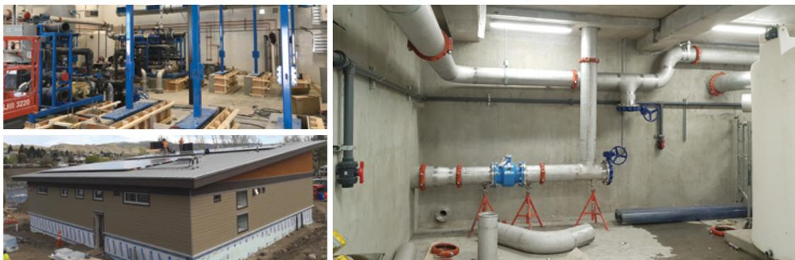
The Village of Ashcroft is building a new water treatment plant (bottom left and right) scheduled to be completed in late summer 2019. The new facility will be equipped with membrane filtration (top left) and a new chlorination system providing primarily disinfection. With the upgrades, the Village will provide potable water that achieves the BC surface water treatment objectives.
