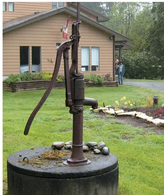
A private water system consisting of a dug well with a hand-pump serving a single-family residence in BC.
