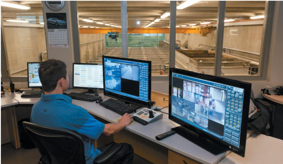
View from the Kamloops Centre for Water Quality Operators Control Room where they have the Supervisory Control and Data Acquisition (SCADA) system and security monitors. Operators can conduct all process operations of the facility from this room.
