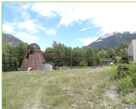
Figure 22 - Decommissioned Wood Residue Burner (ENV inspection files)
