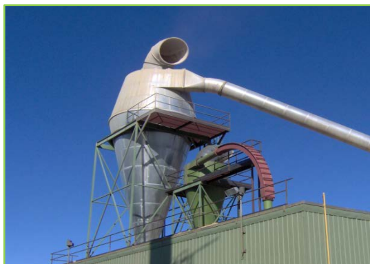
Figure 12 - Cyclone (ENV inspection files)
