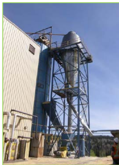
Figure 8 - Planermill Shavings Cyclone (ENV inspection files)
