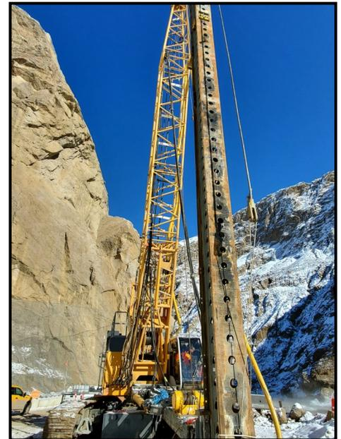
**ABOVE:** The pile installation rig being set-up on the West Beach will be used to drive piles necessary to support the fishway.
